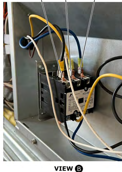
Figure 30 – Supply Connection of the HVAC Heater
