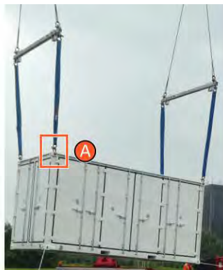
Figure 11 – Crane Lift Assembly (Typical)
