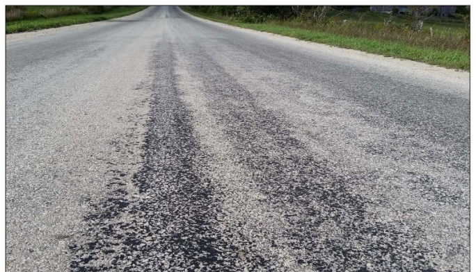
Flushing of pavement
