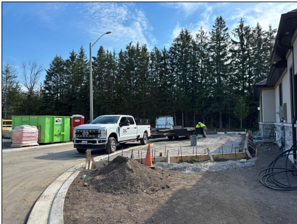
Figure 12: View of the northeastern terminus of the private street on 99 Cloverleaf Drive (future connection to the subject property)
