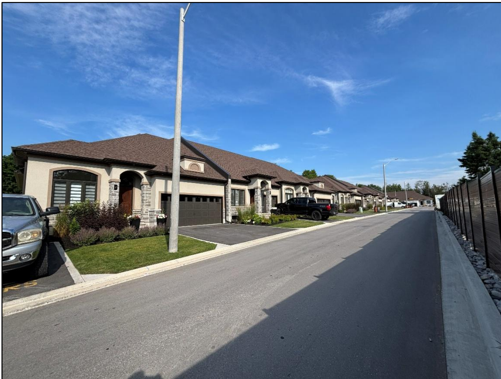
Figure 10: View of 99 Cloverleaf Drive
