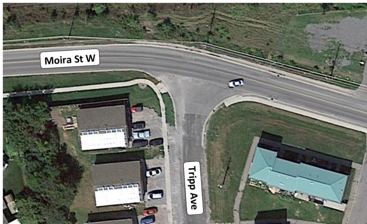
Figure 2-7: Moira St W / Tripp Ave Intersection (Google, Maxar Tech 2015)
