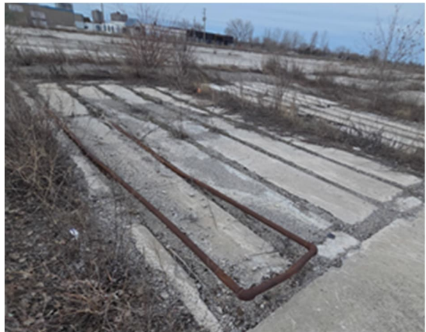
PHOTO 20: View of the pipes imbedded in the concrete footprint of the building located in the central portion of the Phase One Property, facing south.
