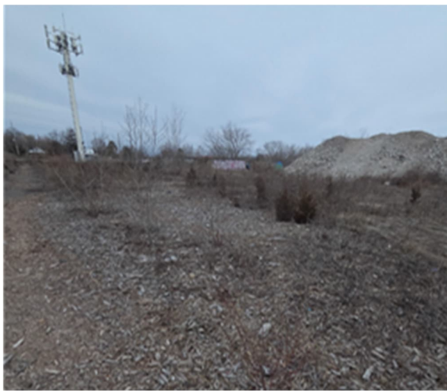
PHOTO 27: Additional view of the 5G tower a large debris pile was located northeast of the tower, facing northwest.
