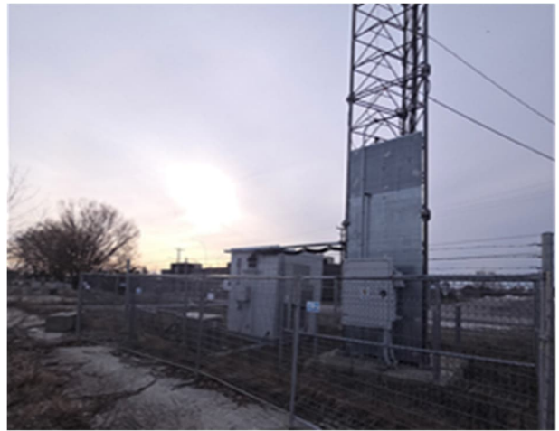
Photo 6: View of communications tower located near the central south limit of the Phase One Property, facing southeast.
