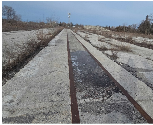
Photo 2: View of formal travel lift lines, with 5G tower near the central portion of the Phase One Property, facing west.
