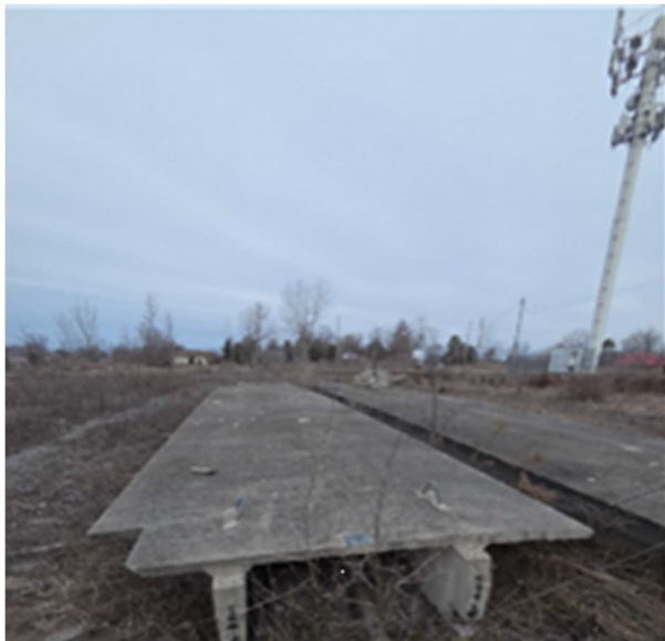
PHOTO 25: View of the concrete platforms located in the field west adjacent to the Phase One Property, within the Study Area, the 5G tower can be seen, facing west.
