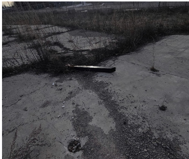
Photo 3: View of a destroyed well, near the central south limit of the Phase One Property, facing southeast.
