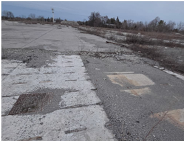
PHOTO 19: View of a catch basin located near the central portion of the Phase One Property, the 5G town can be seen in the distance, facing west.
