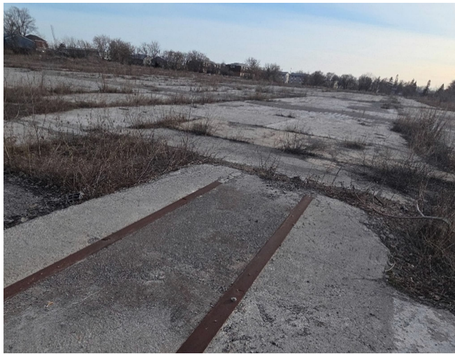
Photo 1: View of former travel lift lines near the central portion of the Phase One Property, facing east.
