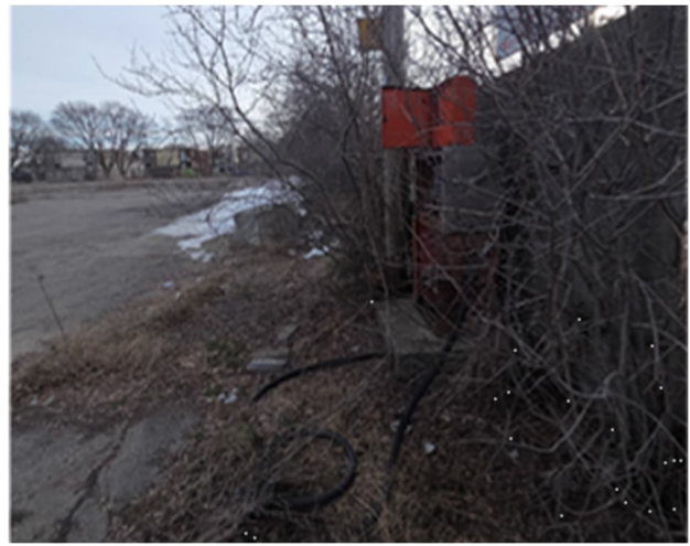
PHOTO 8: Side view of abandoned fuel pump located at the eastern portion of the Phase One Property, facing east.
