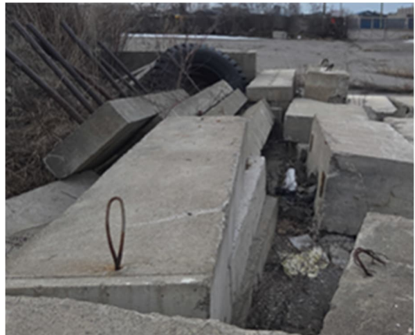
PHOTO 14: View of concrete block debris located west adjacent to the fill pile shown in Photo 16, near the central north portion of the Phase One Property, facing south.
