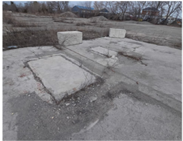
PHOTO 18: View of the raised concrete platform with three (3) cutouts located southwest of the fill piles, that can be seen in the top portion of the photograph, facing north.
