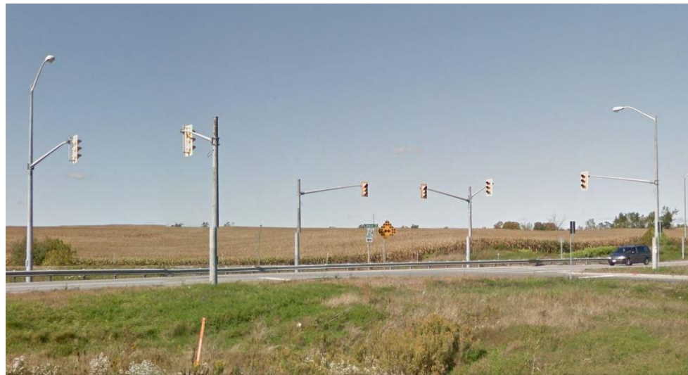
Photo 2: Traffic Signals at Highway 403 Westbound Off-Ramp
