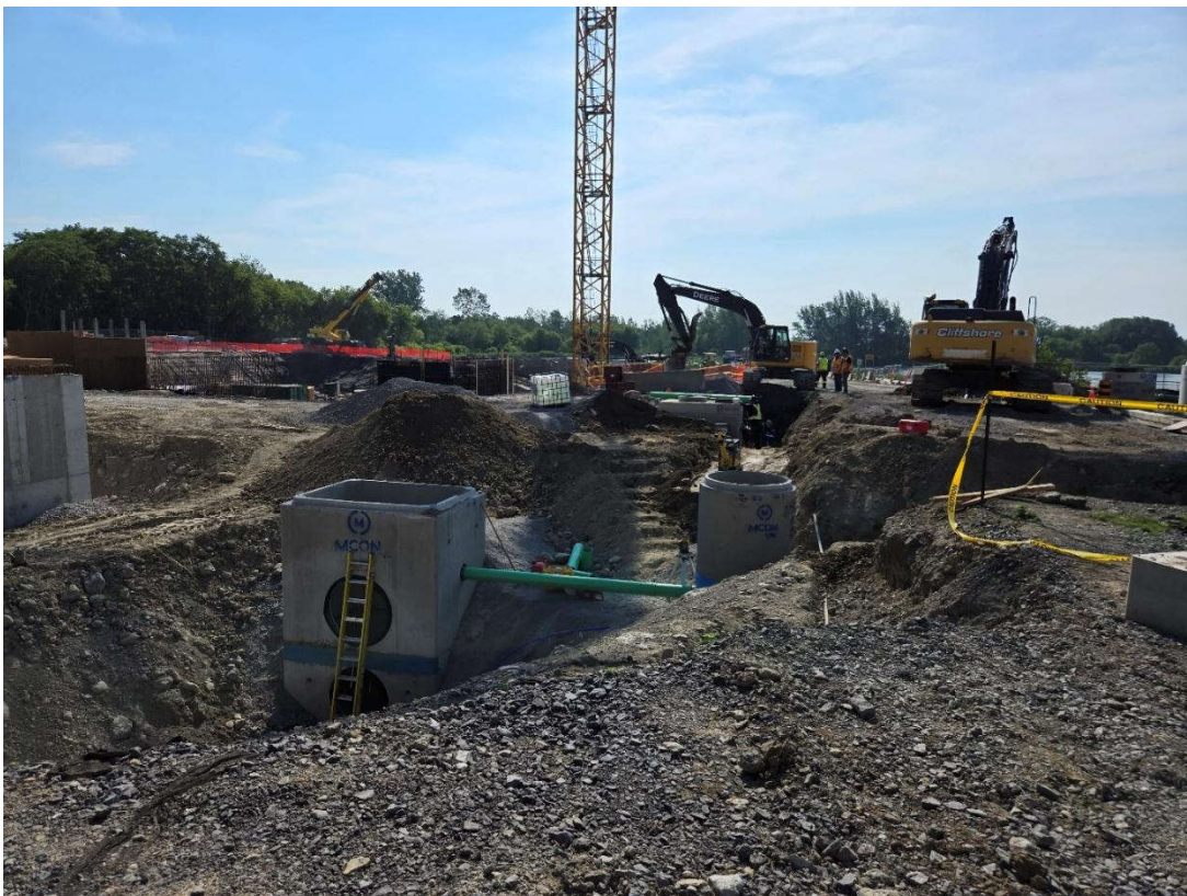
Photo 7: July 14 (manhole installation)
