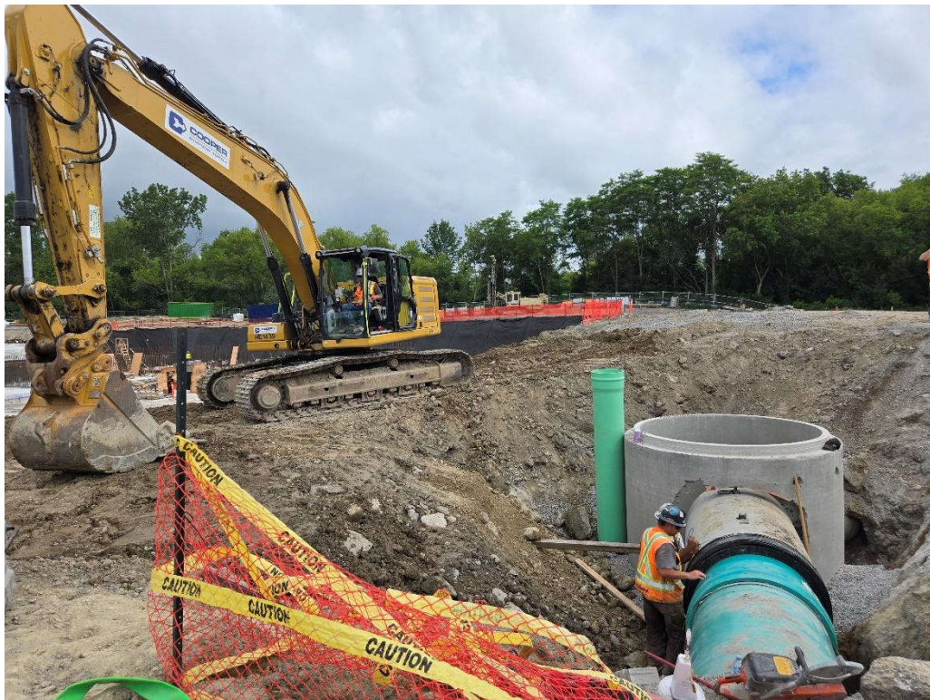
Photo 2: July 7 (manhole installation)
