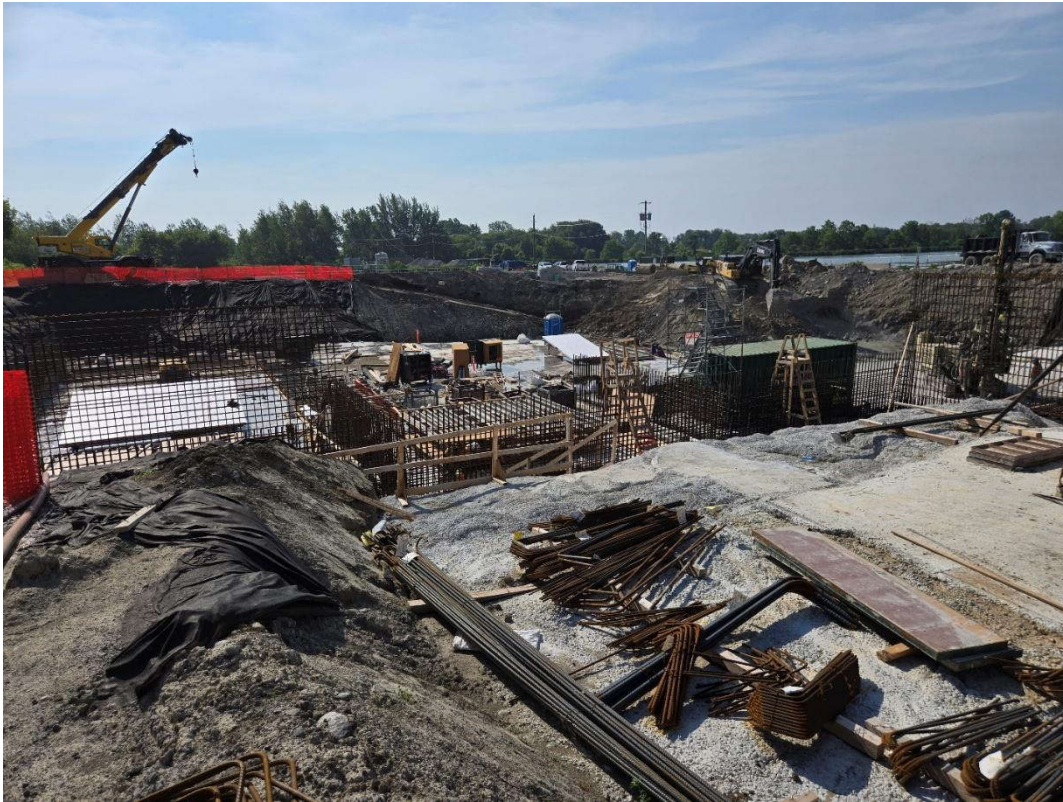
Photo 8: July 14 (aeration tanks and headworks building)
