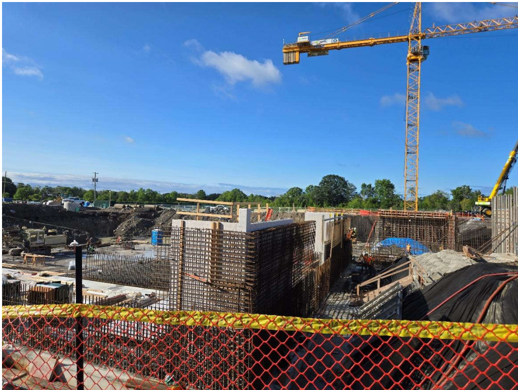
Photo 11: July 22 (aeration tanks)
