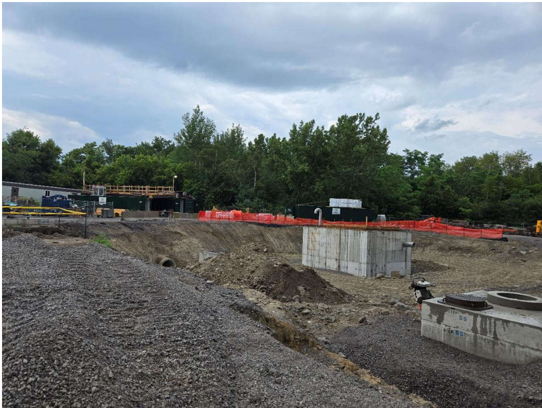
Photo 4: July 9 (pumping station)
