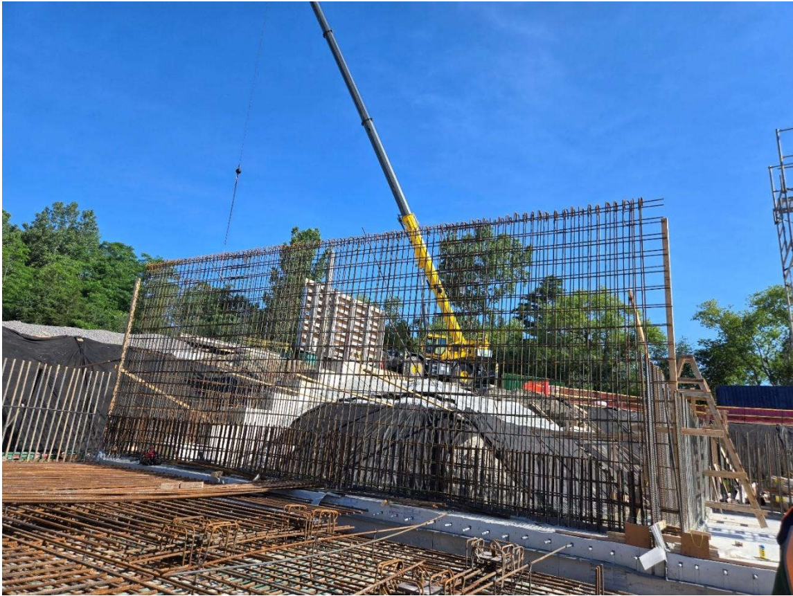
Photo 3: July 8 (aeration tank wall rebar)
