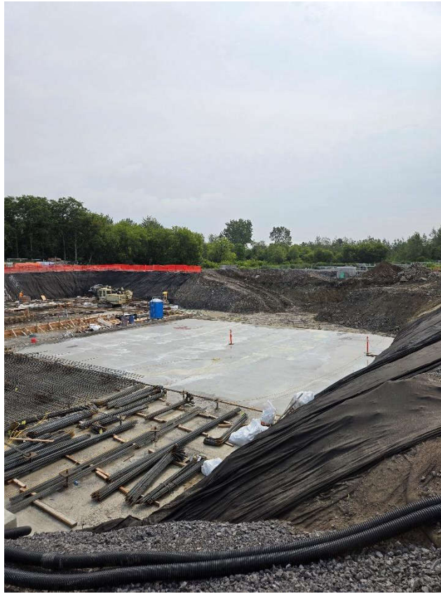
Photo 14: July 28 (clarifier tanks)
