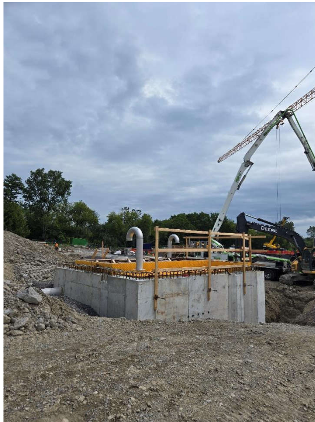
Photo 15: July 29 (pumping station)
