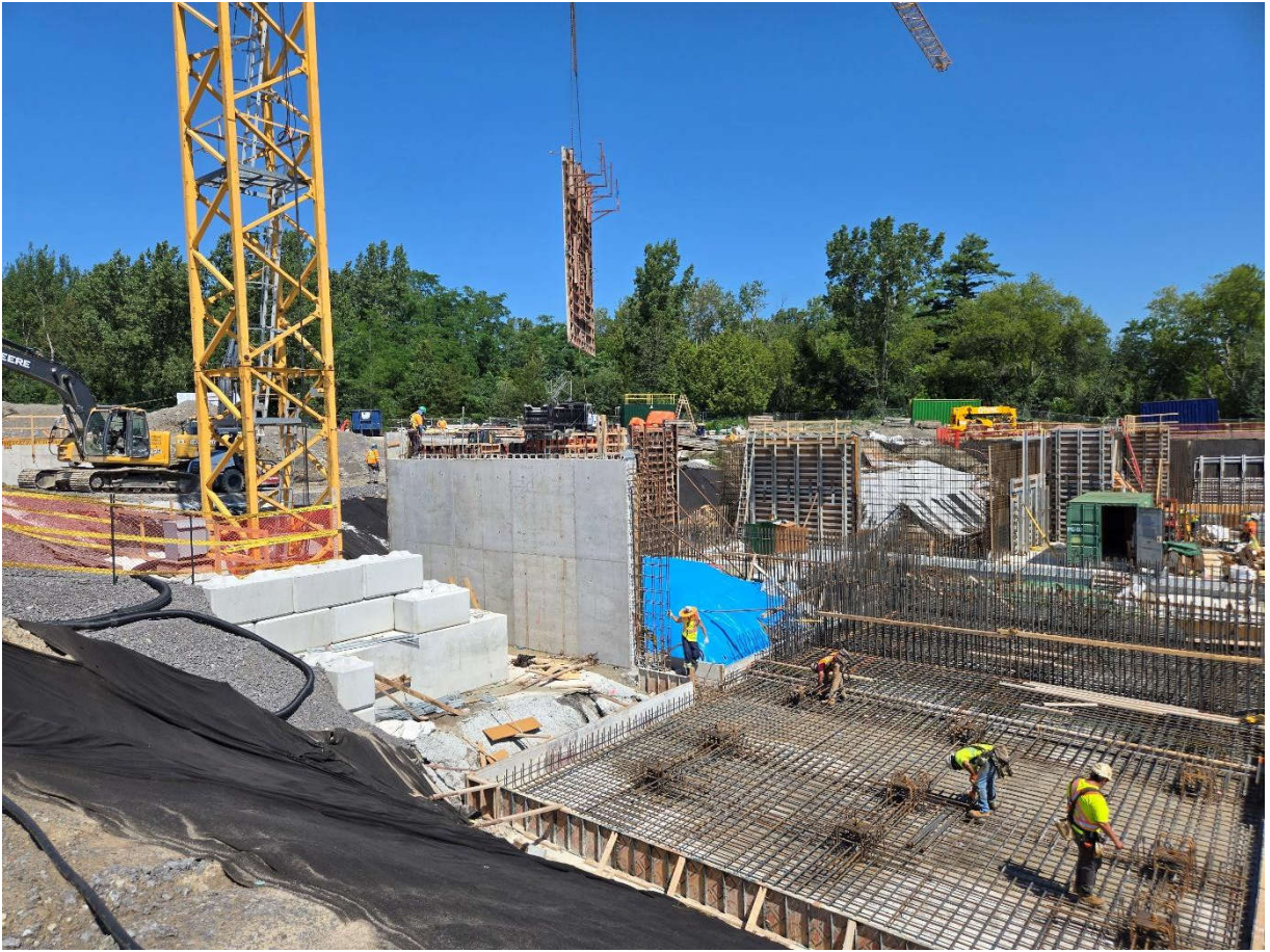
Photo 16: August 4 (aeration and clarifier tanks)
