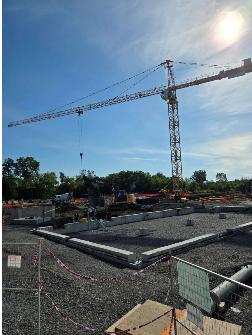
Photo 5: July 10 (admin building)
