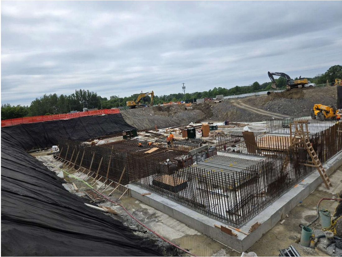
Photo 1: July 6 (aeration tanks)
