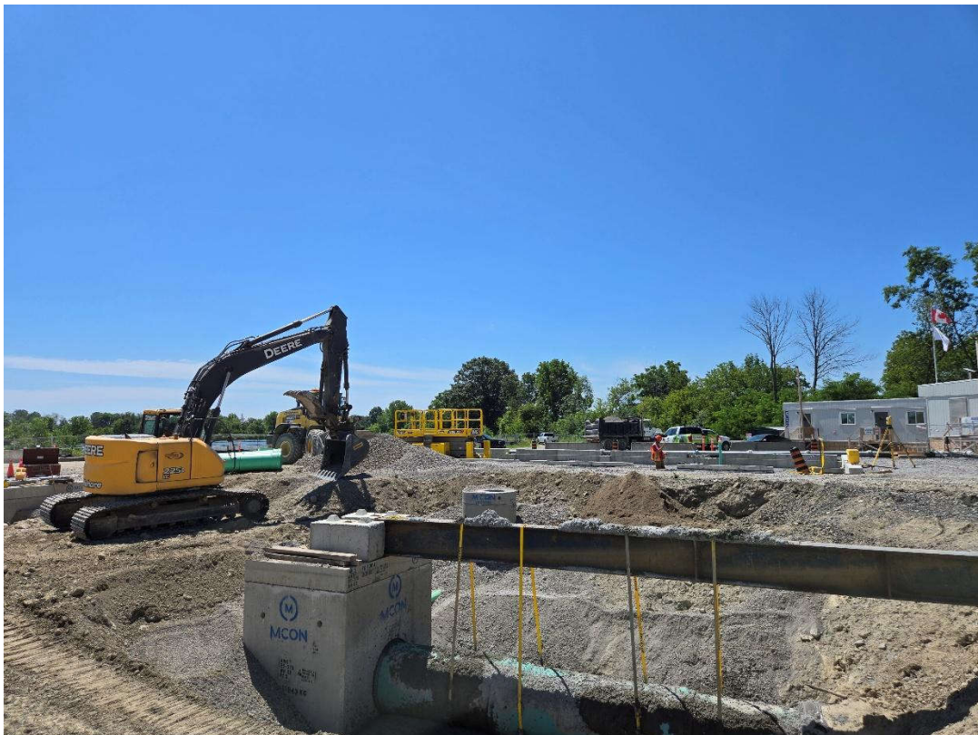
Photo 9: July 17 (manhole and piping installation)
