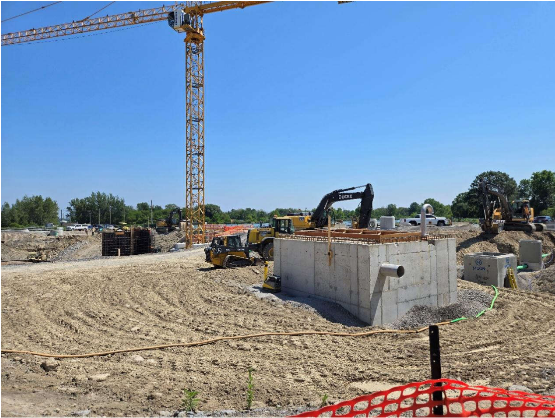
Photo 6: July 13 (pumping station)
