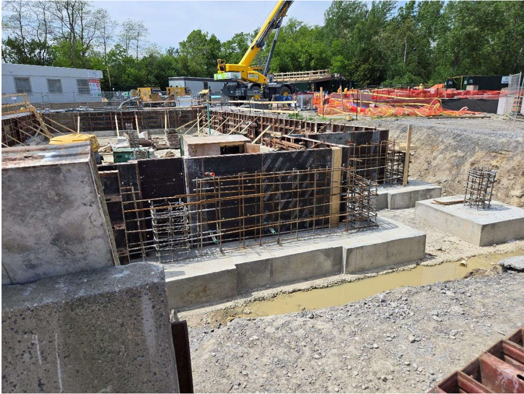
Photo 1: June 4 (admin building)
