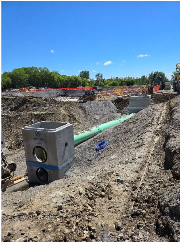
Photo 14: June 23 (manhole and pipe installation)
