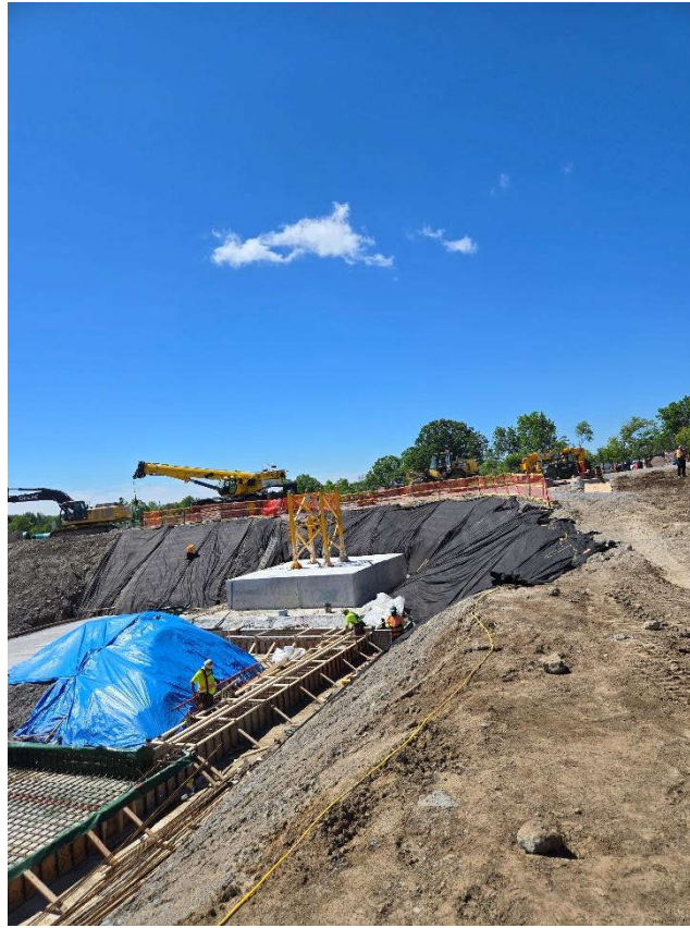
Photo 13: June 23 (tower crane)
