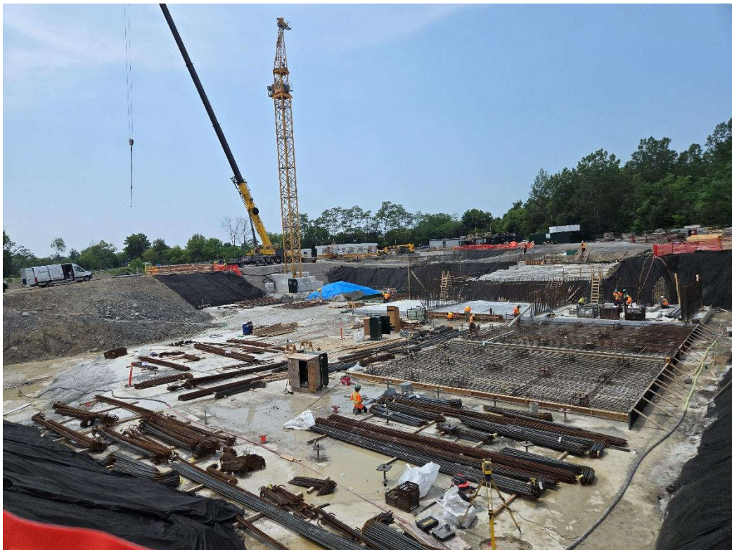
Photo 16: June 30 (tower crane, aeration and clarifier tanks, headworks and UV building)
