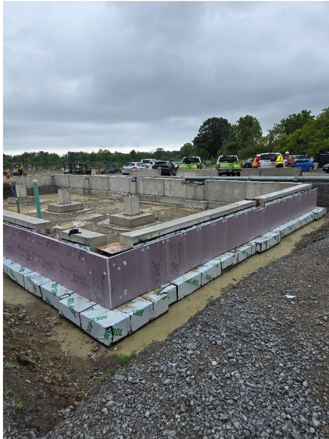
Photo 15: June 26 (admin building)
