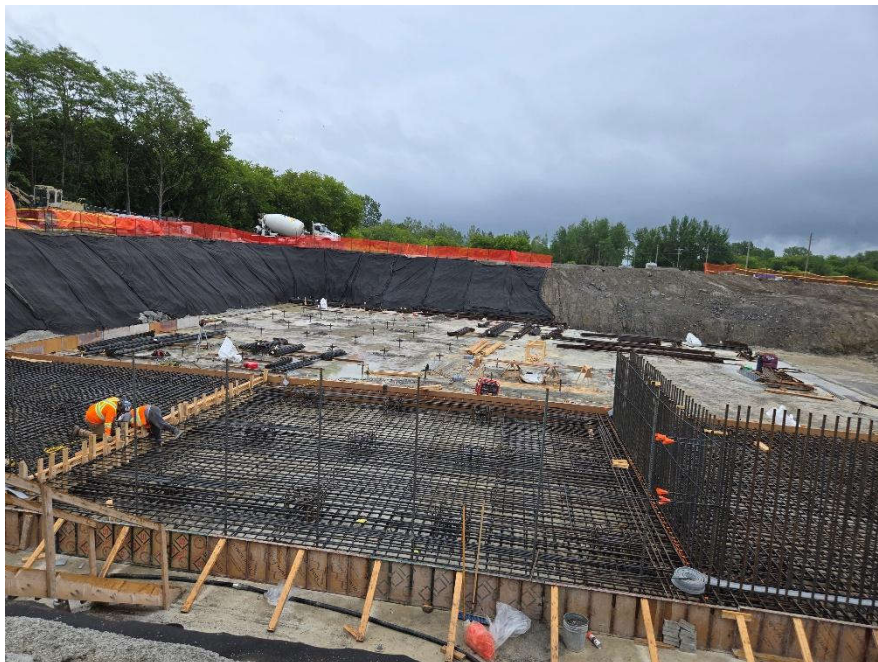
Photo 12: June 22 (headworks building and aeration tanks)
