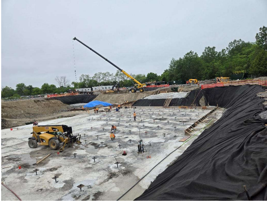
Photo 3: June 10 (aeration tanks)
