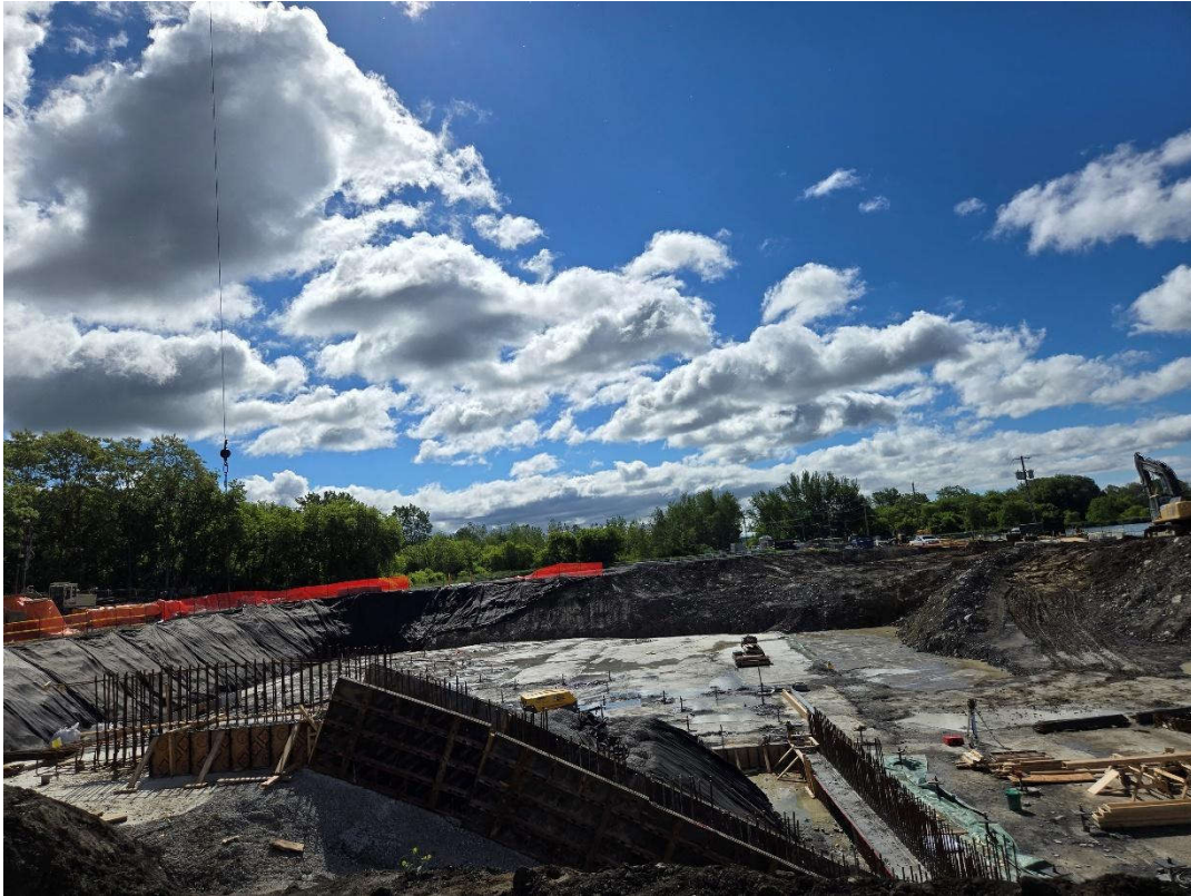
Photo 7: June 15 (aeration tanks and headworks building)
