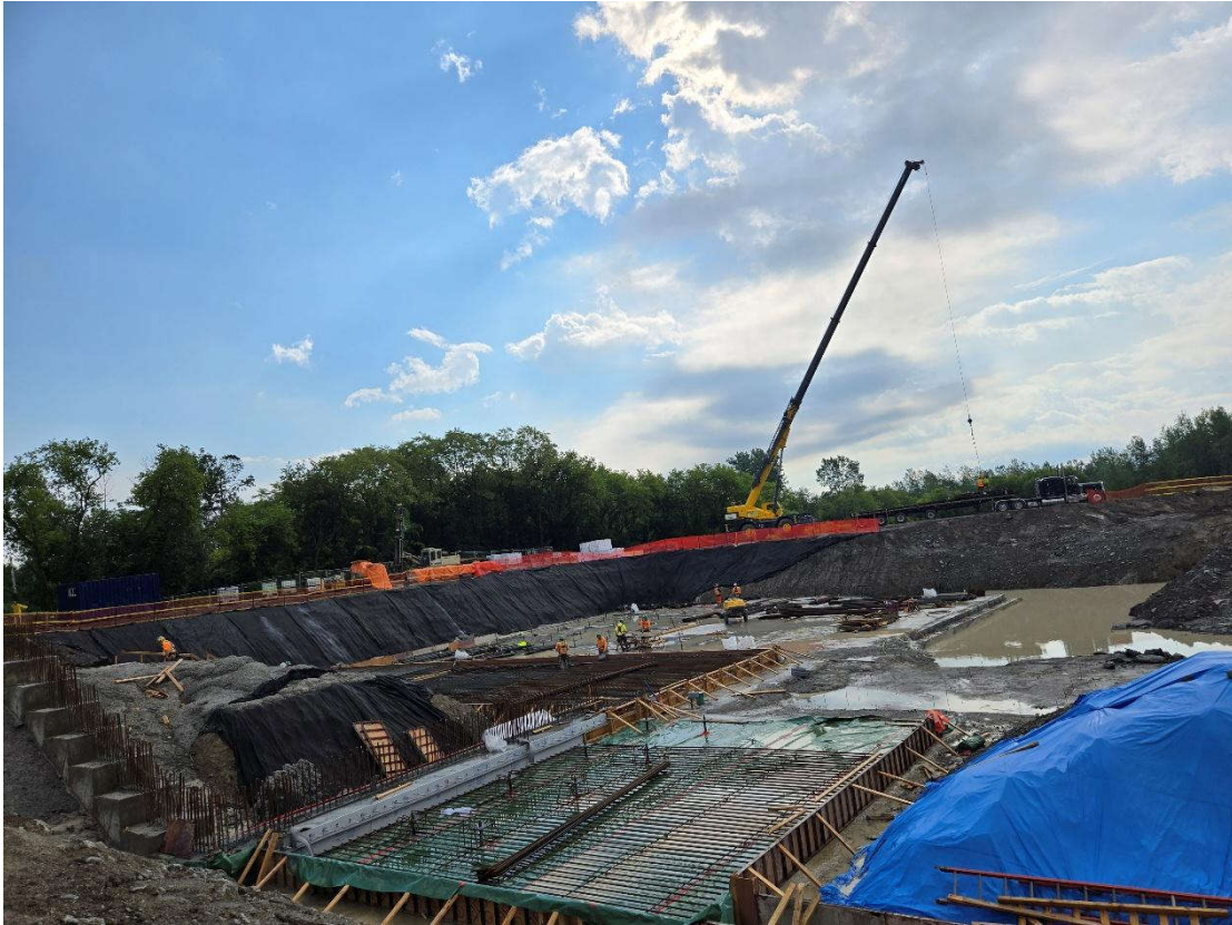
Photo 9: June 18 (aeration tanks, headworks building)
