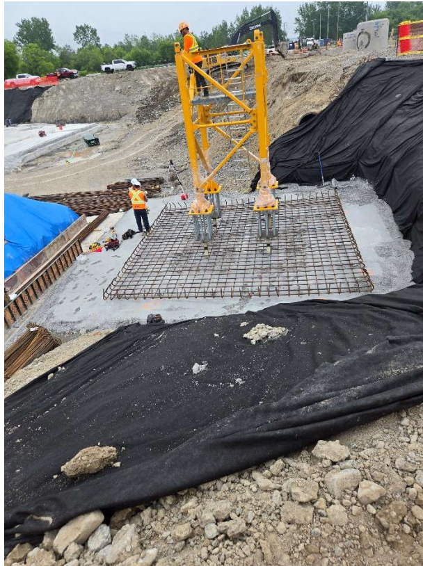
Photo 4: June 10 (tower crane)
