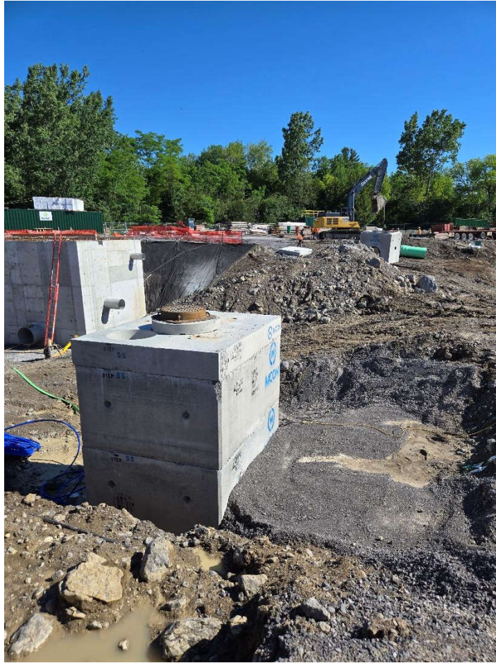
Photo 11: June 19 (pumping station and manhole)
