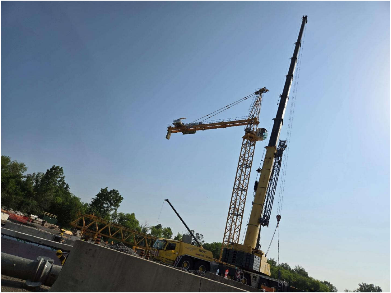
Photo 17: June 26 (tower crane)
