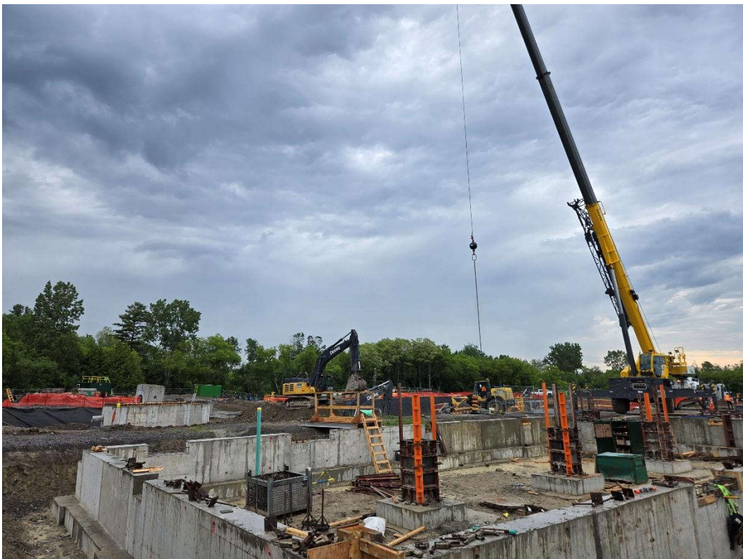
Photo 8: June 17 (admin building)
