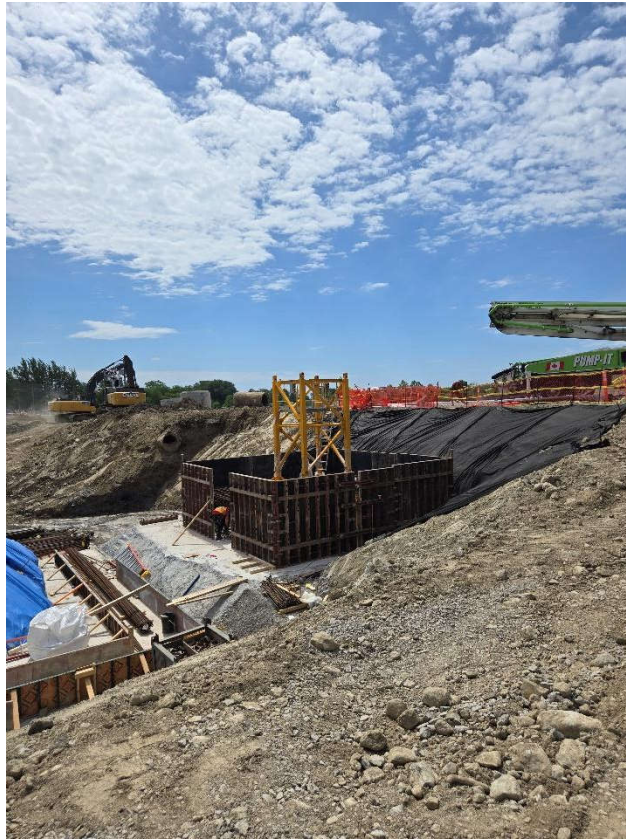
Photo 5: June 12 (tower crane)
