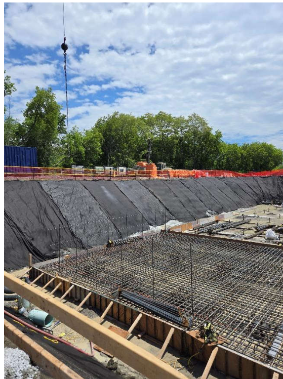
Photo 10: June 18 (headworks building)
