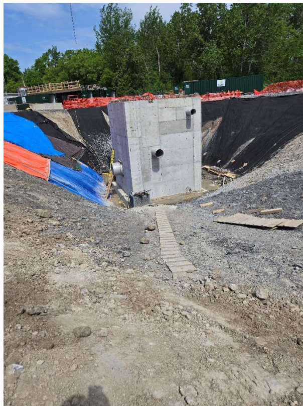
Photo 2: June 5 (pumping station)
