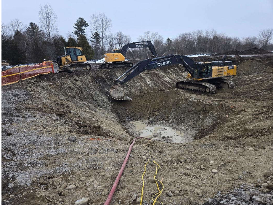
Photo 7: March 3 (pumping station)
