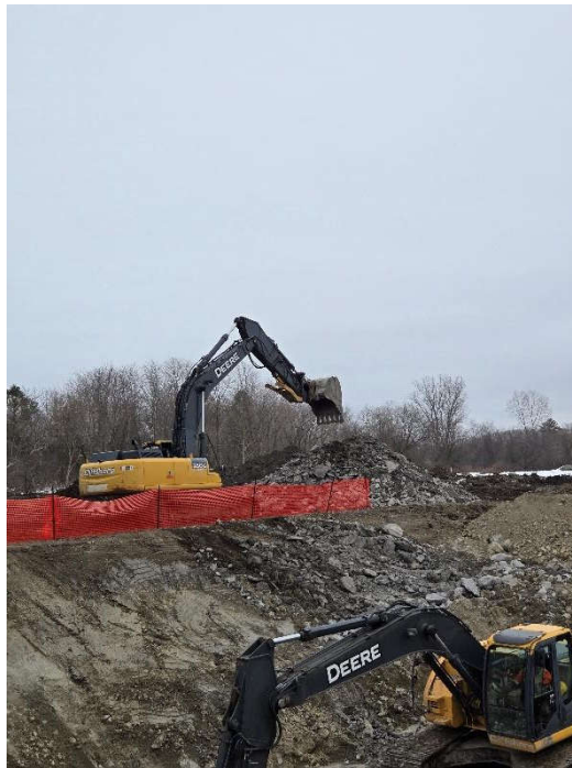
Photo 10: March 6 (pumping station)
