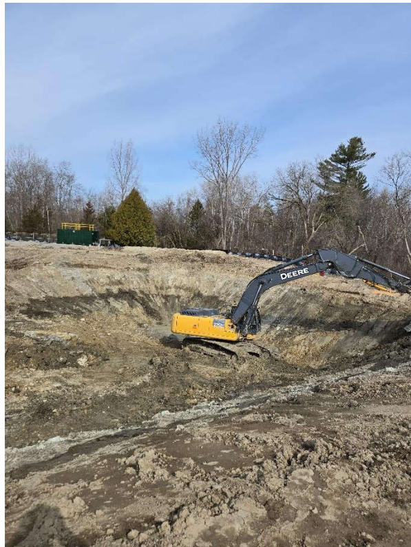
Photo 8: March 30 (aeration tanks)
