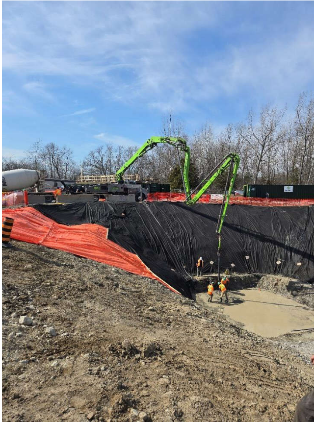
Photo 5: March 30 (pump station)
