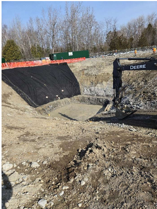
Photo 2: March 30 (pump station)
