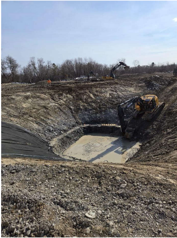
Photo 1: March 30 (pump station)
