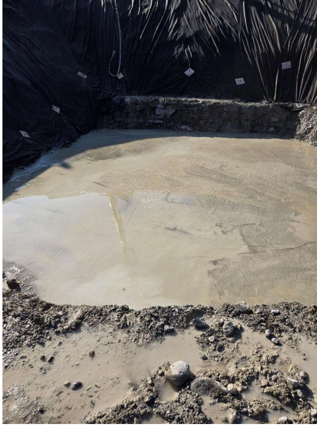
Photo 7: March 30 (pump station)
