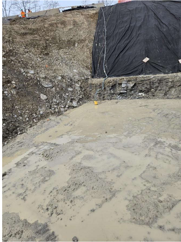
Photo 3: March 30 (pump station)
