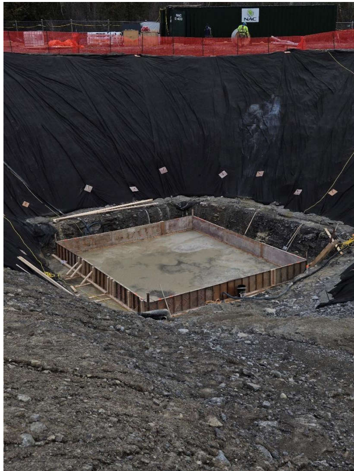
Photo 16: April 2 (pumping station baseslab form)
