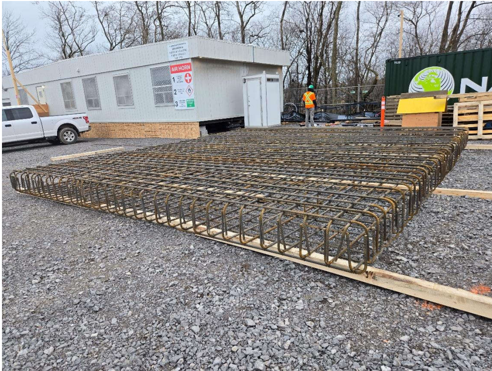
Photo 15: April 1 (pumping station baseslab rebar)
