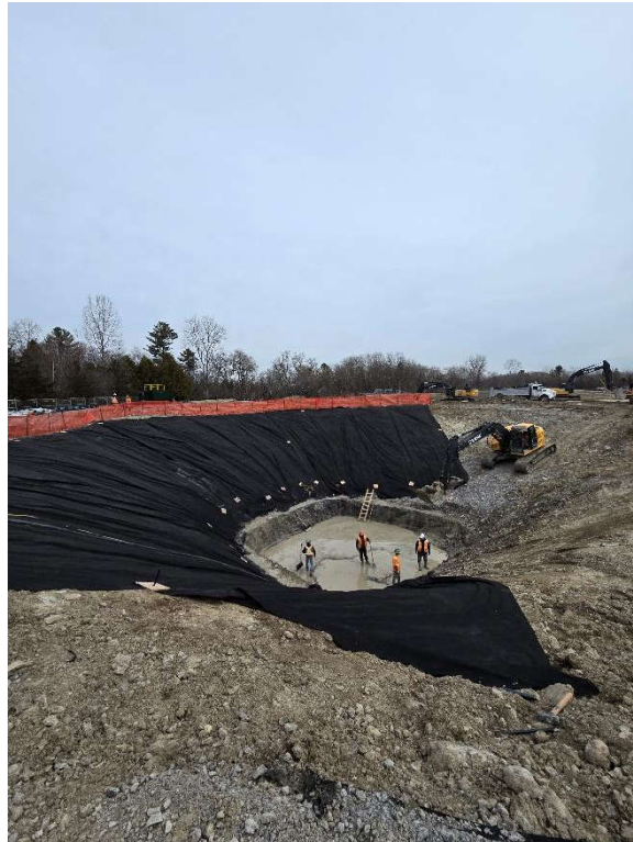
Photo 4: March 30 (pump station)
