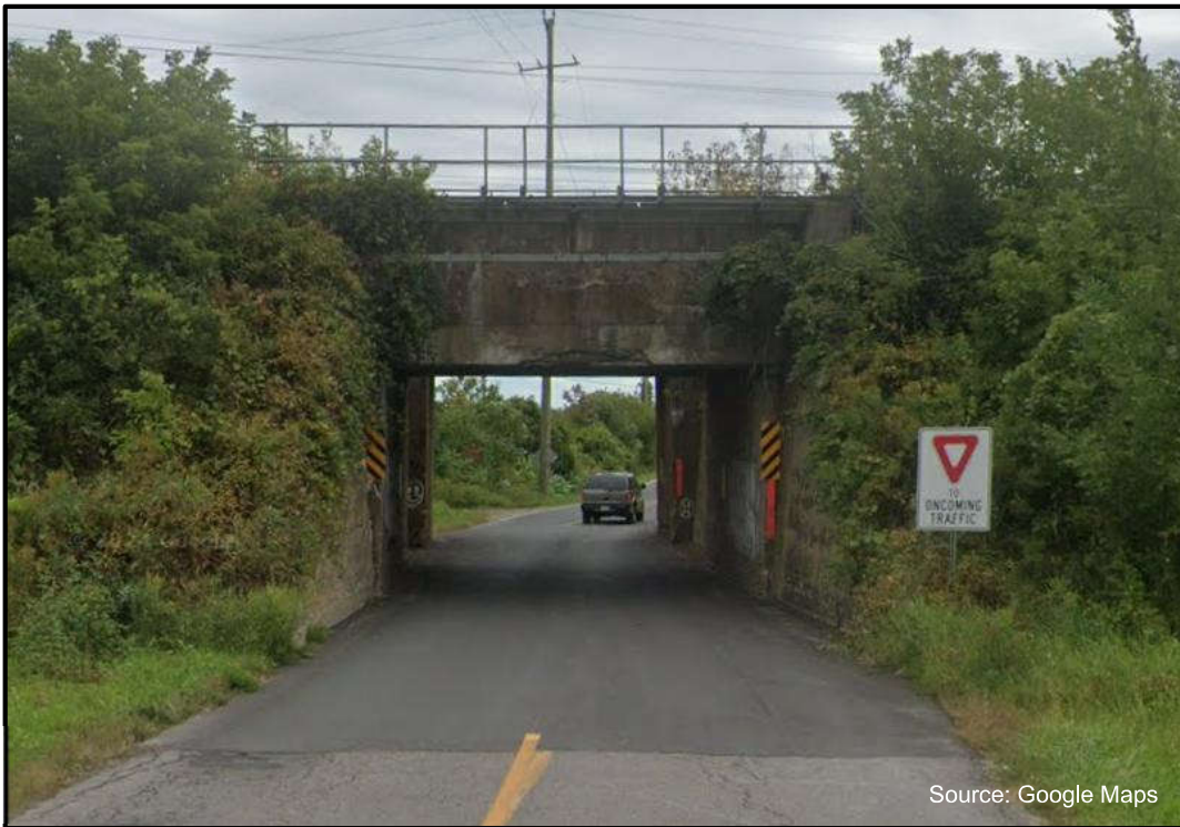
Exhibit 2.9 Boes Road Rail Underpass
