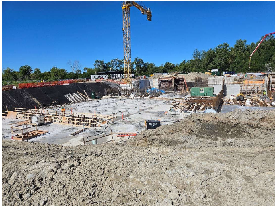
Photo 12: August 28 (rock anchor installation for clarifier tanks)
