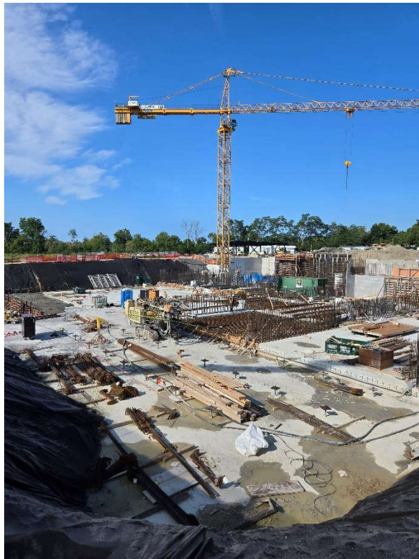
Photo 6: August 21 (clarifier and aeration tanks)
