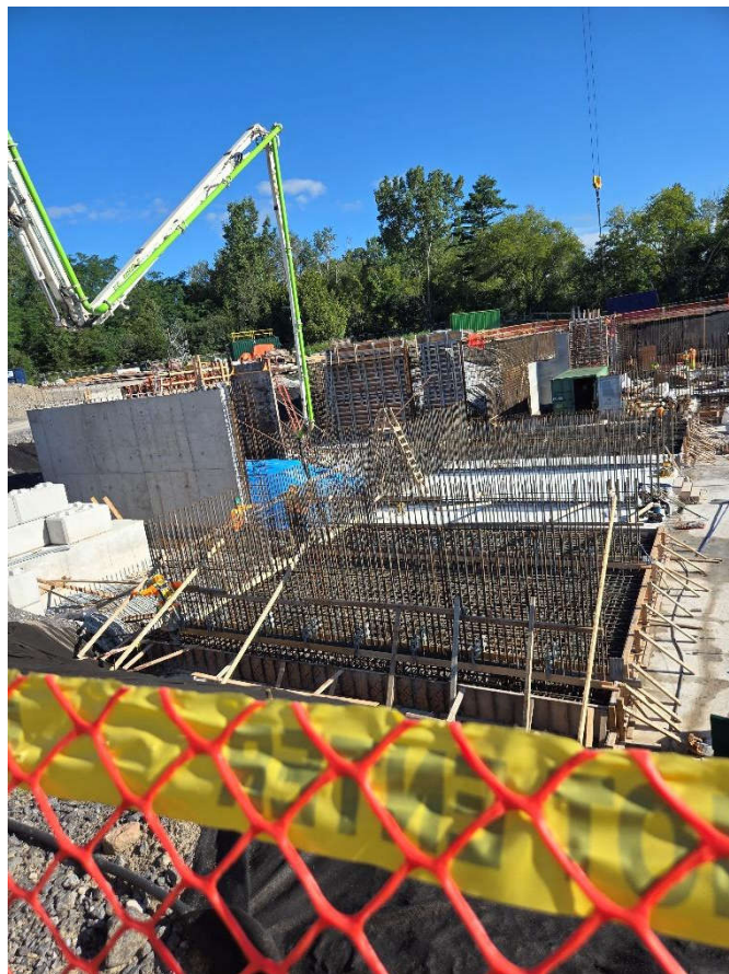
Photo 4: August 18 (tank slab)
