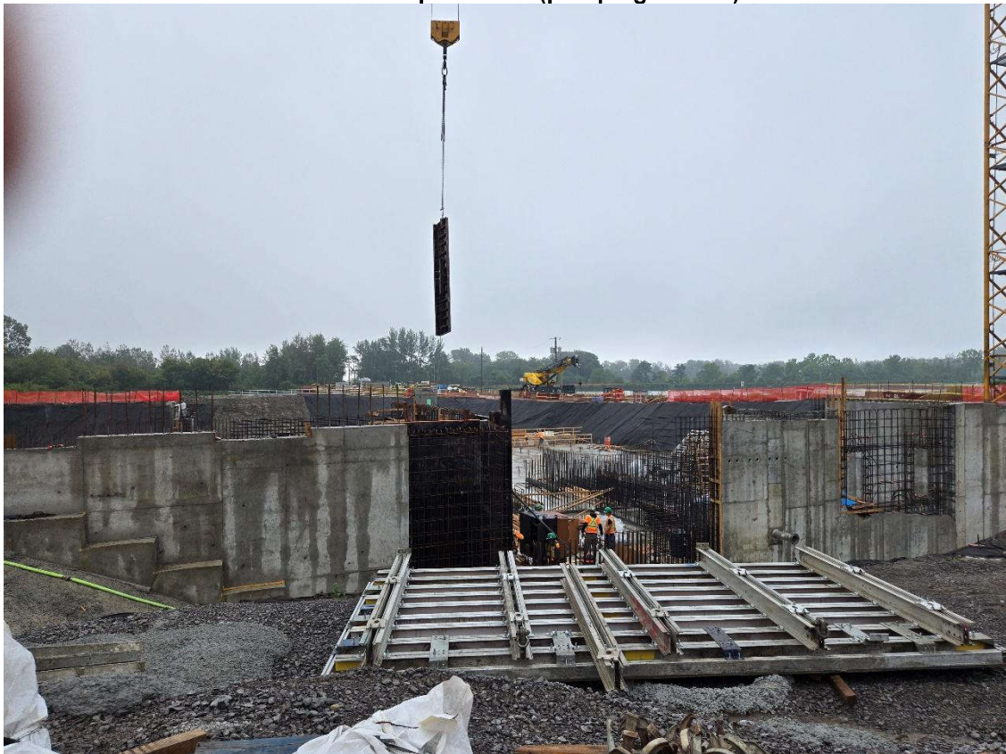
Photo 14: September 2 (clarifier/aeration tanks and headworks/UV building)
