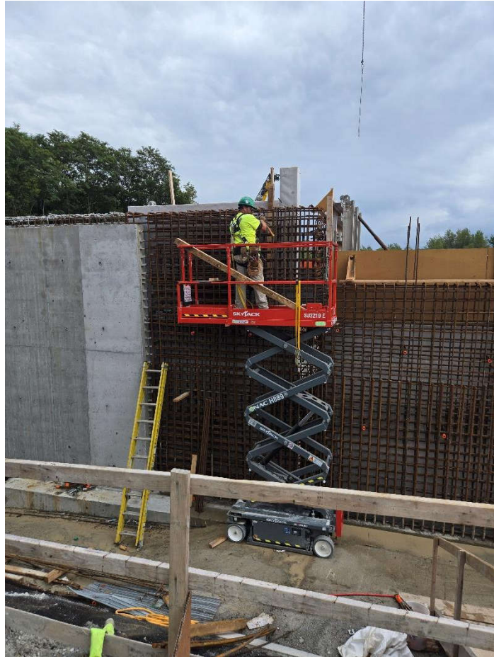
Photo 7: August 24 (aeration tank wall)
