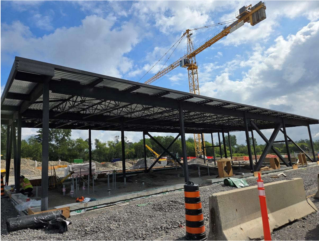
Photo 3: August 17 (admin building)
