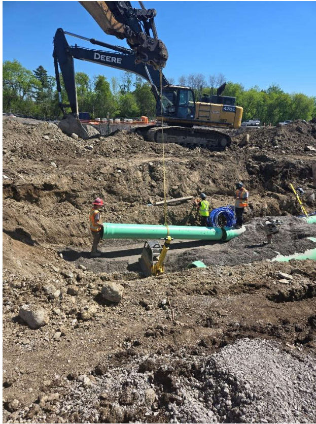
Photo 9: May 26 (sanitary pipe install)
