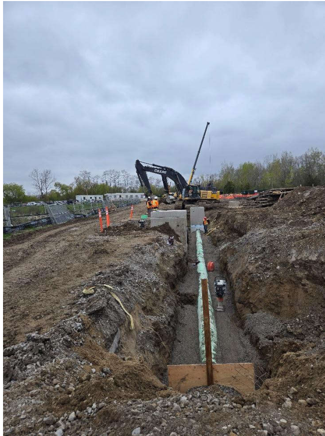
Photo 3: May 14 (trenching, pipe installation and backfilling)
