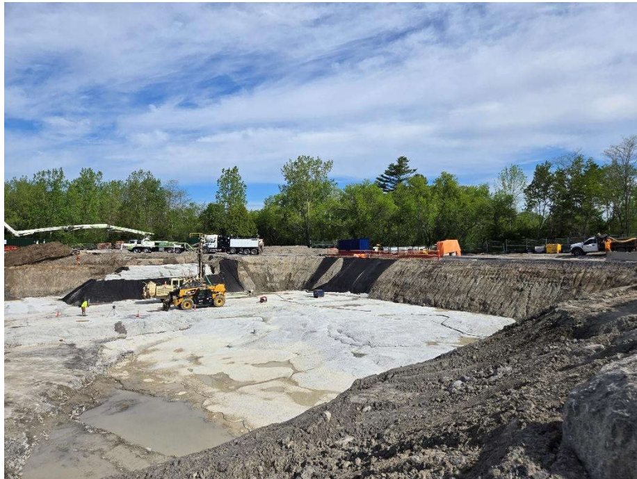
Photo 12: May 27 (aeration tanks)
