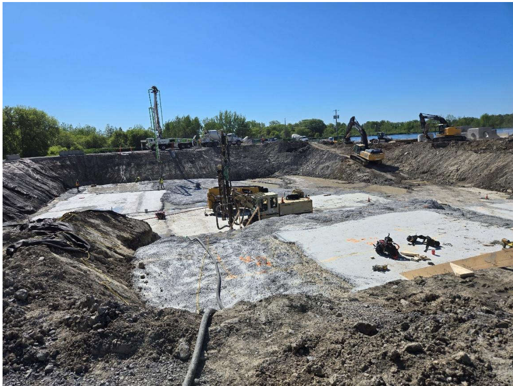
Photo 14: June 1 (headworks and aeration tanks mudslab pour)
