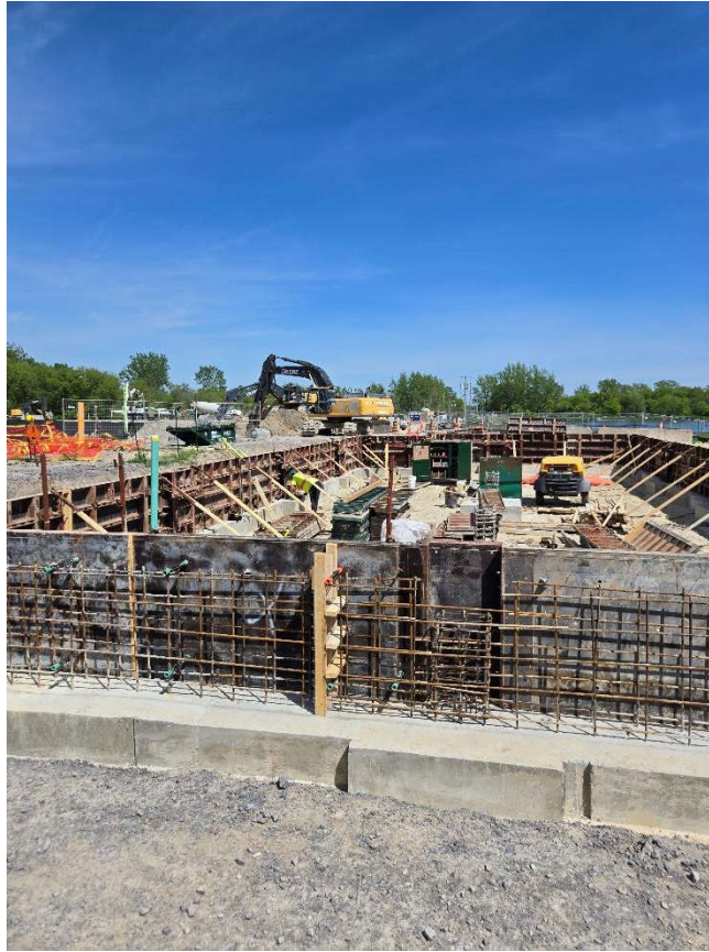
Photo 15: June 2 (admin building)
