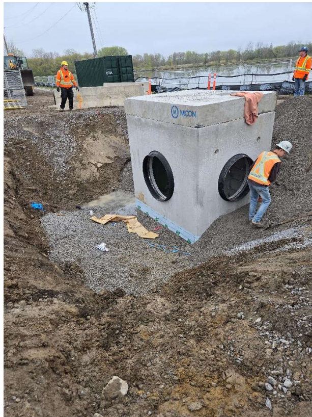
Photo 2: May 14 (manhole installation)
