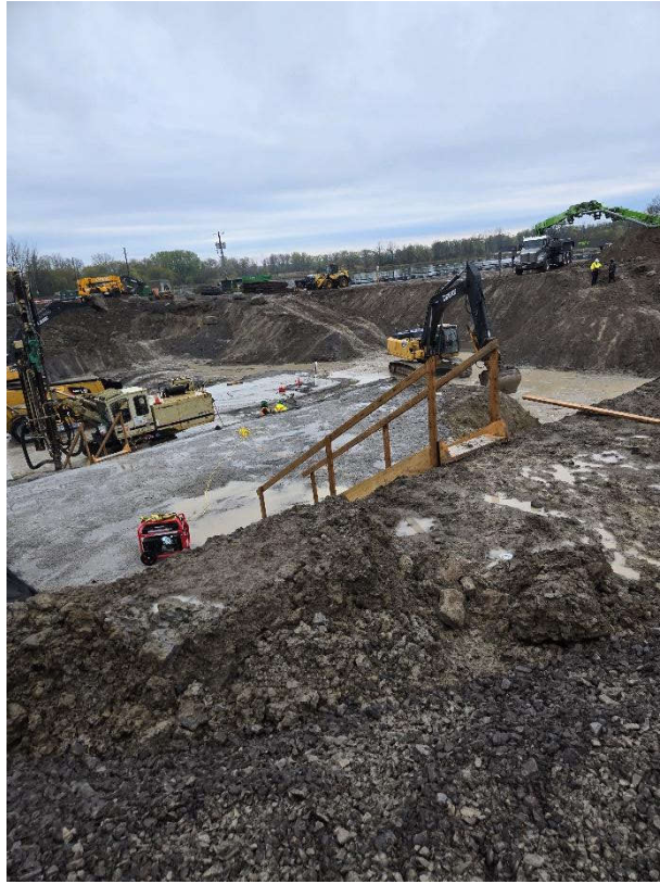
Photo 1: May 13 (aeration tanks)
