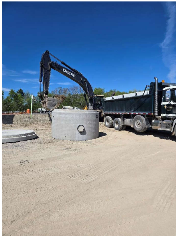
Photo 6: May 21 (excavation – hauling of soil)
