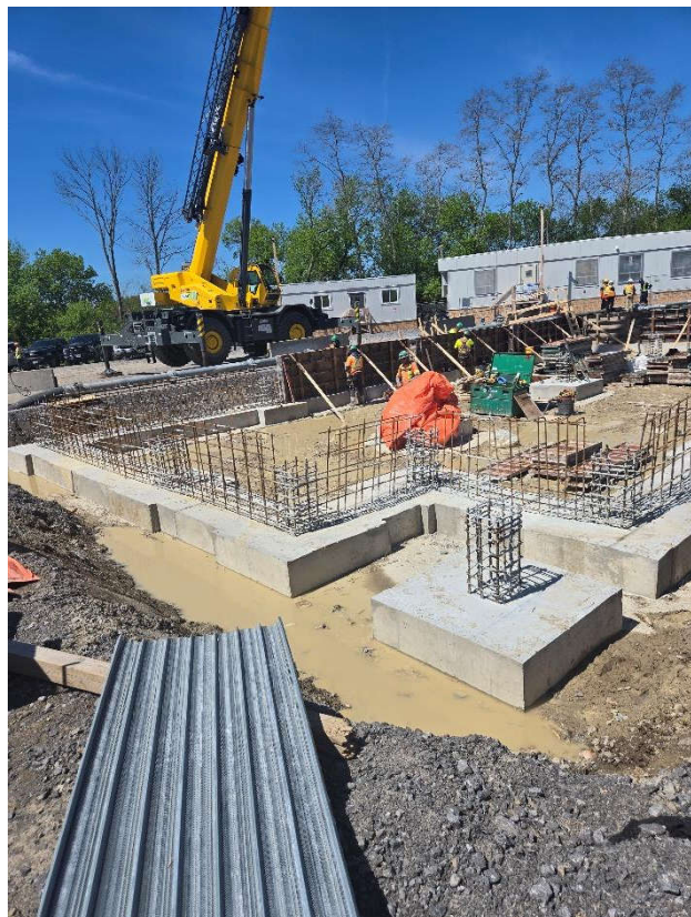
Photo 10: May 26 (admin building foundation)
