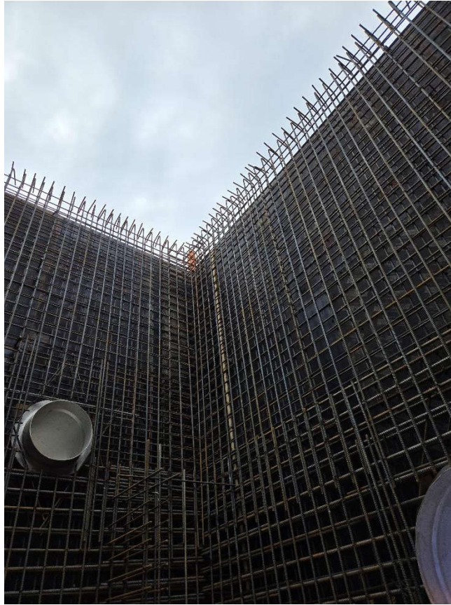
Photo 5: April 21 (pump station)
