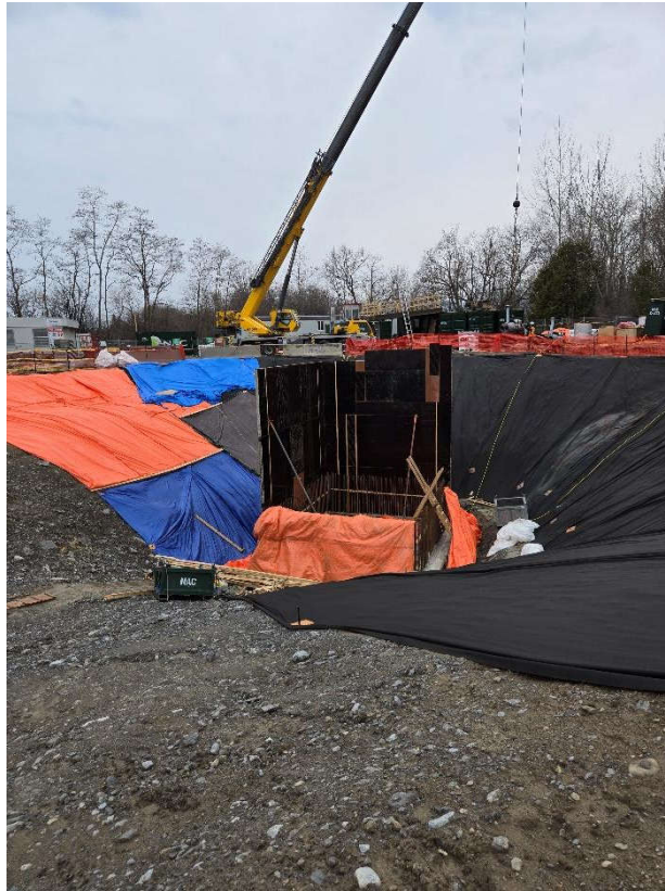
Photo 1: April 10 (pump station)
