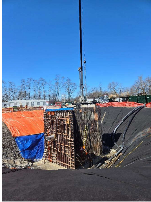
Photo 3: April 17 (pump station)
