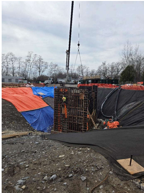
Photo 2: April 13 (pump station)
