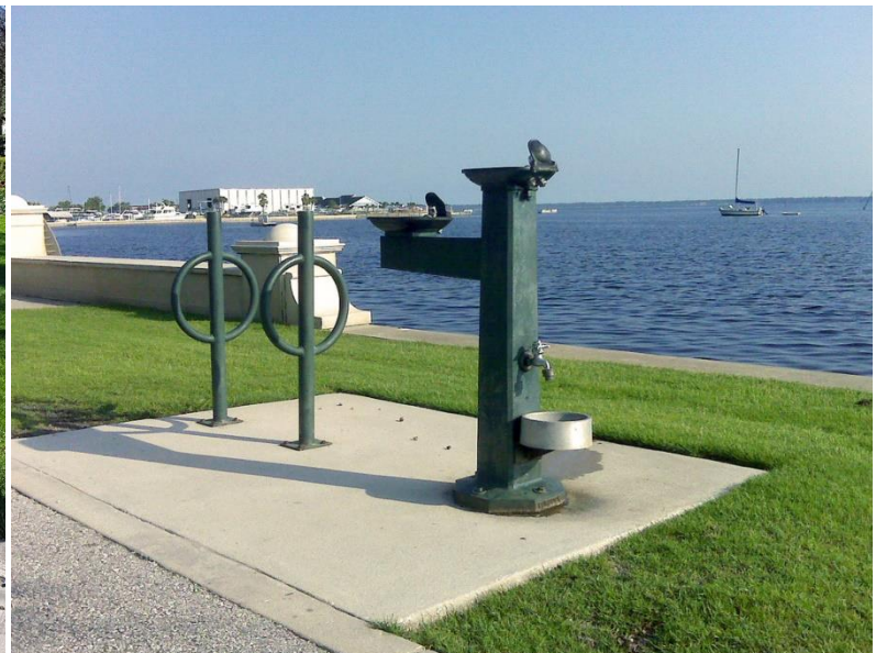
Good = Dual height drinking fountains, provides sufficient knee space to access the drinking fountain. They are well located adjacent to, but out of the path of travel, and have a clear level area in front and underneath. Also has a filling station for dog
