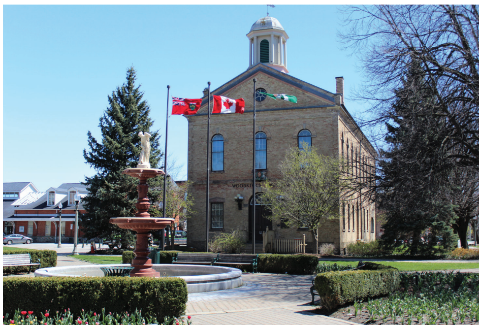
City Hall and the Woodstock Museum are two of the City's key historic buildings.
