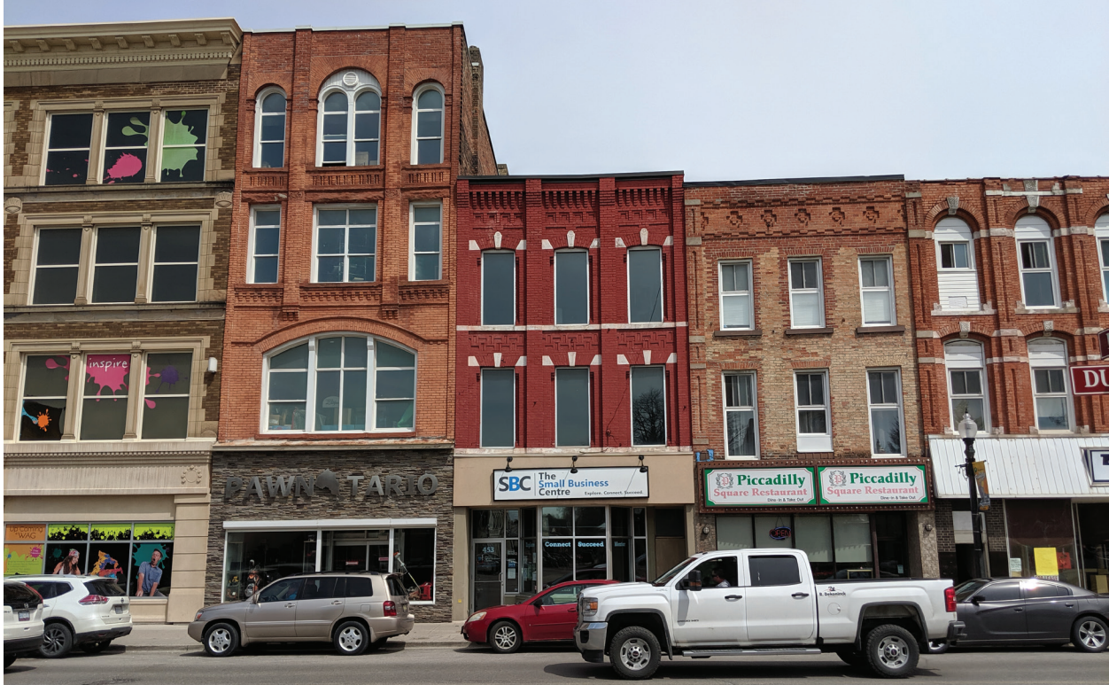
An example of a consistent, heritage streetscape with the new Art Gallery building carefully reflecting the established rhythm and datum lines.
