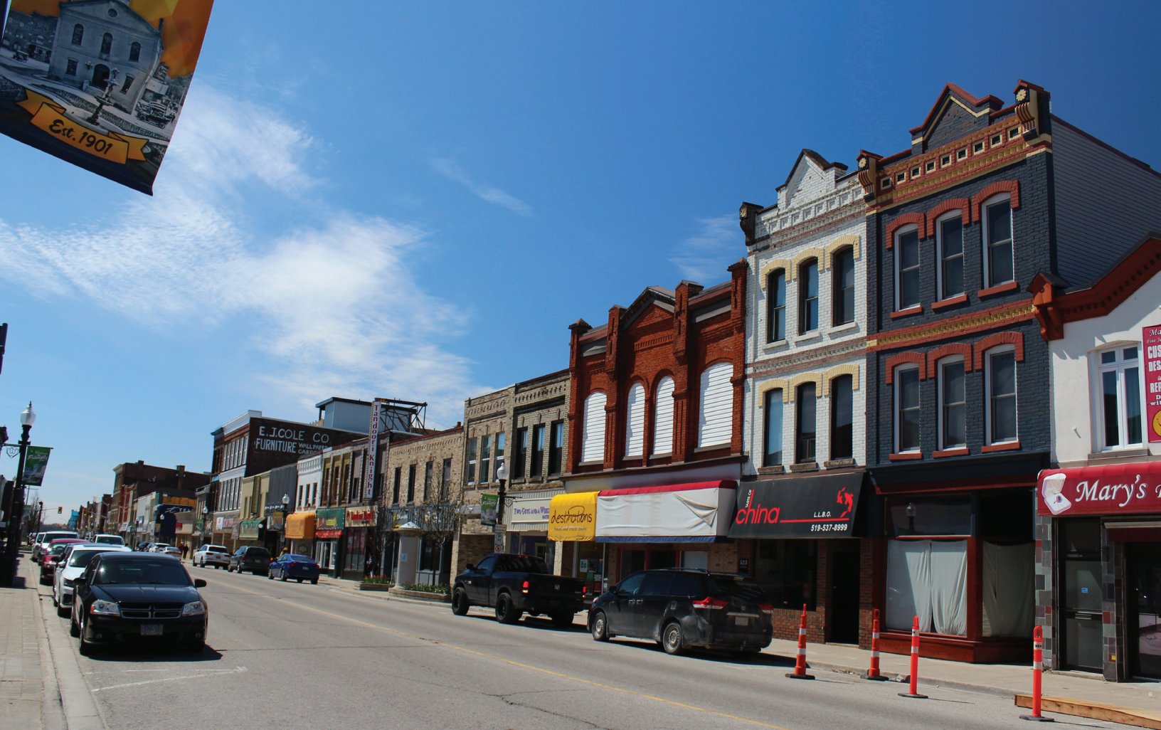
Dundas Street is characterized by a strong core of historic 2 to 3-storey buildings.
