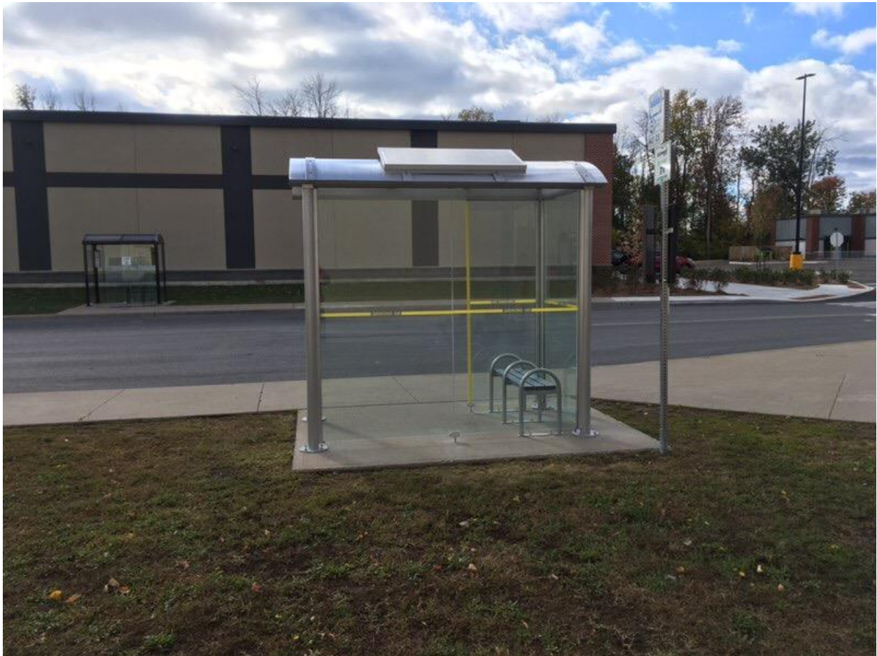
Bus Stop at SmartCentres with New Bus Shelter and Solar Panel – Concrete Pad Connecting to Sidewalk
