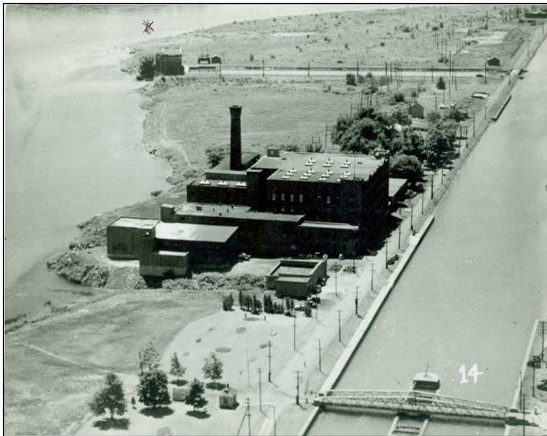
Image 14: Photograph showing the area west of the Augusta Street Swing Bridge with the Stormont Mill in the centre and old powerhouse in the upper left (CCM 2015).
