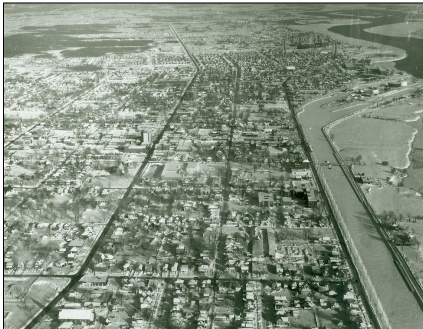
Image 13: View east showing the waterfront in the 1950s (CCM 2015). Notice that the area south of the canal has been infilled.
