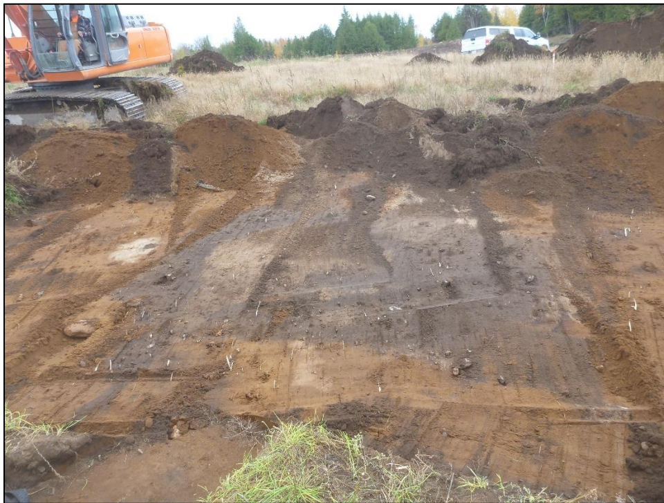
Image 5: Example of a large rectangular sub-surface feature in the process of being uncovered during mechanical topsoil removal (WSP Canada Inc.).
