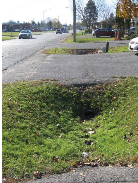
Plate 6: Ditch in the ROW, facing west.
