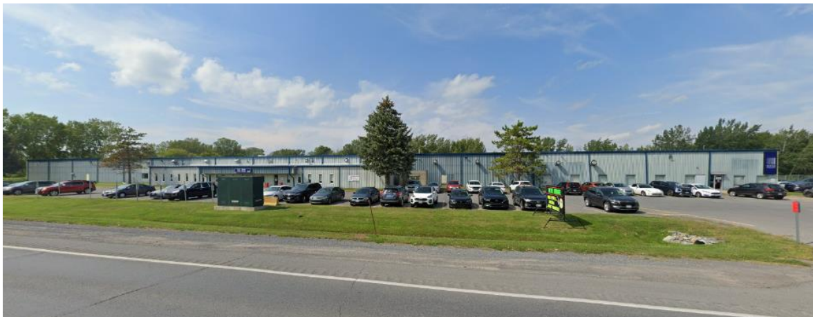
Figure 7 - Street View of 2850-2880 Marleau Road
