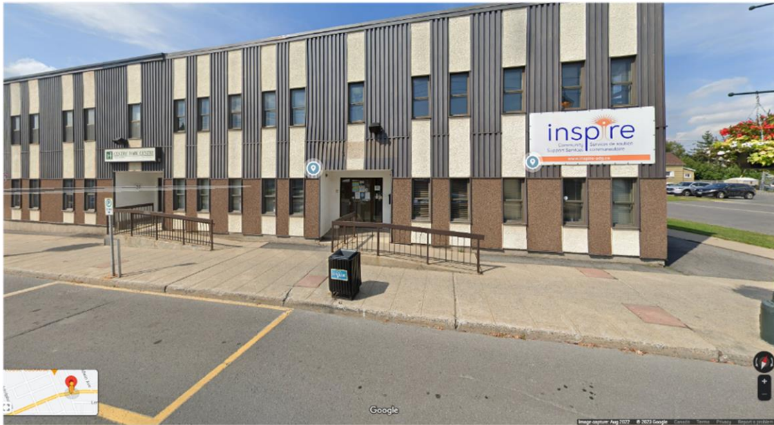
Figure 8 - Street View of 26 Montreal Road
