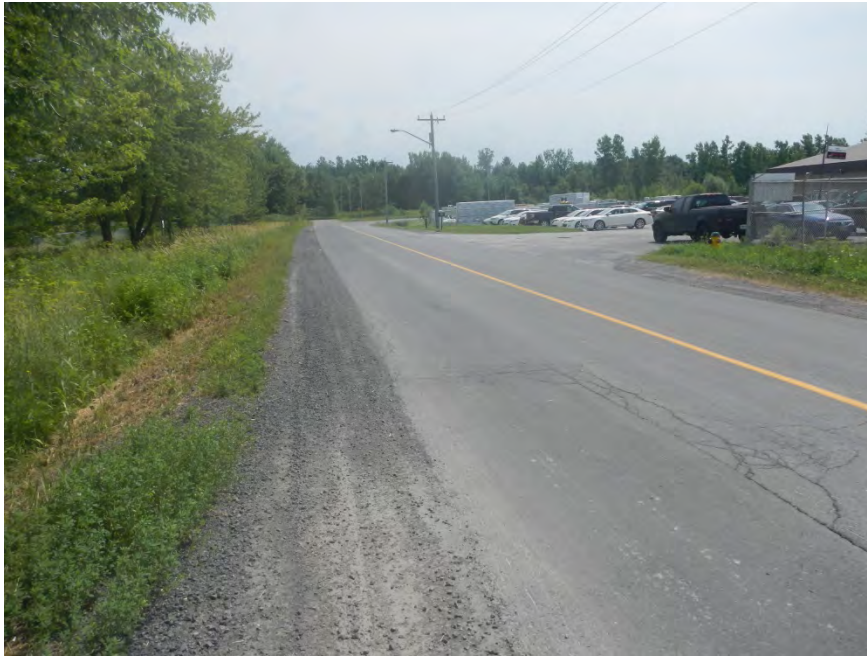
Photo 13. Virginia Drive facing south towards Tenth Street East.
