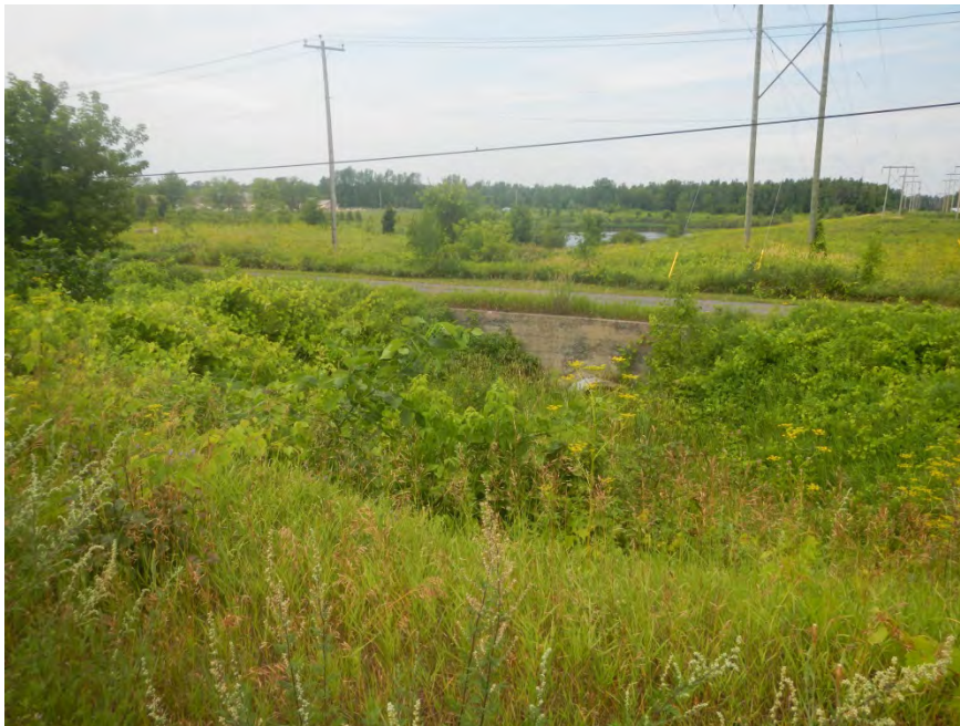
Photo 6. Culvert and stormwater retention pond on North portion of Site.
