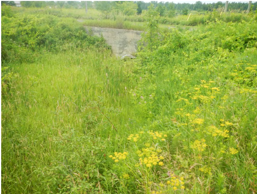
Photo 4. Culvert and seasonal drainage located on the northeast portion of the Site.
