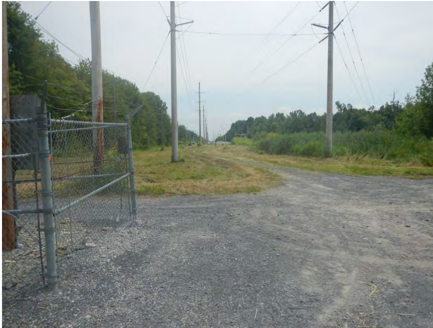
Photo 3. Facing west from hydroline along railway access road.
