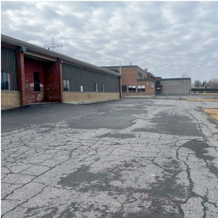
View looking southeast along existing parking lot
