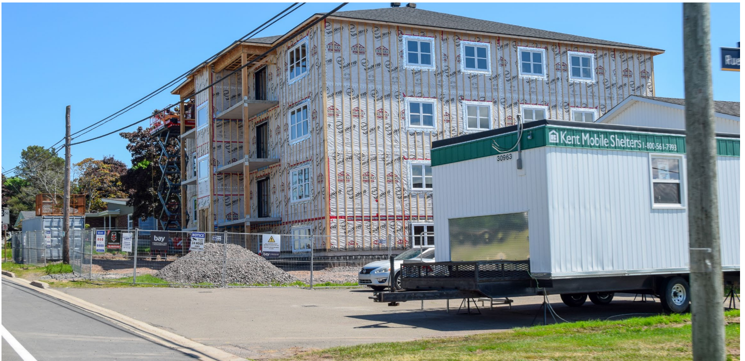
Figure 1: Construction site on Amirault Street.
