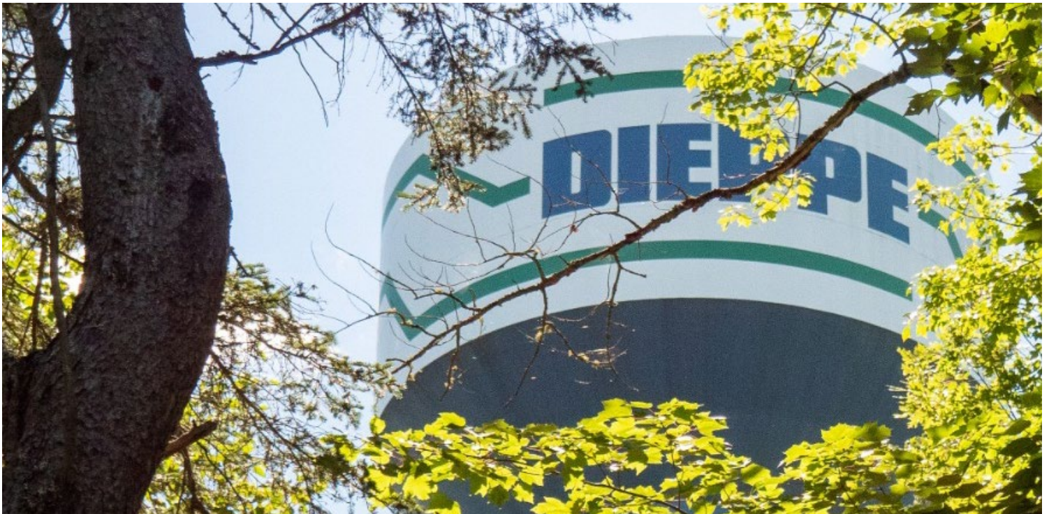
Figure 41: Close-up of the water tower in Dieppe.
