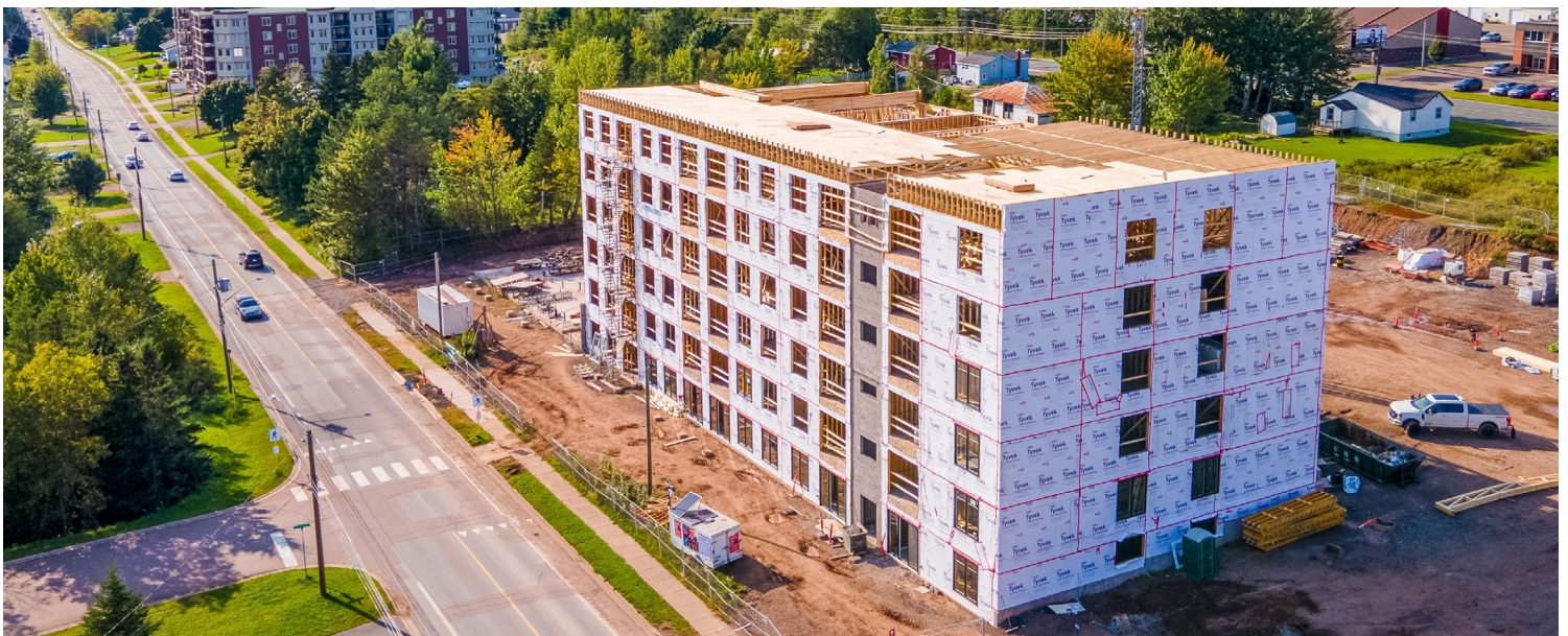
Figure 29: Apartment construction on Gauvin Road.
