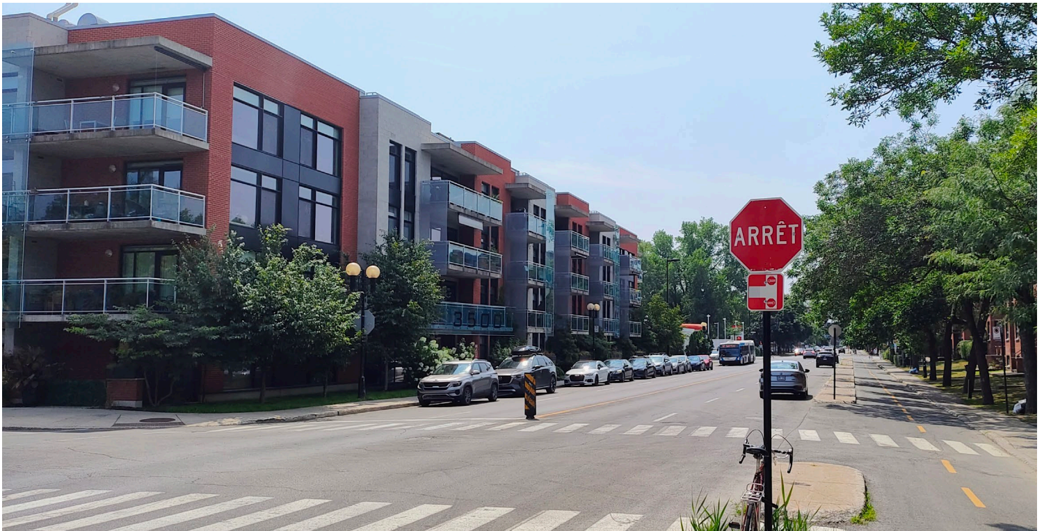
Figure 53: Example of well-designed compact, urban form with appealing streetscape in Montréal.
