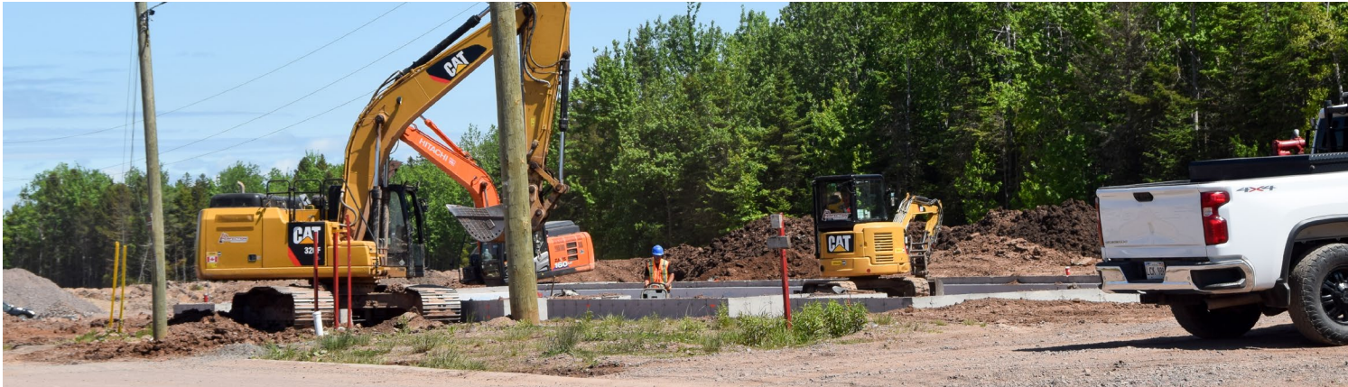
Figure 8: Home construction on Melanie Street
