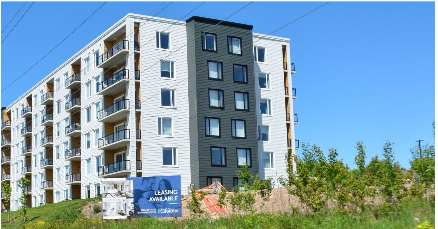
Figure 6: Recently constructed multi-unit dwelling on Dieppe Boulevard
