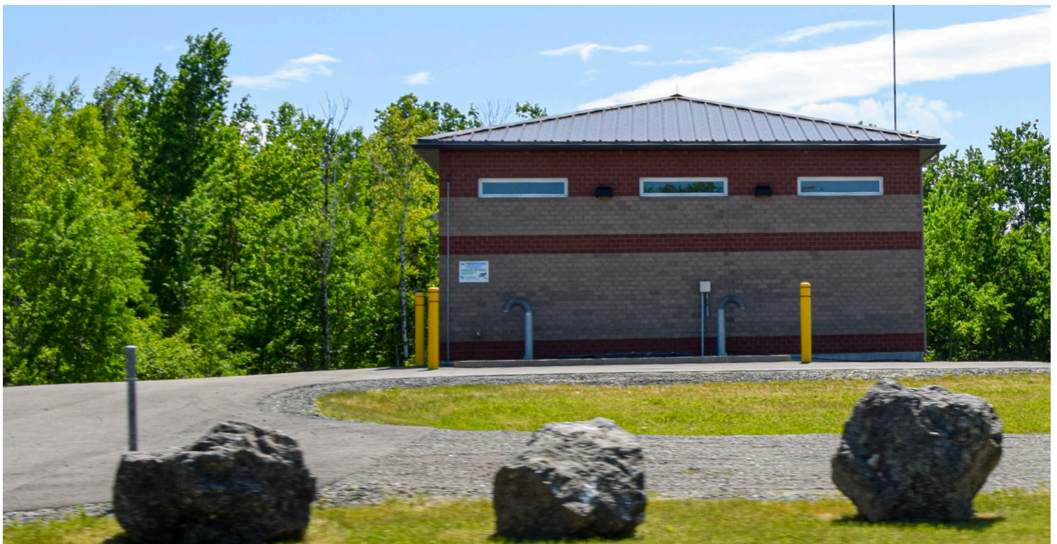
Figure 31: Fox Creek sewage pumping station on Amirault Street
