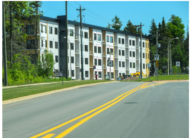
Figure 54: Housing construction in Dieppe.
