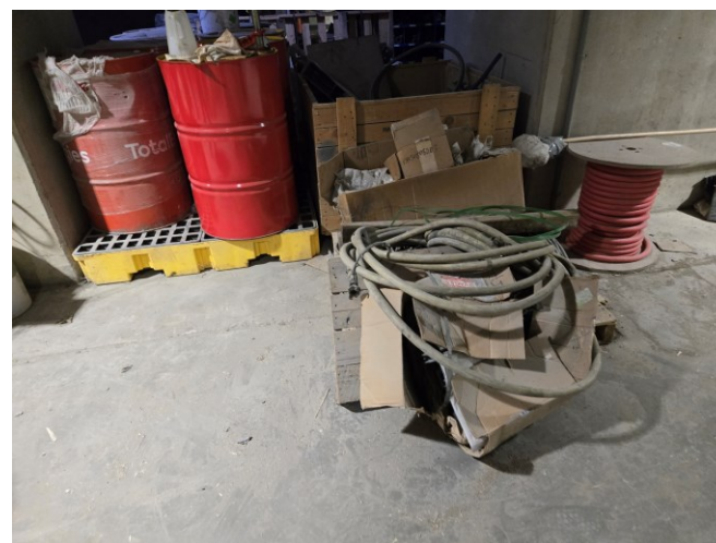
Photo 32: View of hoses in the Boiler Building.
