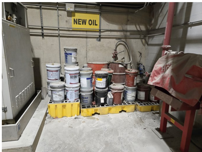
Photo 17: View of the new oil storage area.
