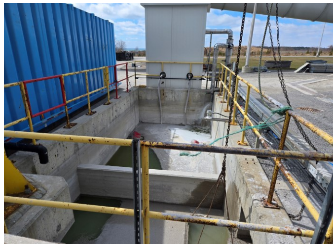
Photo 34: View of the wastewater settling basin.
