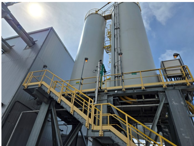
Photo 35: View of Pozzalon and Cement Silos.
