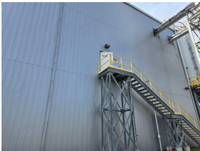
Photo 23: View of open Residue Building Door.
