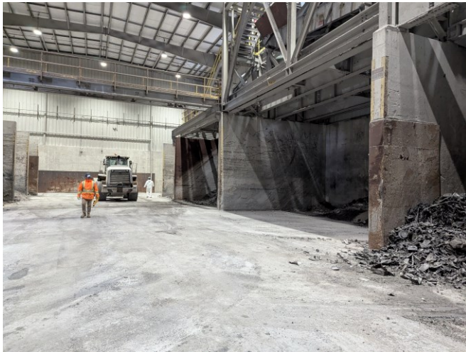
Photo 37: View of loader in the Residue Building.
