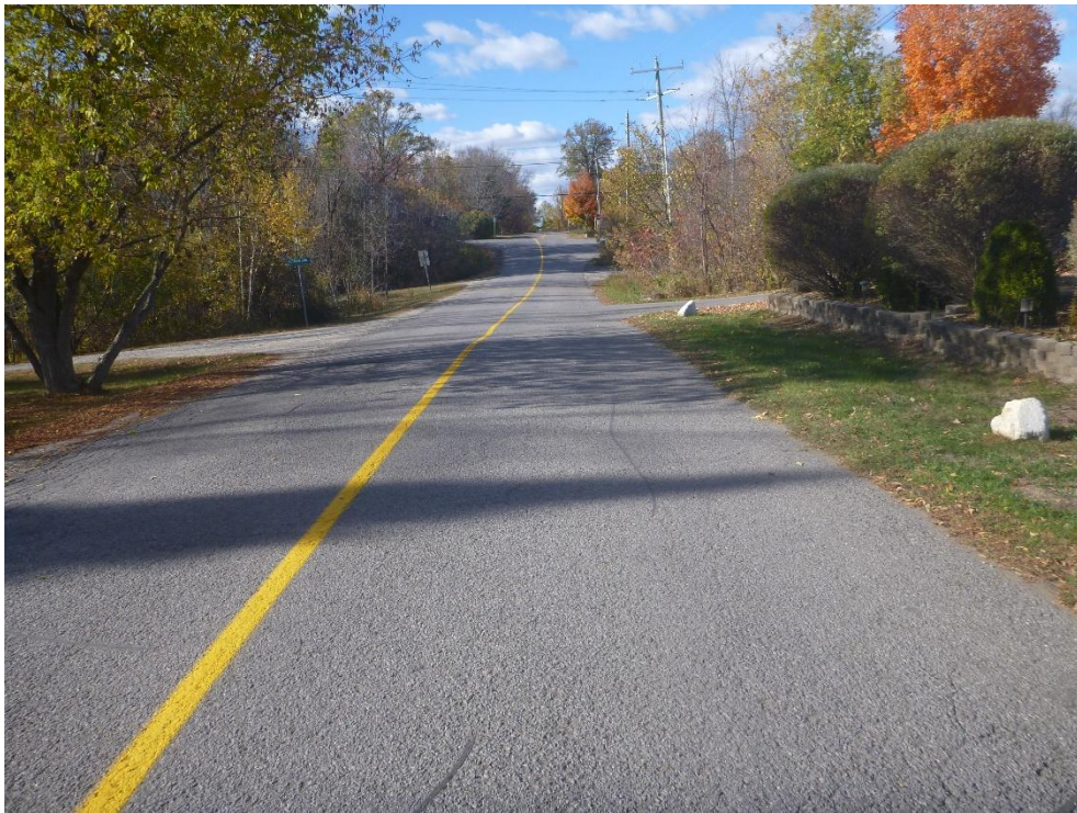
Photo 6: Looking north at roadway over the cross culvert located on Francis Street, approximately 56 m south of Mill Street
