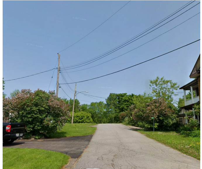
Figure 26 Existing condition of Blake Road
