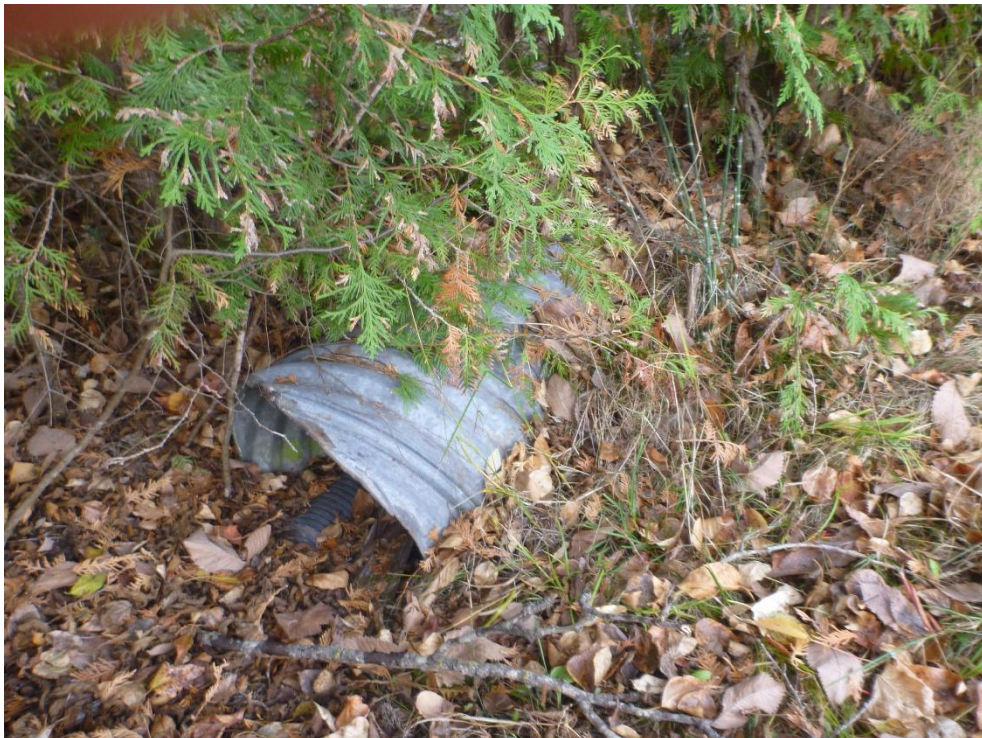
Photo 16: Cross culvert located on the Maple Street, approximately 140 m north of Calabogie Road
