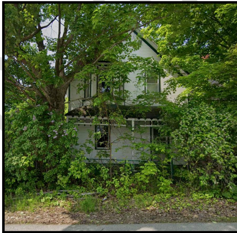
Figure 74. 21 Mowat St. Google Streetview, June 2025.
