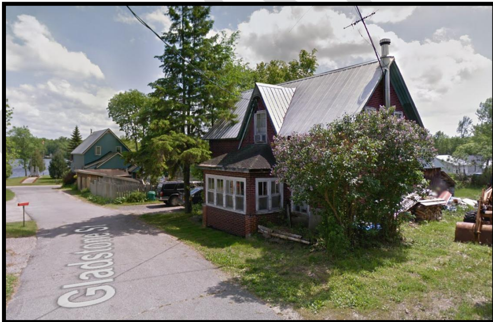
Figure 20. 513 Gladstone St. Google Streetview, May 2012.
