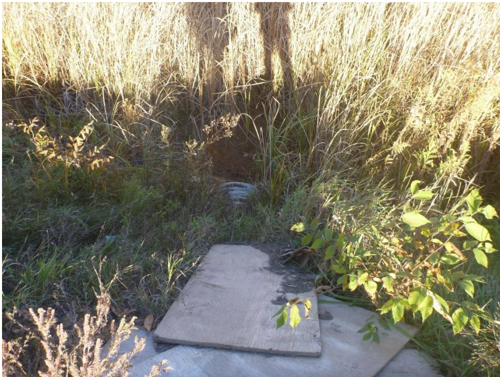
Photo 18: Looking west through the cross culvert located on Mill street, approximately 25 m south of Calabogie Road
