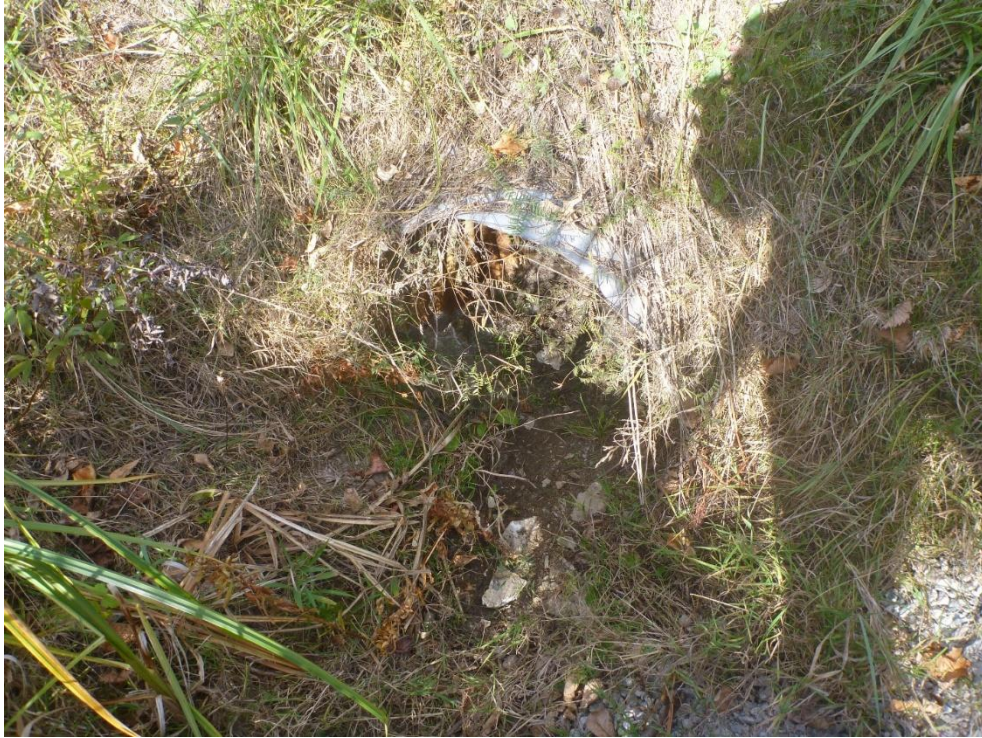
Photo 7: Looking west at the cross culvert located on Francis Street, approximately 56 m south of Mill Street
