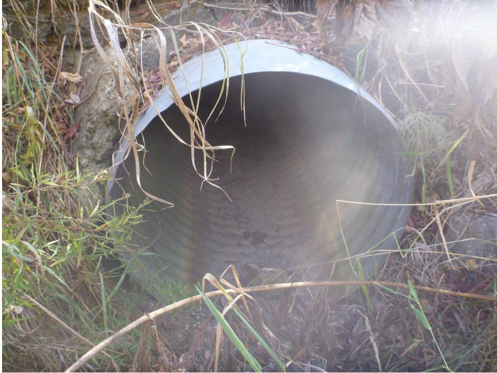
Photo 5: South elevation- Cross culvert located on Mill street, approximately 165 m east of Francis Street
