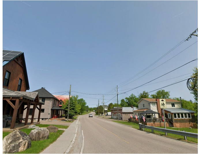
Figure 23 Existing condition of Calabogie Road/Highway 508
