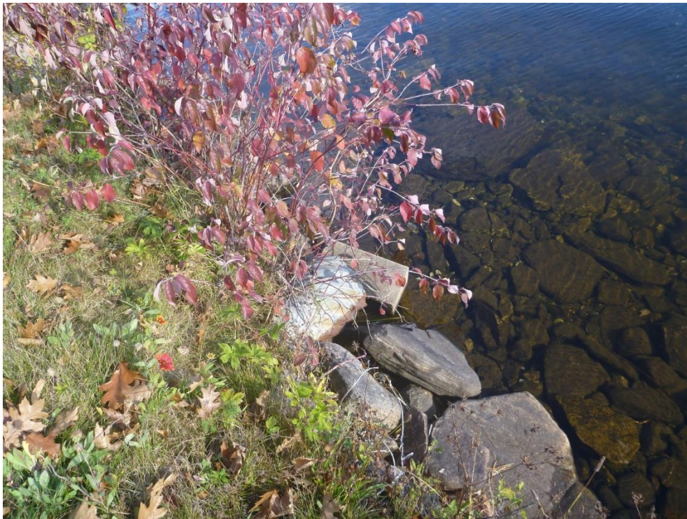
Photo 12: Outlet pipe, located on Gladstone street approximately 400 m west of Lanark Road, dischrjing stormwater south to the Madawaska River
