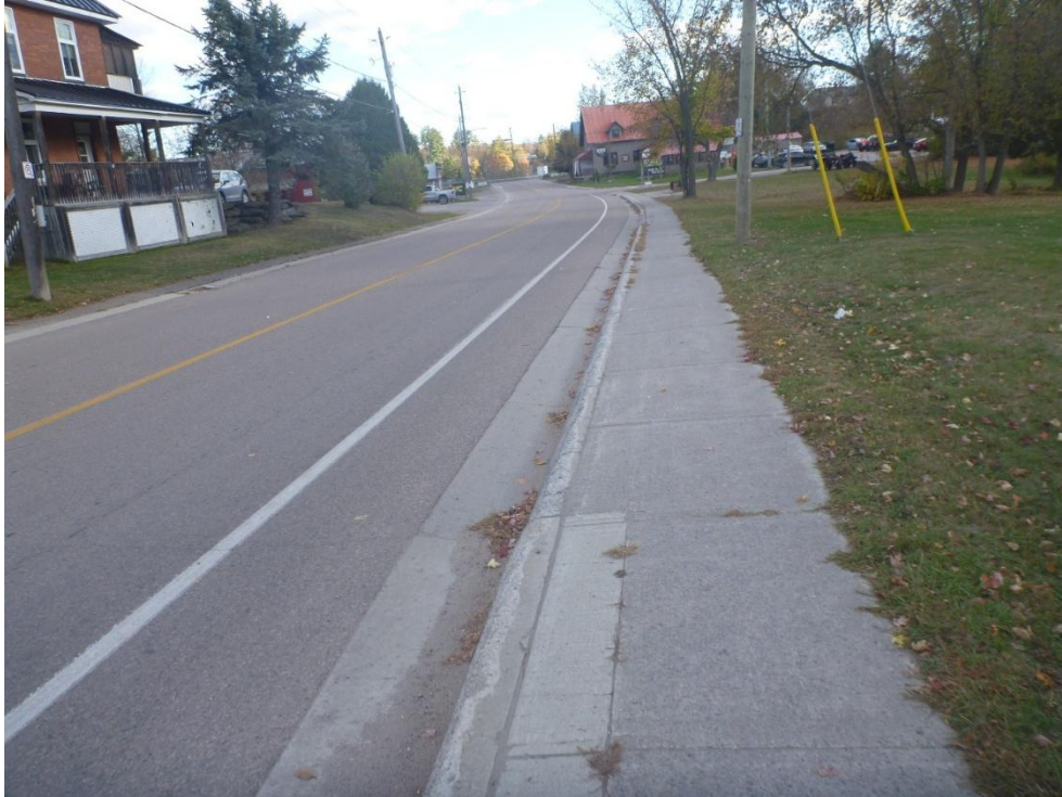
Photo 13: Looking south at Lanark Road, approximately 45 m south of Mill Street
