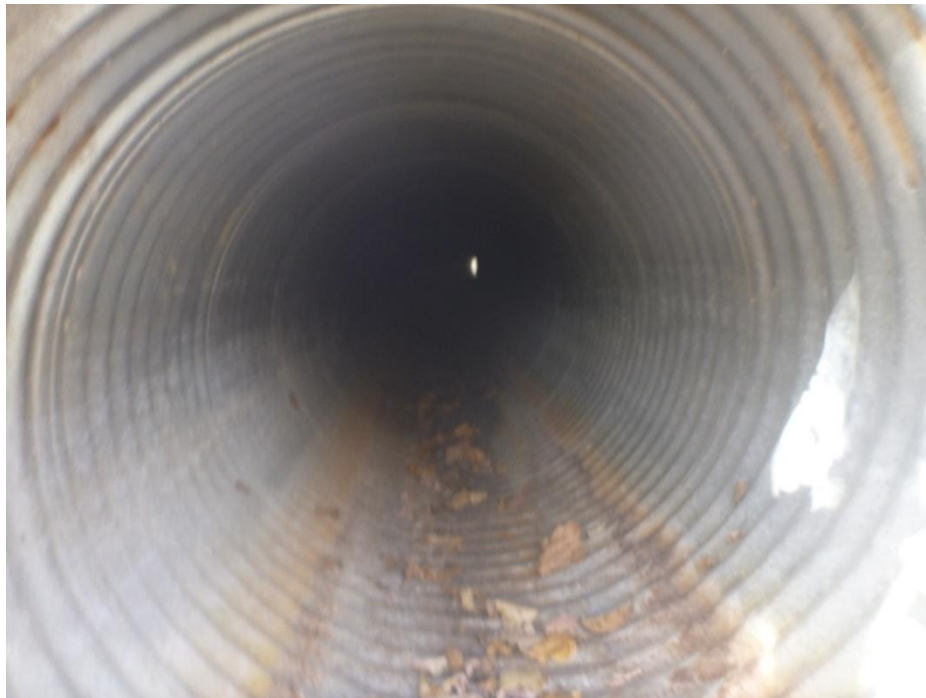
Photo 4: Looking south through barrel from end- Cross culvert located on Mill street, approximately 165 m east of Francis Street
