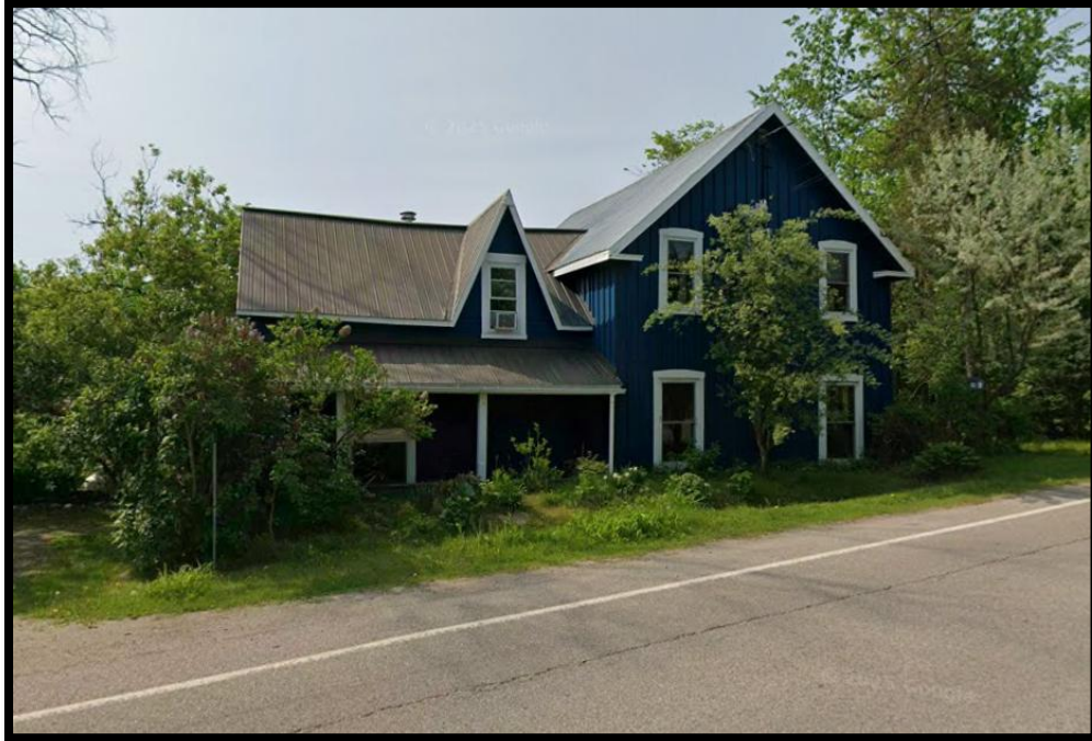
Figure 71. Old train station, 12676 Lanark Road. Google Streetview, June 2025.
