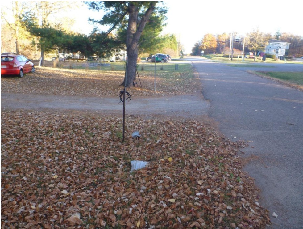
Photo 8: Looking west at the cross culvert located on Francis Street, approximately 100 m north of Calabogie Road
