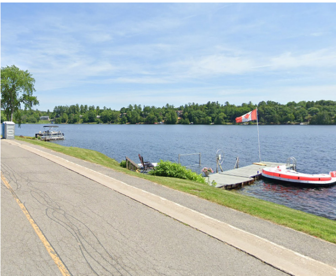
Figure 28 Existing condition of private docks along the waterfront
