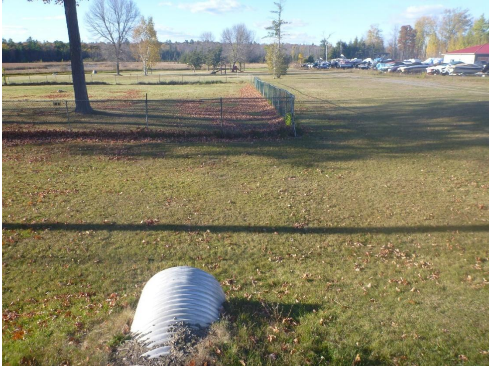
Photo 17: Looking north through the cross culvert located on Calabogie Road, approximately 80 m east of Mill Street
