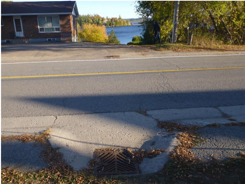
Photo 3: Catchbasins, located on Mill Street, approximately 367 m west of Francis Street, southly conveying stormwater to the Madawaska River
