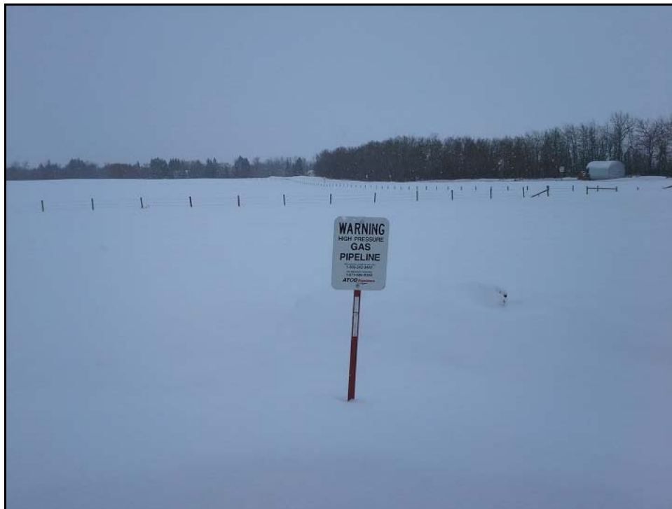
Photograph 4: Standing near the acreage roadway and facing southwest showing a sign for the Atco Gas pipeline located on the western portion (March 26, 2014).
