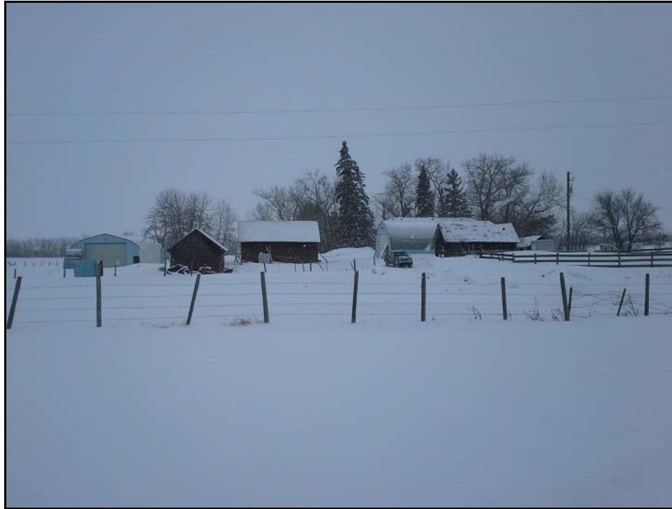
Photograph 3: Looking west showing the fenced acreage including barns and sheds (March 26, 2014).
