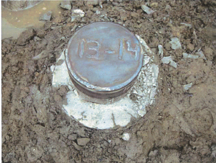
Capped wellbore casings using Lionhead's triple security system
