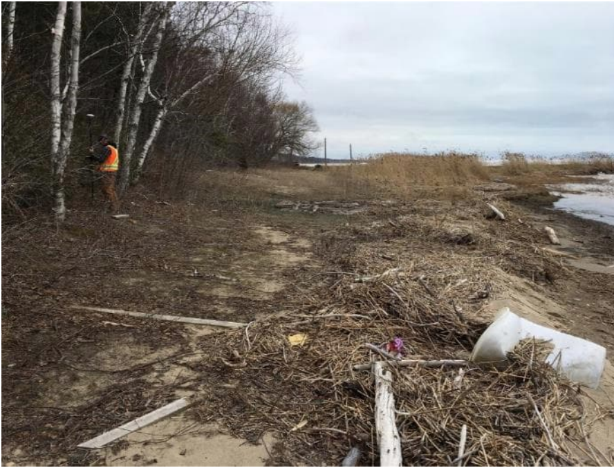
Photograph 2a: Section A-A' at beach looking south. No toe erosion on April 18, 2018.
