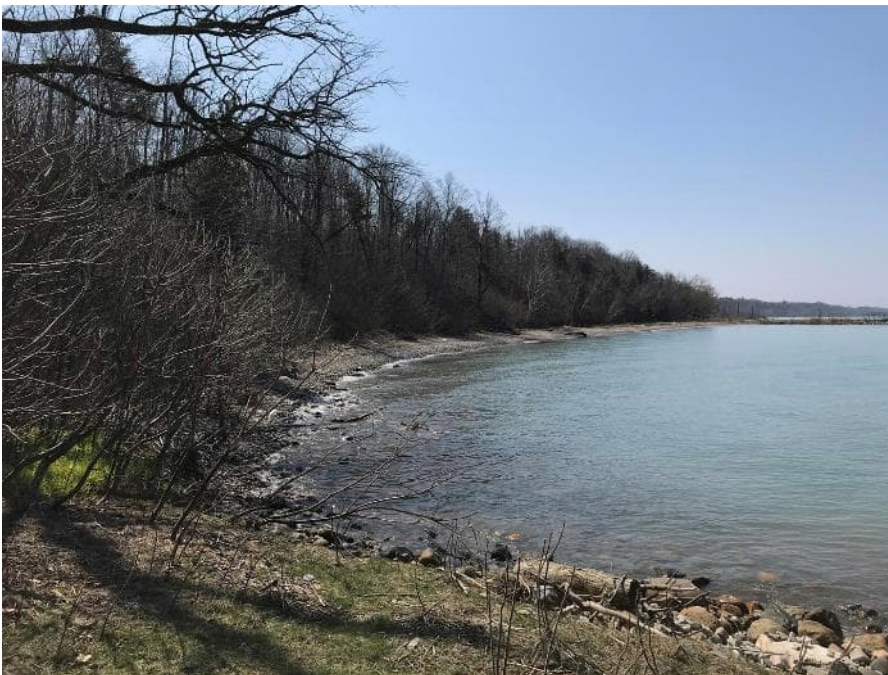
Photograph 8b: Section B-B' at toe looking south on April 8, 2020. Note higher Lake Huron water level on April 8, 2020, compared to April 18, 2020, however, no erosion at the slope toe was observed.
