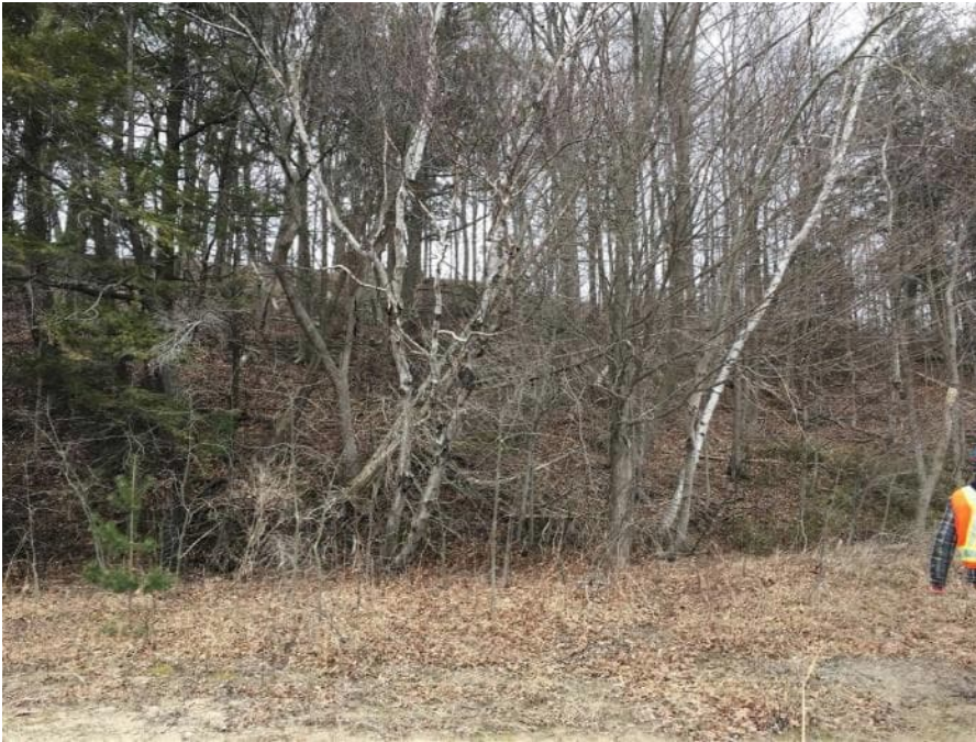
Photograph 1a: Lakeshore slope south of Section A-A'. No toe erosion on April 18, 2018.
