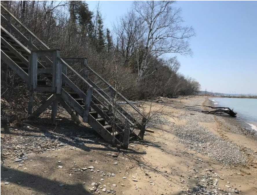
Photograph 15: Wooden staircase between Section A-A' and Section B-B' looking south. No erosion noted on April 8, 2020.
