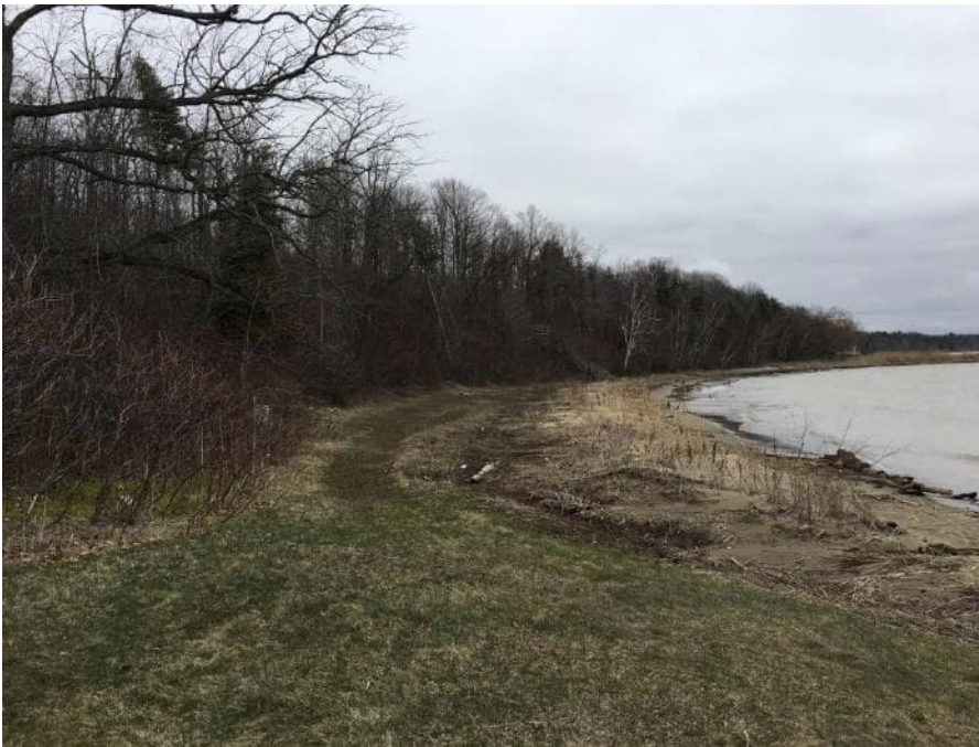
Photograph 8a: Section B-B' at toe looking south on April 18, 2018.
