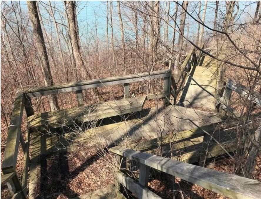
Photograph 21: Wooden staircase from top of slope looking west on April 8, 2020. Staircase in good condition.
