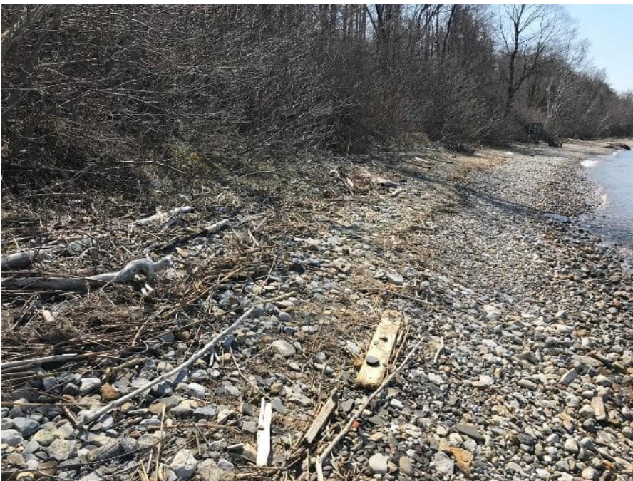
Photograph 14: Section B-B' at beach looking south on April 8, 2020. No erosion at toe of slope; however, evidence of higher Lake Huron water levels close to the toe of slope.
