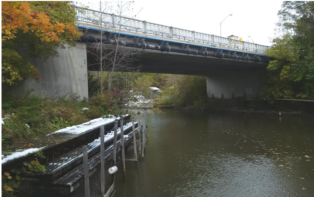
View of Highway 21 Bridge looking downstream (west)
