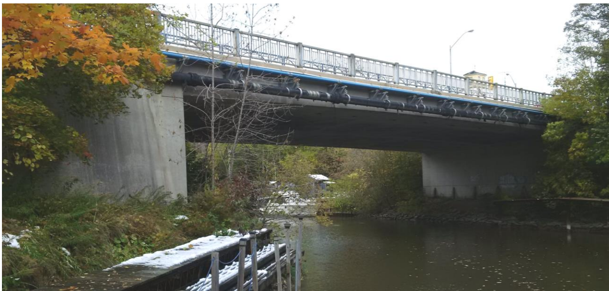
View of Ontario Street bridge looking northwest (downstream)
