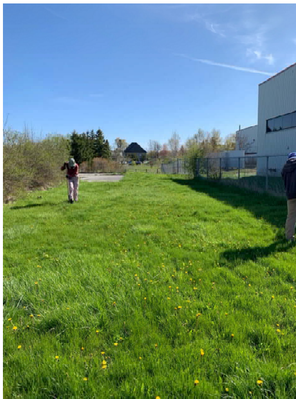
Image 25: Test pitting disturbed area behind building at 10 metre intervals (view facing North).
