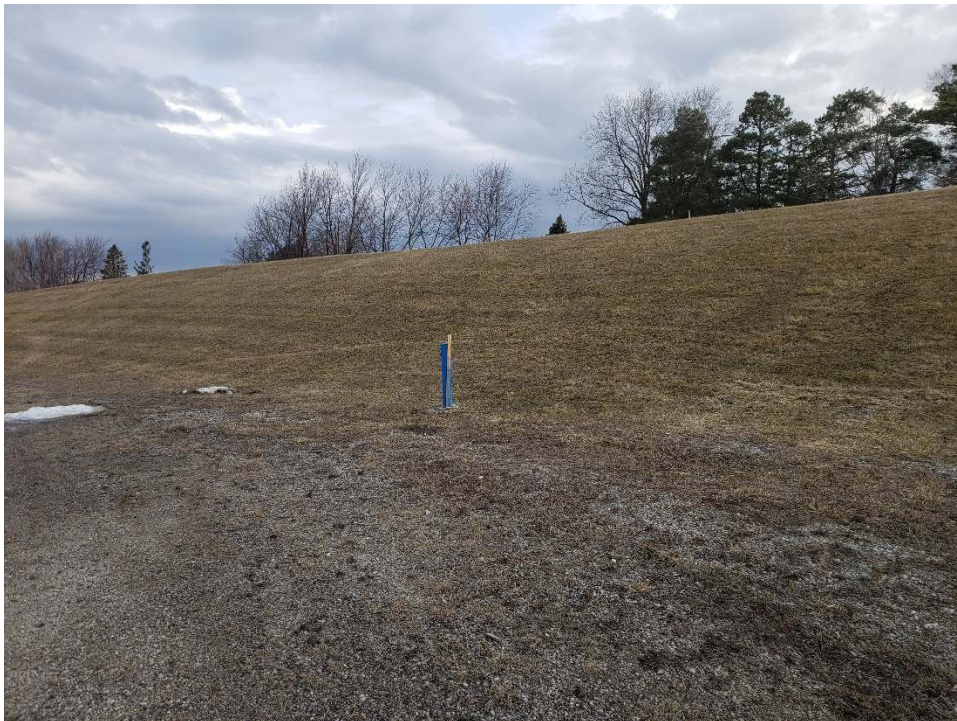
Image 8: Heavily sloped area at the east of the building (View facing North).
