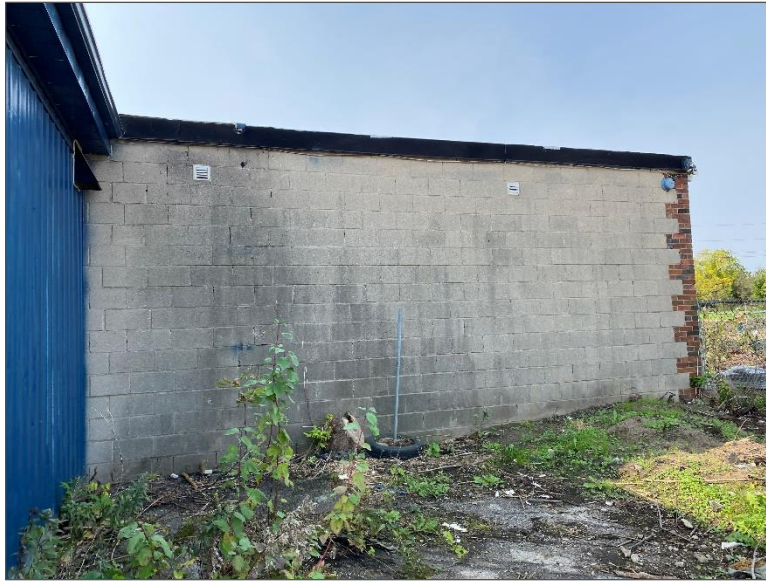
Photo 3 – Site Building (portion of the northeast elevation).
