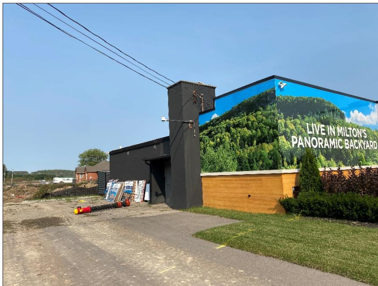
Photo 4 – Site Building (southwest elevation).
