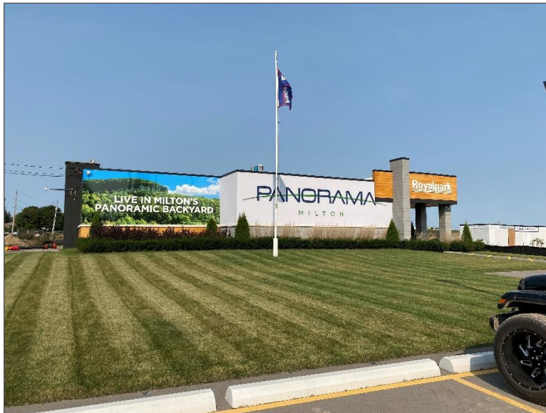
Photo 2 – Site Building (southeast elevation).
