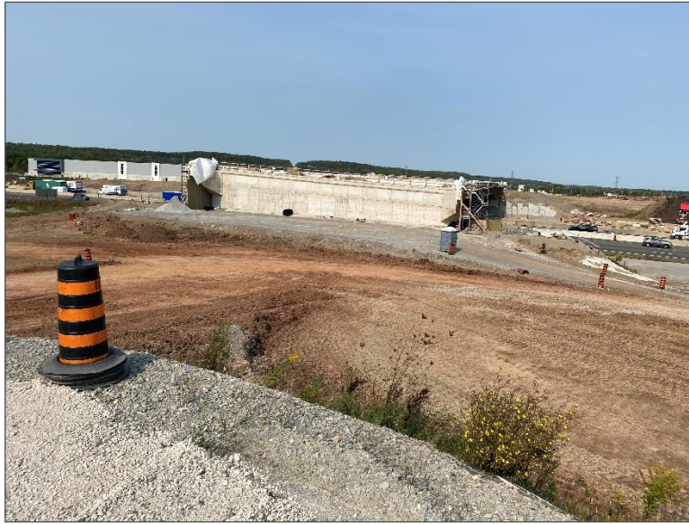
Photo 11 – View of the north portion of the Site facing northwest.
