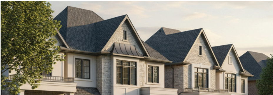
Example of traditional roof form
