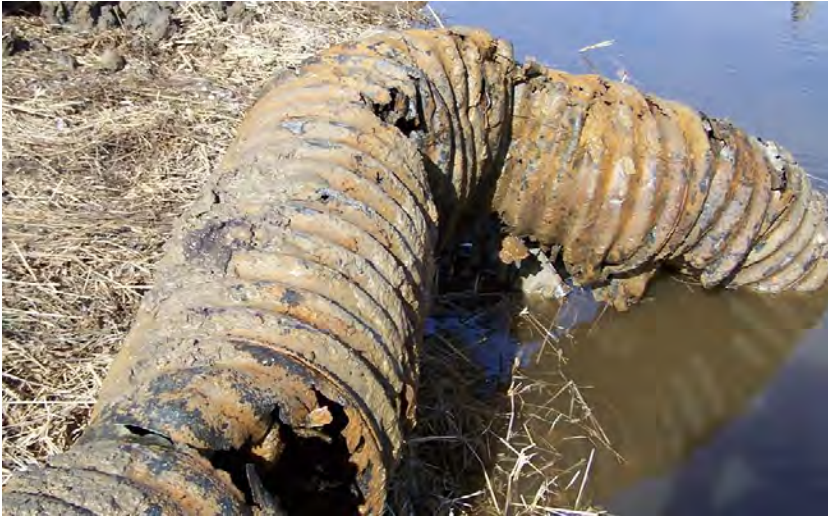
Damaged culvert
