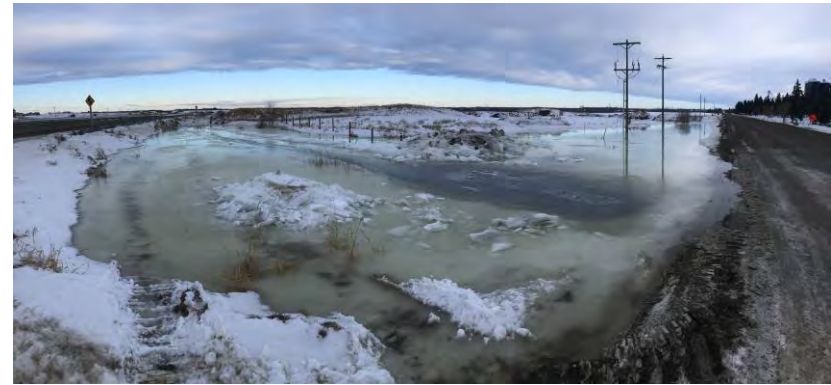
Spring runoff encroaching roadway.
