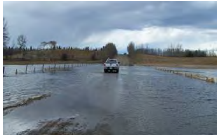
Runoff overtopping Township Road 514 in April 2013
