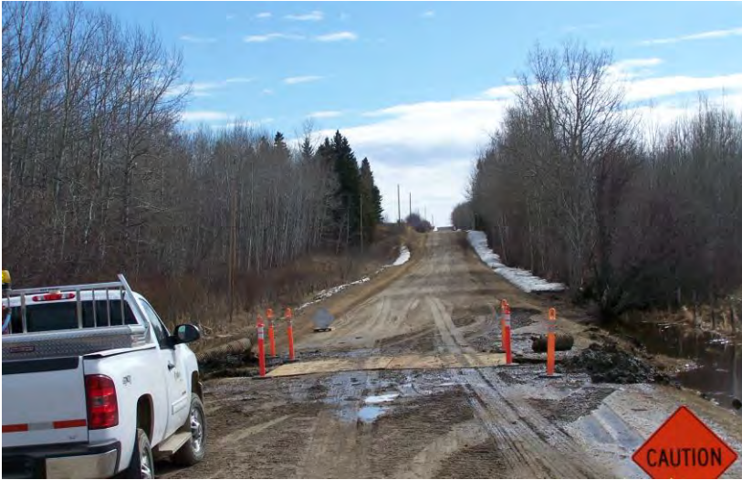
Roadways Maintenance and Drainage crew repairing washed out culvert
