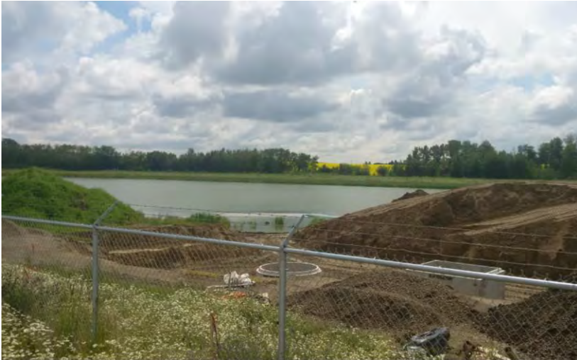
Construction of Stormwater Control Structure
