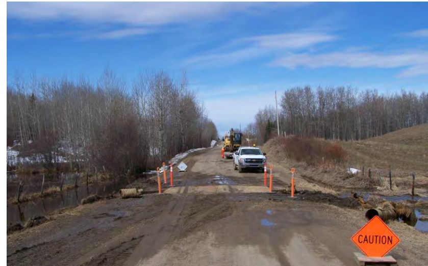
Township Road 514 Culvert Replacement
