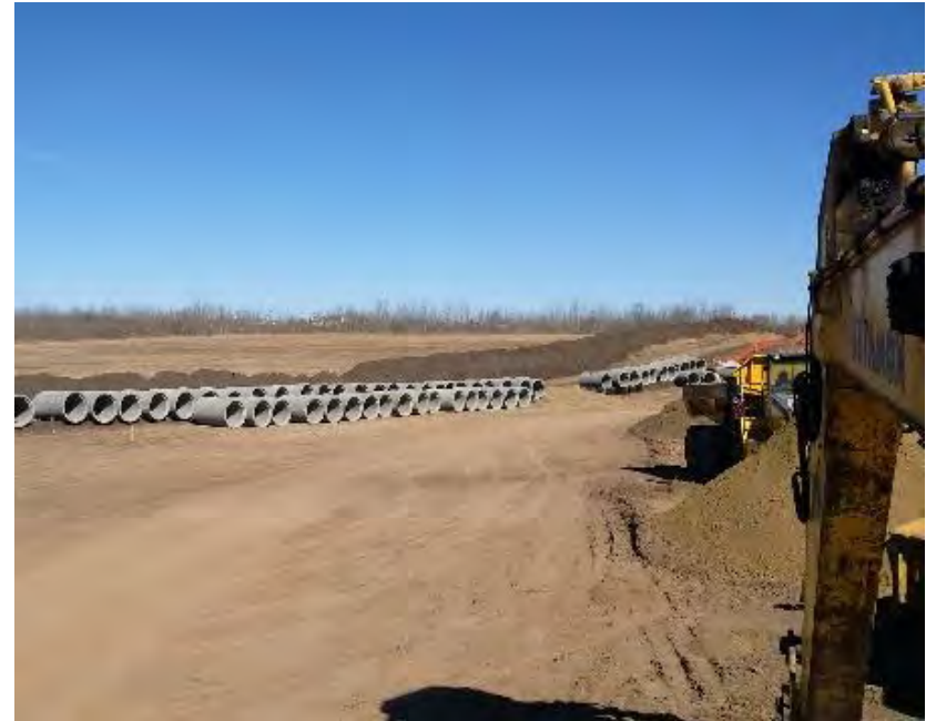
Acheson Basin 1 Storm Trunk Installation
