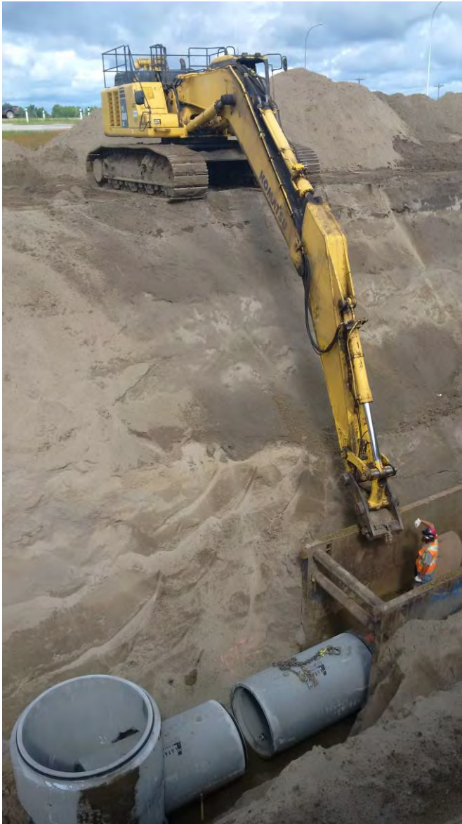
Acheson Basin 1 Storm Trunk Installation
