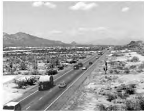
Level of Service "B"
