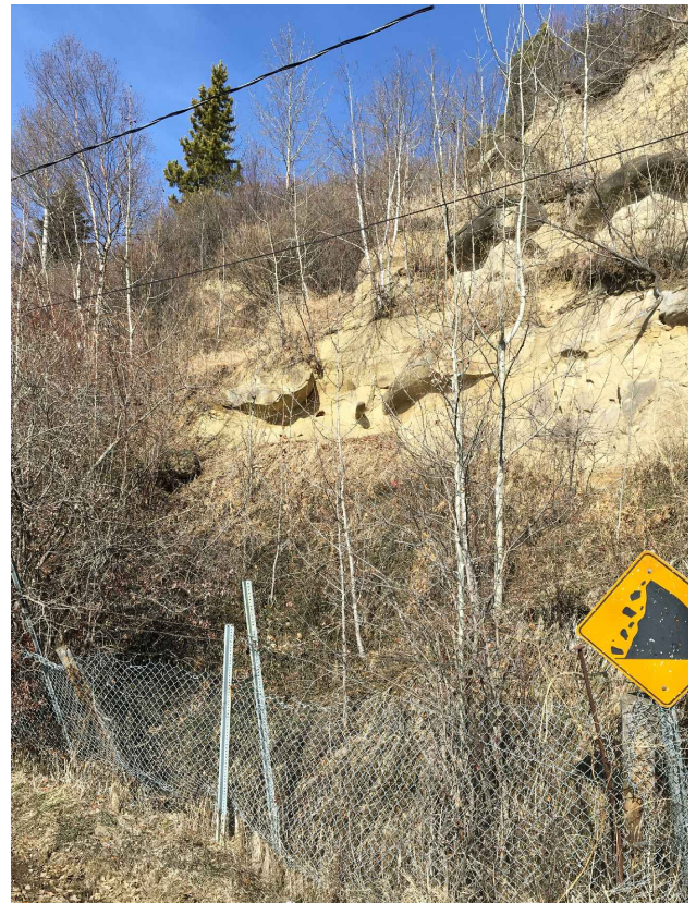
PHOTO 5 - VIEW OF FENCE LOCATED ALONG FIRST AVENUE. FENCE LOCATION MARKED ON DRAWING 21720-1B.
