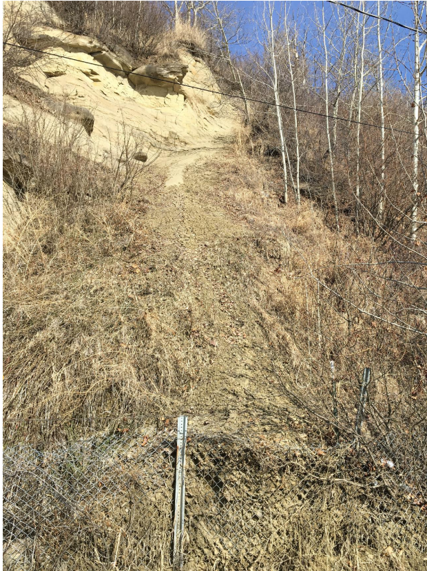
PHOTO 6 - VIEW OF ACCUMULATED SAND AT FENCE
