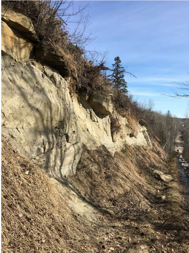
PHOTO 4 - VIEW OF SANDSTONE OUTCROP ALONG ABANDONED COUNTY ROADWAY
