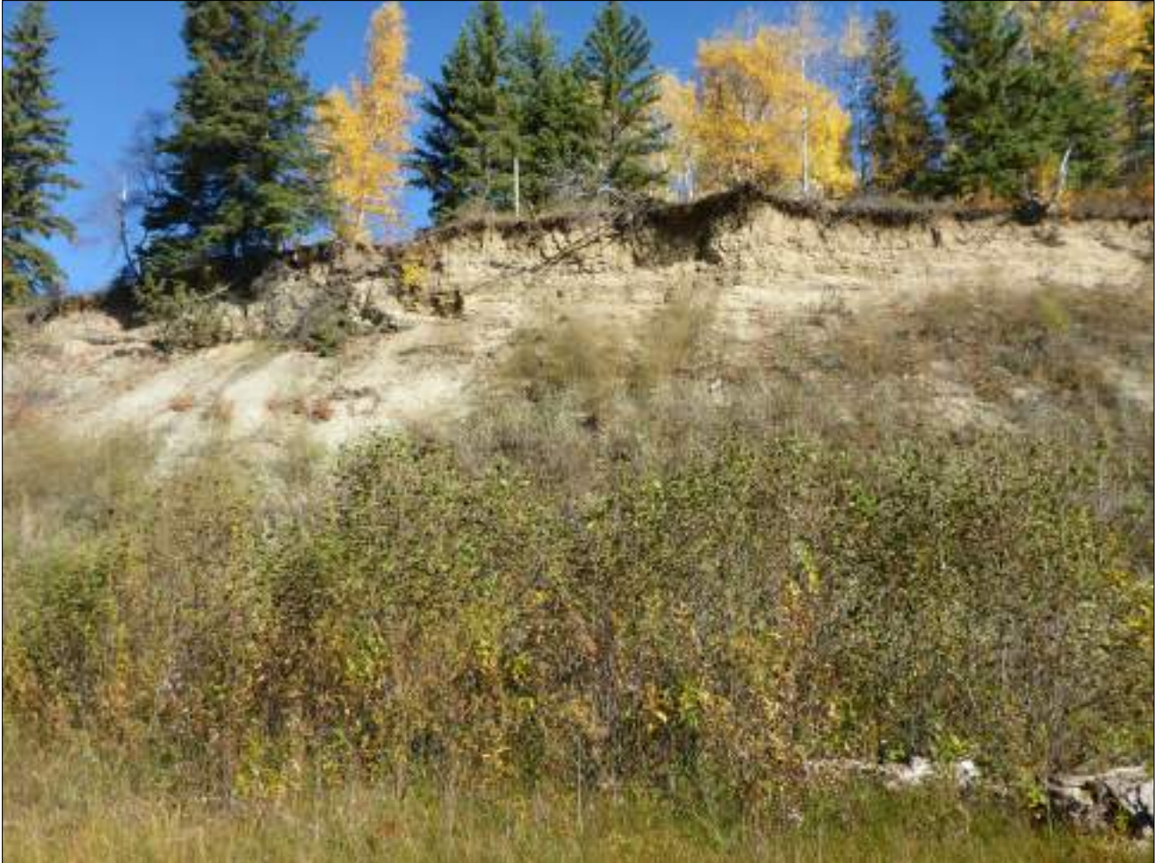
PHOTO 12 SITE 2 - OVERALL VALLEY SLOPE - NORTH
