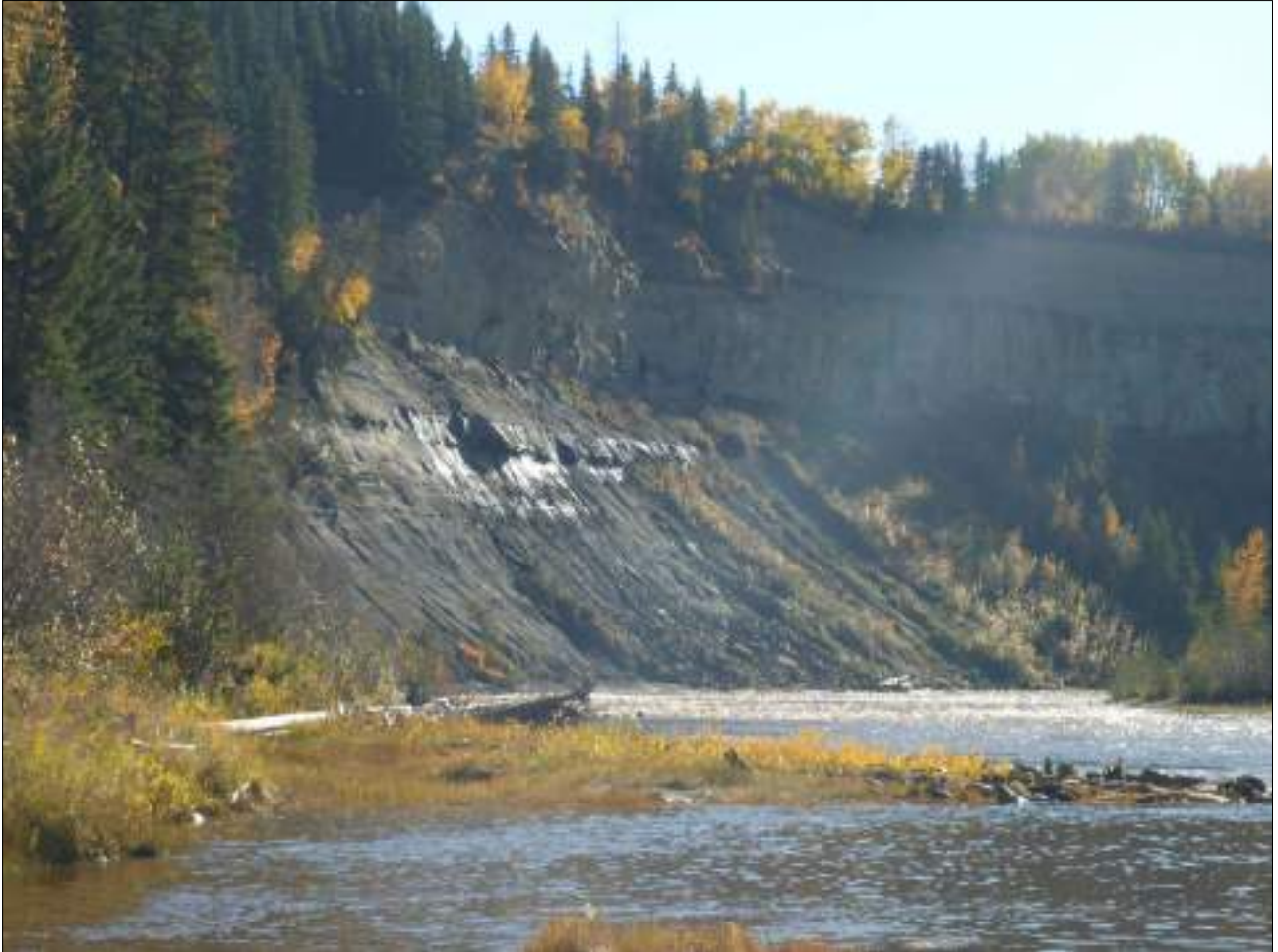
PHOTO 10 SITE 2 - MIDSLOPE SEEPAGE AND COLLUVIUM SLOPE
