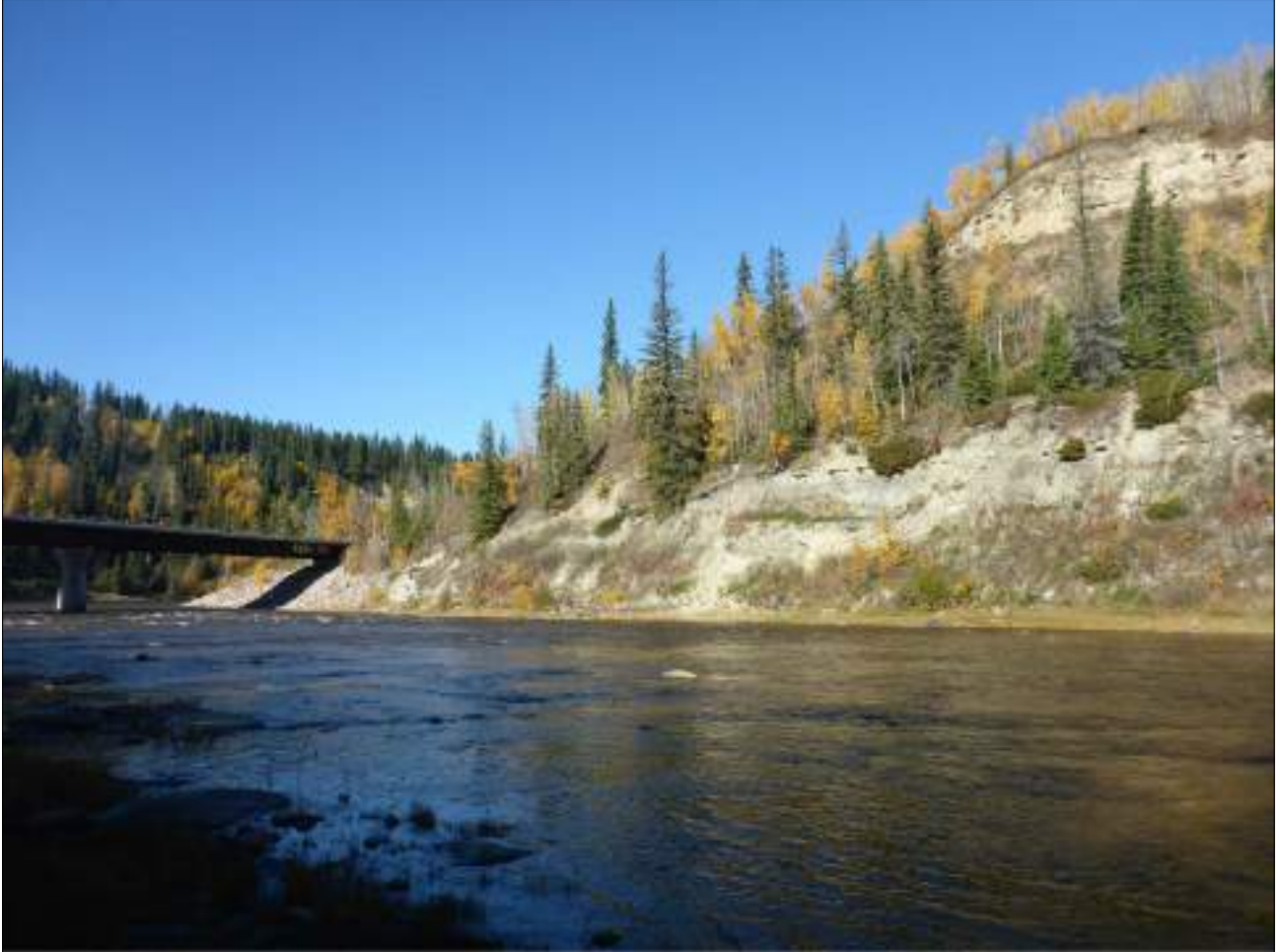
PHOTO 26 SITE 4 - OVERALL VALLEY SLOPE - NORTH
