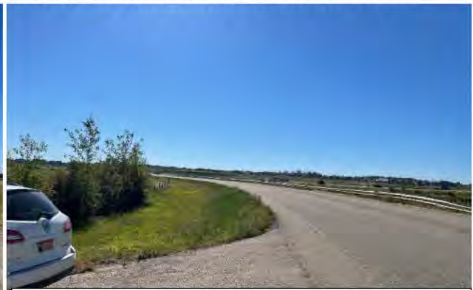
Viewing to the south onto Twp. Rd. 532A from the proposed RV Storage Site Access approach.
