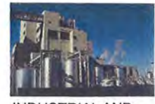
INDUSTRIAL AND WASTE TREATMENT
