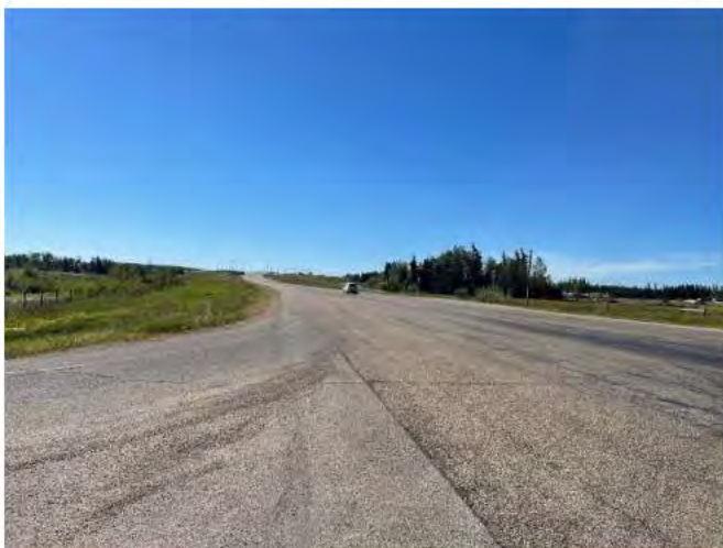
Viewing to the south from the Twp. Rd. 532A East approach.
