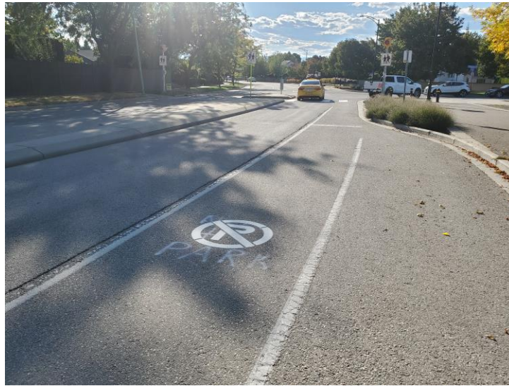
Figure 27. No Parking symbols installed in the bike lane on Casorso Rd
