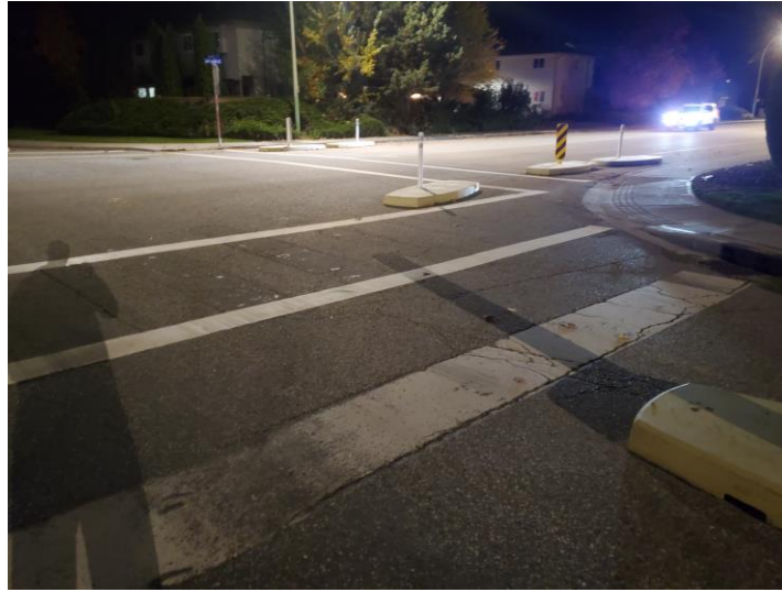
Figure 29. Parallel bar crosswalks were installed at the Lanfranco Rd
