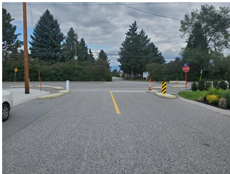
Figure 28. Traffic calming curbs, stop bar and centerline on the Bechard Rd.
