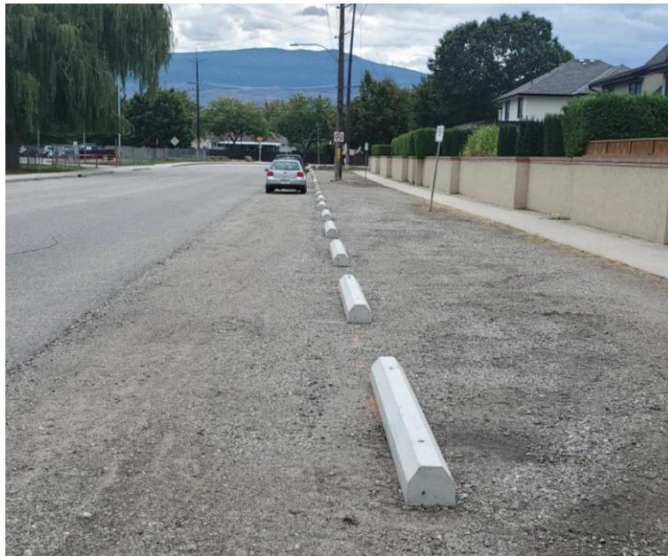
Figure 25. Parking curbs were installed on Casorso Road
