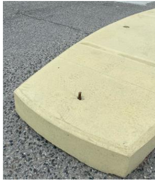
Figure 32. Photo of rebar to be trimmed down
