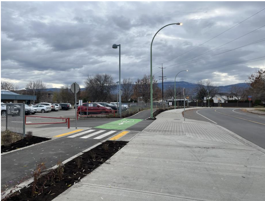
Figure 34. Casorso ATC fronting Casorso Elementary School access.
