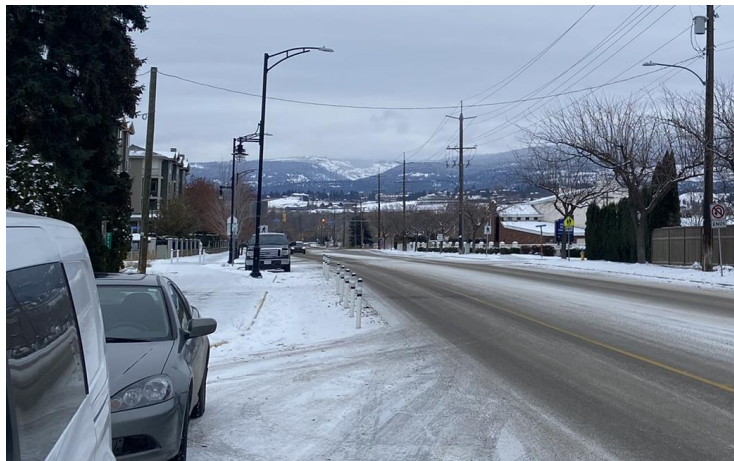
Figure 33. Delineator posts adjacent to the bike lane
