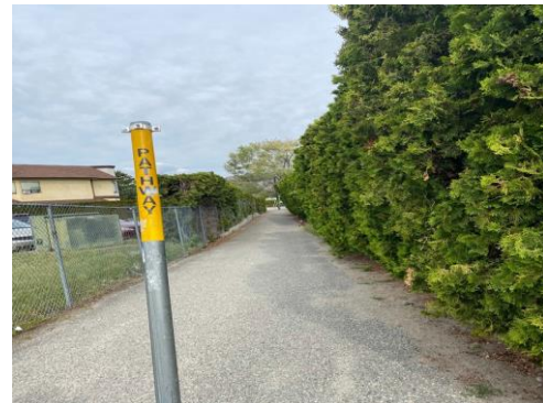
Figure 30. Overgrown bushes on Walkway
