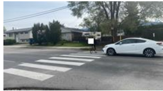
Figure 26. Cars stop too close to crosswalk
