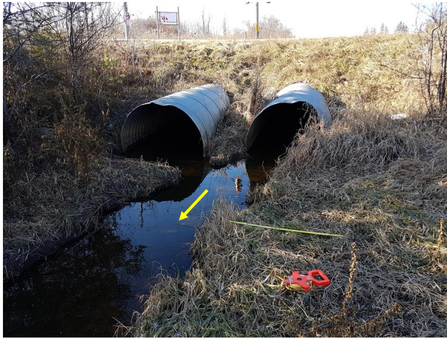
Speedville Road culvert outlet.
