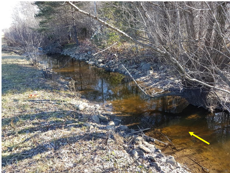
Plane bed with riverstone bank armouring along channel.
