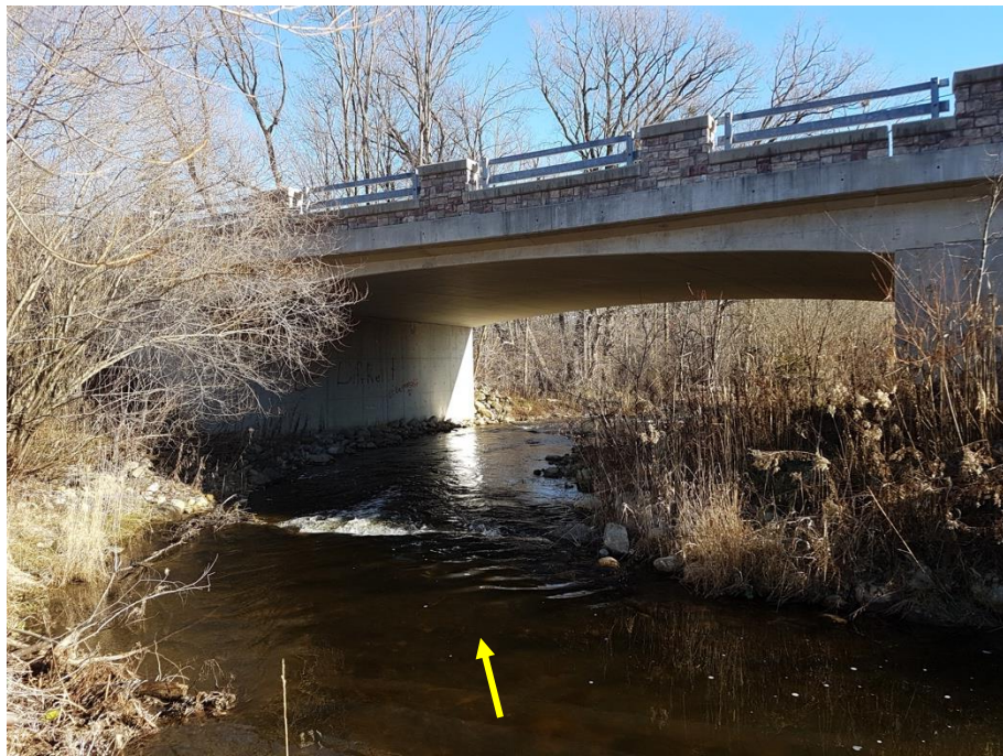
Chilligo Road bridge at the downstream end of reach. A weir is positioned just upstream of the bridge and provides upstream channel bed grade control.
