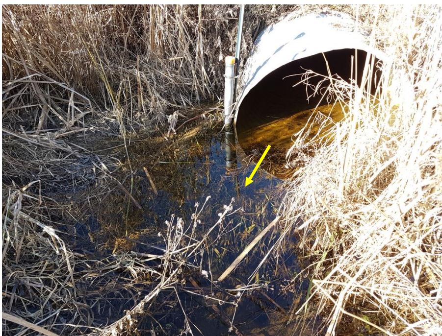
CSP culvert outlet at Maple Grove Road.
