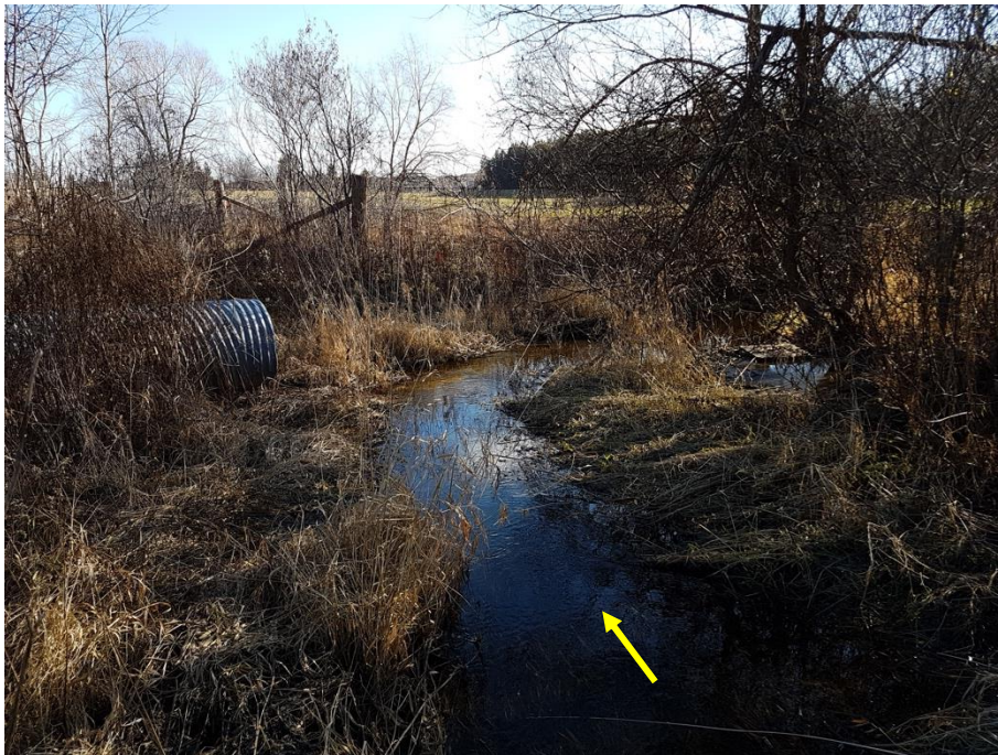
Downstream end of reach where the channel turns away from the road.
