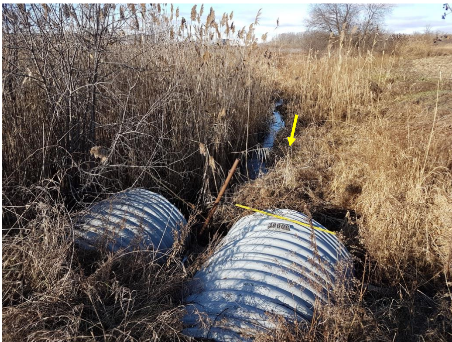
Reach viewed upstream from Maple Grove Road at downstream end of reach.
