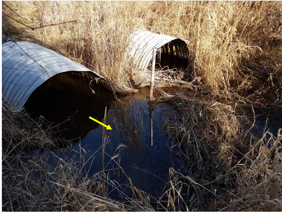
Culvert outlet at upstream end of reach at Maple Grove Road.
