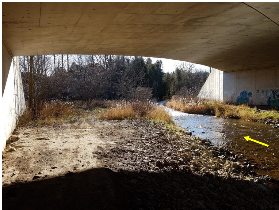
Channel and overbank area under the Maple Grove Road bridge.
