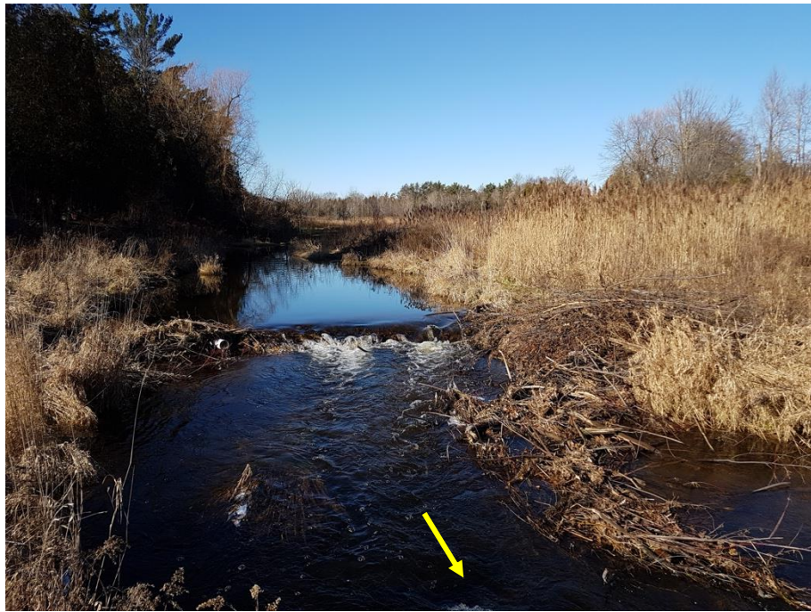
Beaver dam with overtopping flow.
