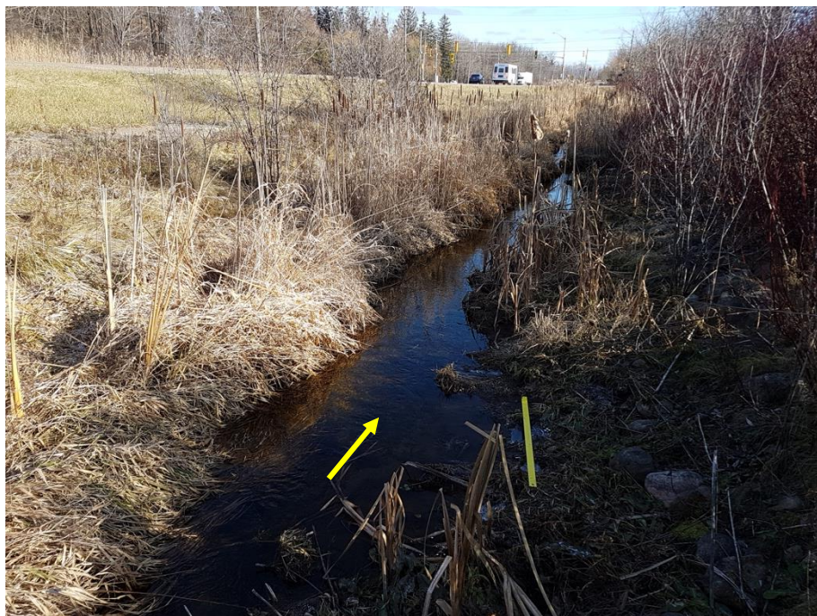
Linear channel along the south side of Maple Grove Road with some riverstone armouring along south bank. The channel along the road is also known as Hunsperger Drain.
