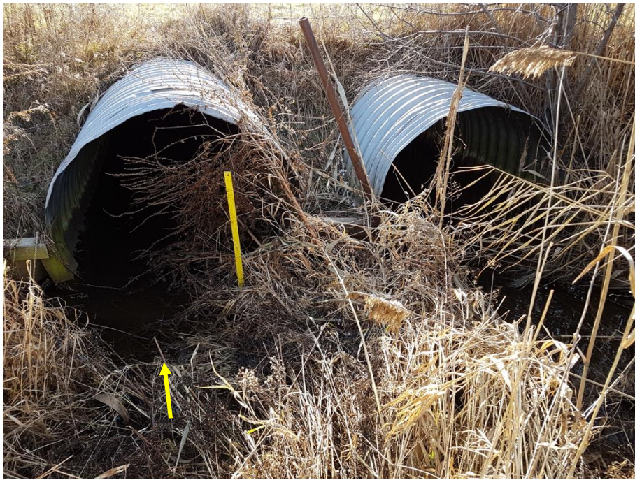
Twin corrugated steel pipe culvert inlet at Maple Grove Road. The pipes are partially embedded.
