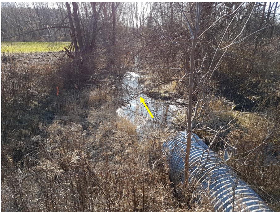
Upstream end of reach viewed downstream from Maple Grove Road. A CSP culvert conveys flow from the north side of Maple Grove Road into the reach.
