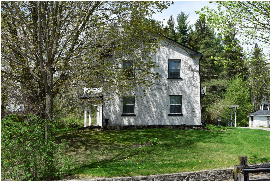
Figure 17: Gable end of 328 Main Street
