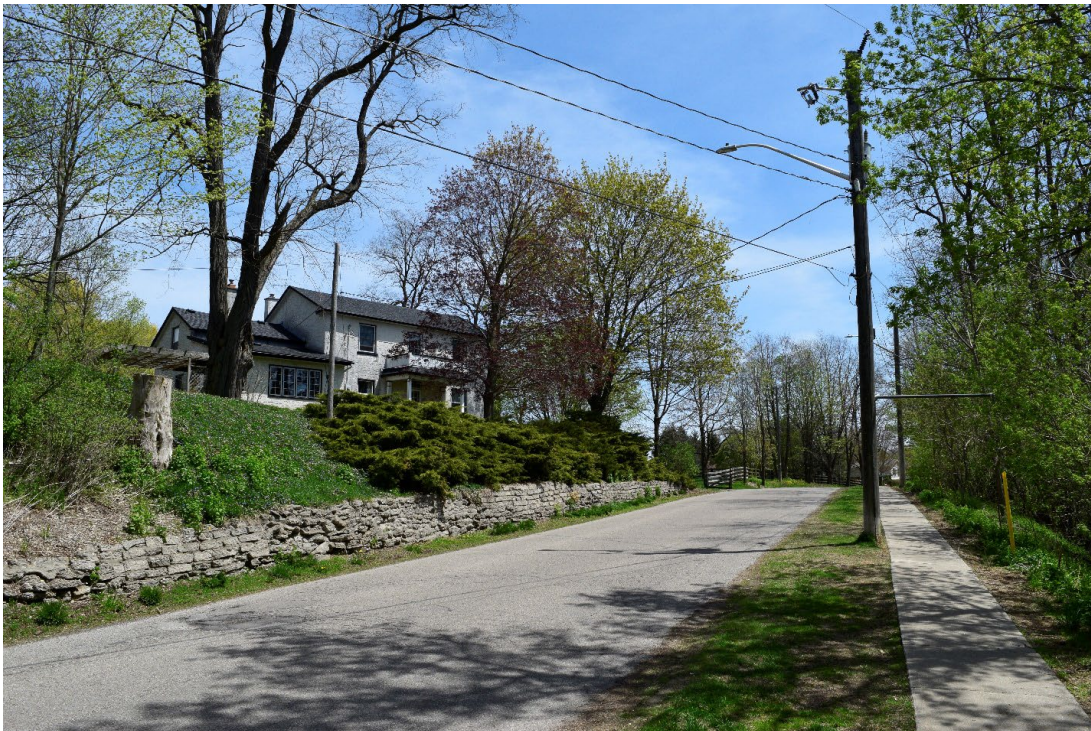
Figure 10: 328 Main Street as seen from intersection of Alderview Drive and Main Street
