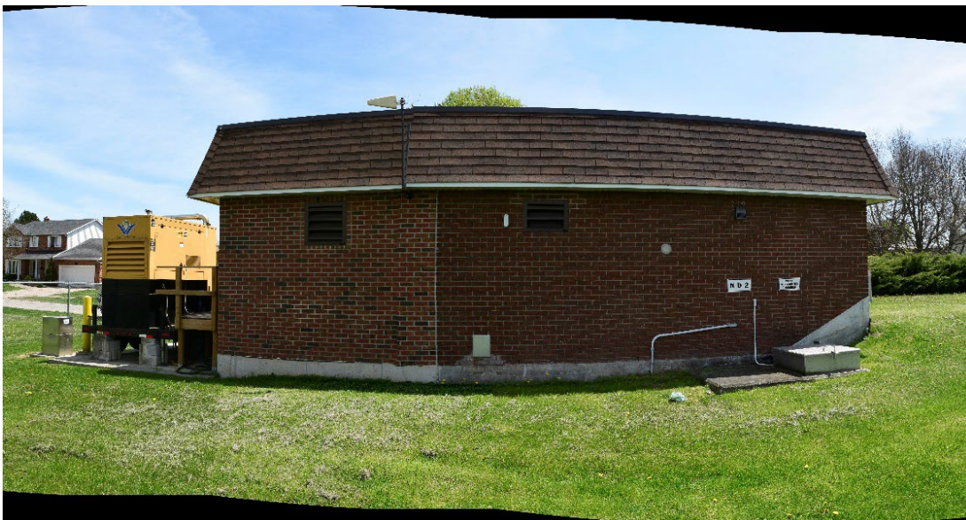
Figure 25: Rear of 156 Alderview Drive
