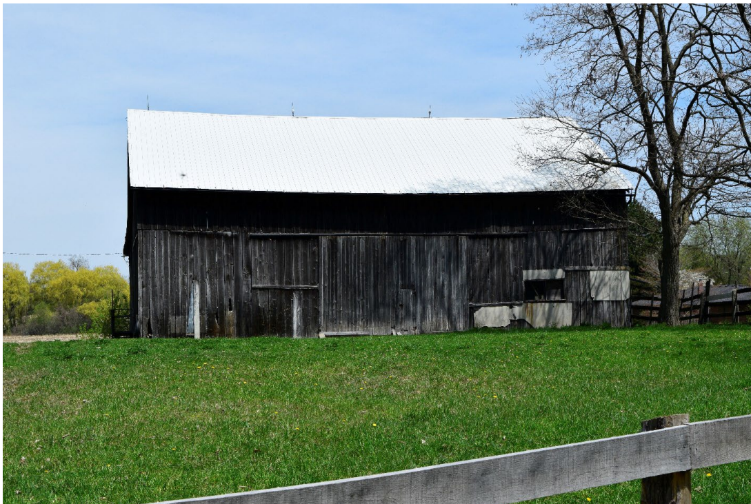
Figure 19: Main Street exposure of timber frame barn
