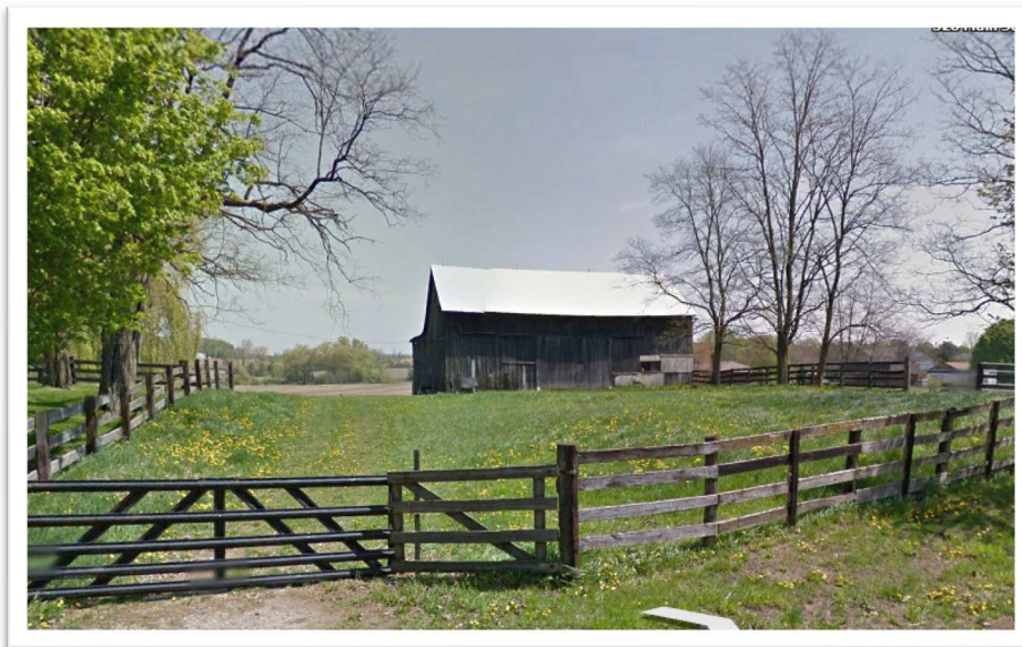
Image 7: 328 Main Street, property adjacent to (north) current New Dundee Pumping Station. Mid- to late-19th century farmstead.
