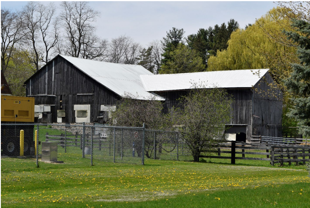
Figure 21: Northeast exposure of timber frame barn, all three segments of the structure are clearly visible, current water supply infrastructure is visible on left of image
