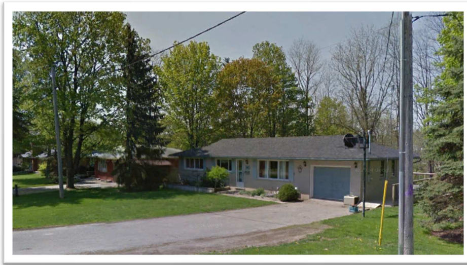
Image6: 96 Alderview Drive, property adjacent to (east) current New Dundee Pumping Station. Mid-20th century residence.
