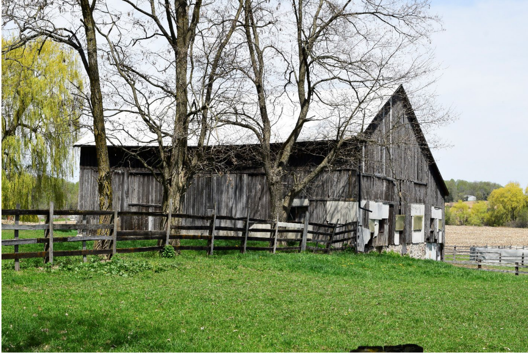
Figure 20: Southeast corner of timber frame barn, shed roof addition is visible on right of image
