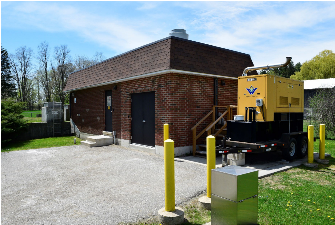
Figure 24: Existing water supply infrastructure at 156 Alderview Drive, 328 Main Street is located behind, timber frame barn is visible on right of image
