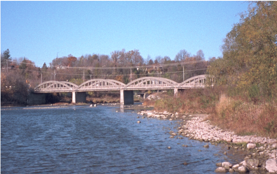
North West View
