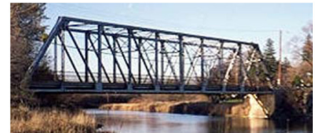
Haysville Bridge, Wilmot (Demolished)
