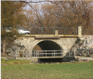
Mill Creek Bridge, Cambridge
