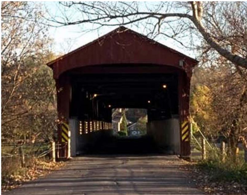
West Montrose Covered Bridge, Woolwich
