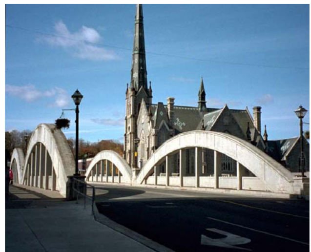
Main Street Bridge, Cambridge
