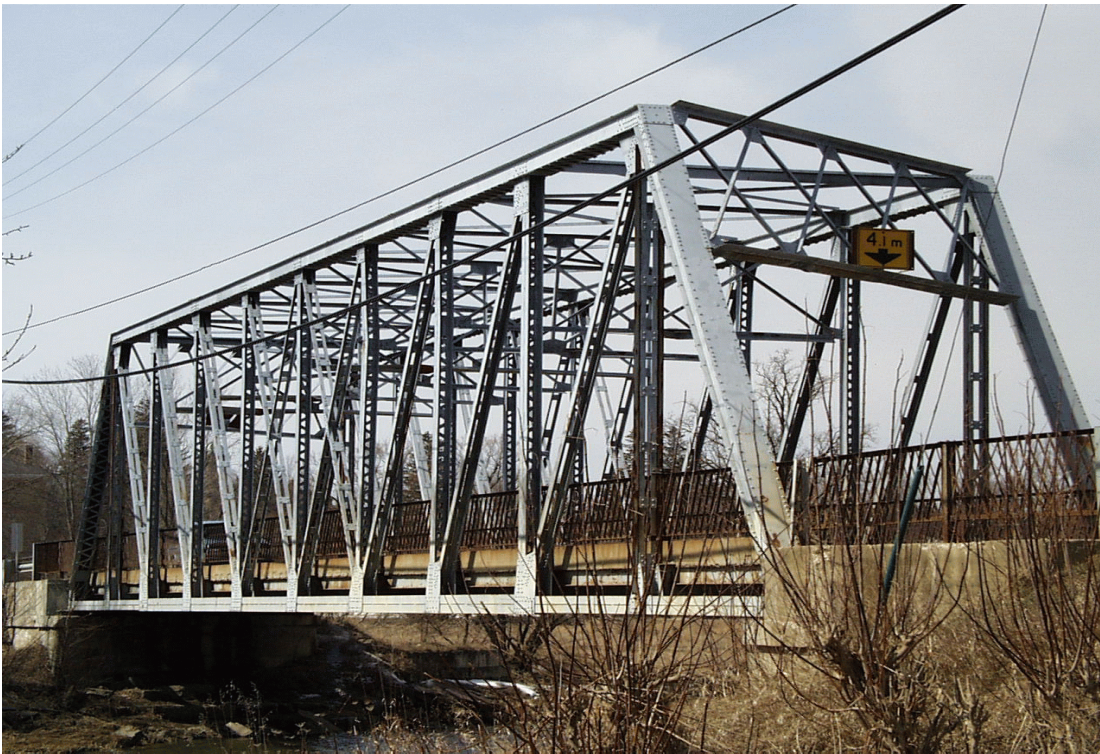
North West View
