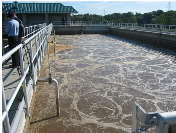
Photograph 1 ↑ New Hamburg WWTP SBR
