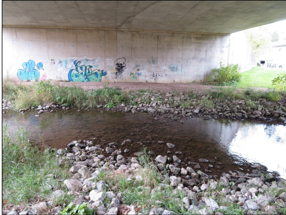
Photo P37 – Typical Condition of West Slope
