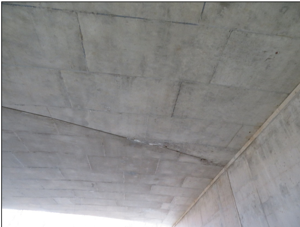
Photo P14 – Typical Condition of Soffit @ West (fair-to-good condition – wet areas and efflorescence staining at construction joint)
