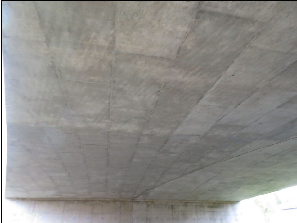
Photo P15 – Typical Condition of Soffit from East (fair-to-good condition – wet areas and efflorescence staining at construction joint)
