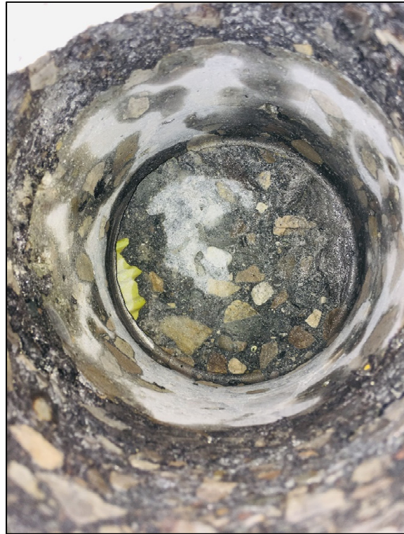
INSIDE CORE HOLE
