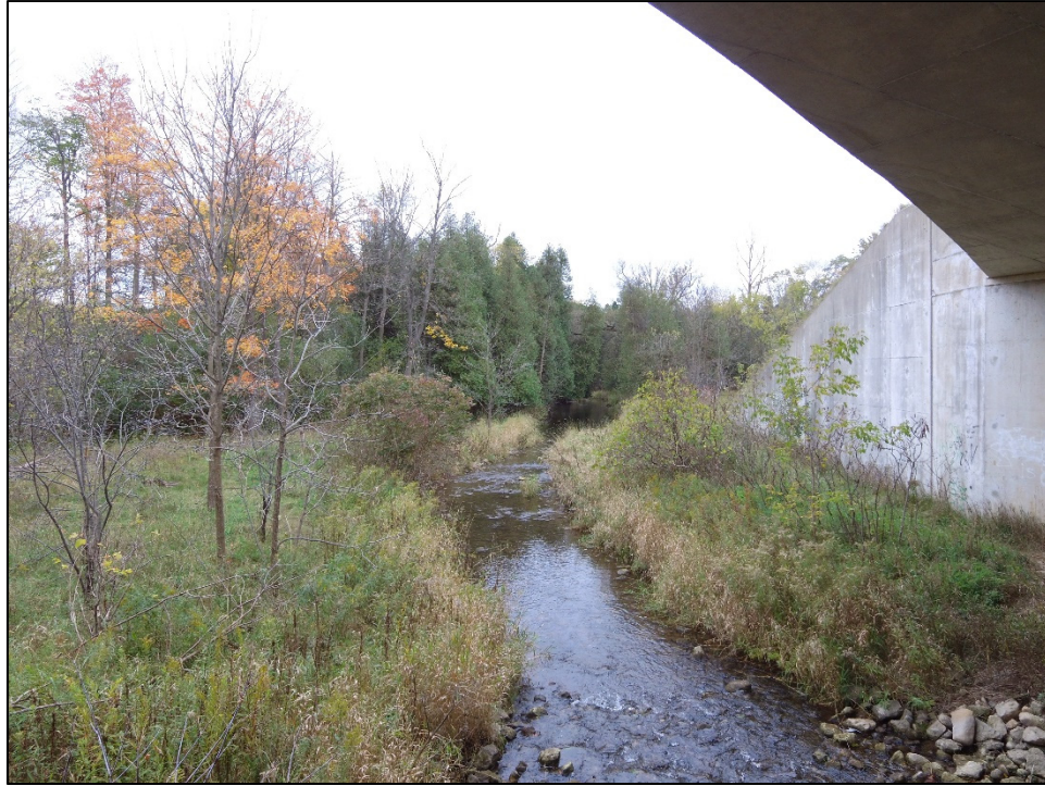
Photo P7 – General Overview Looking South (downstream)
