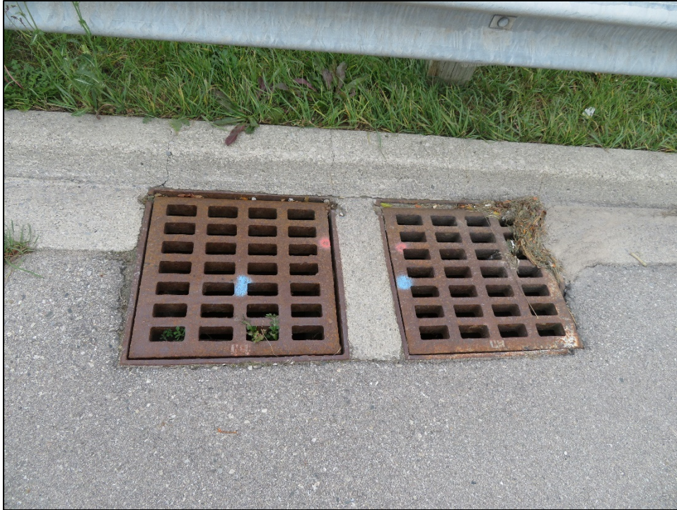
Photo P35 – Typical Condition of South-West Catchbasin
