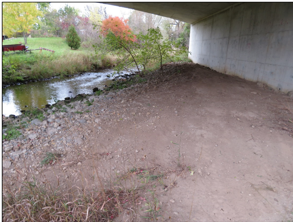
Photo P38 – Typical Condition of East Slope
