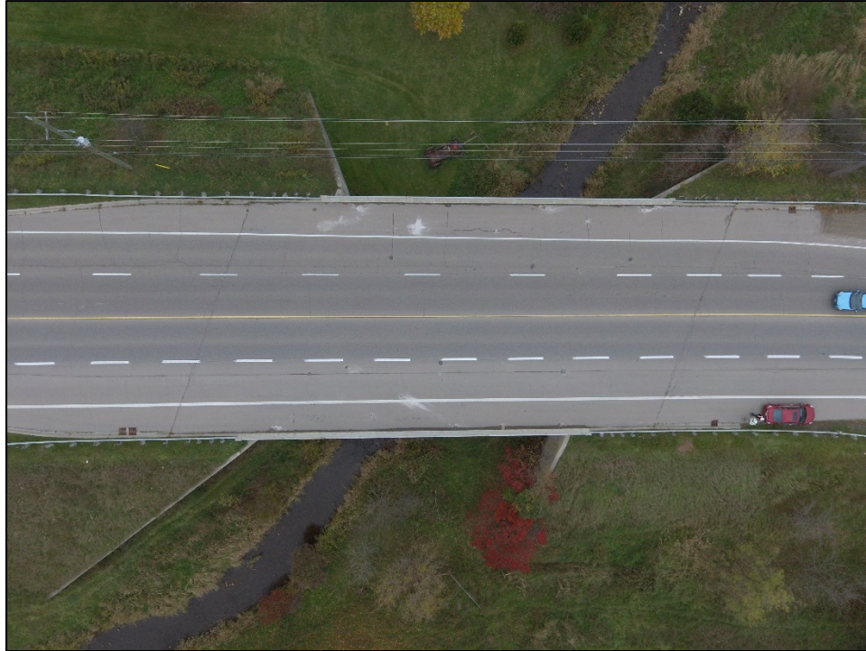
Photo P3 – Aerial Overview of Structure
