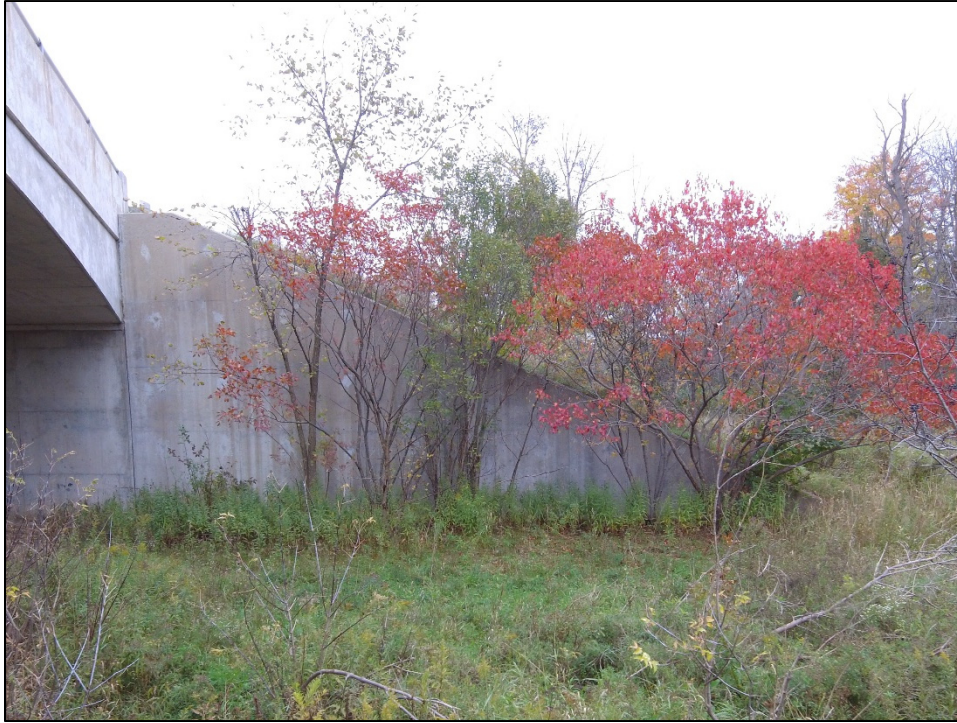
Photo P31 – Typical Condition of South-East Retaining Wall (fair condition)
