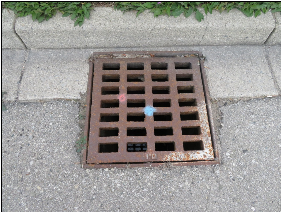
Photo P34 – Typical Condition of South-East Catchbasin
