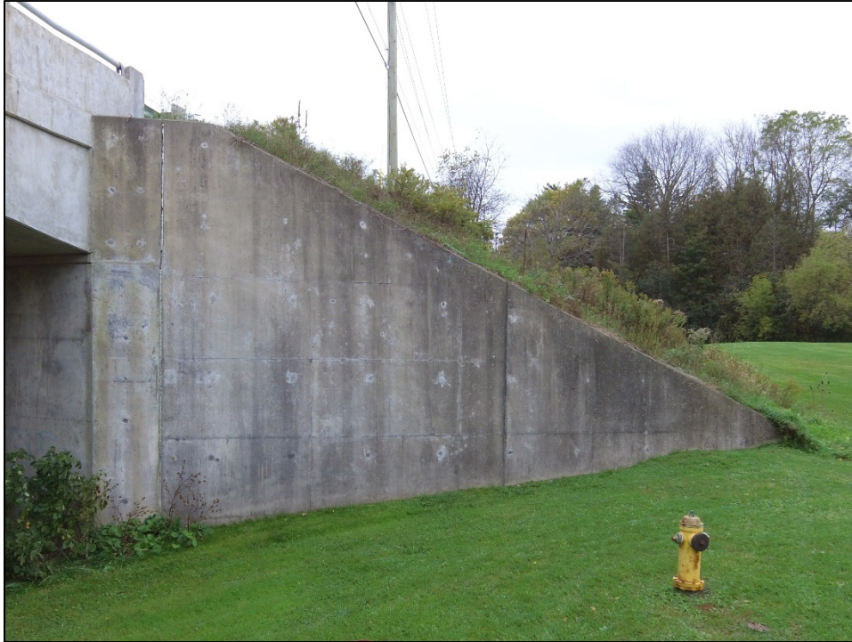
Photo P29 – Typical Condition of North-West Retaining Wall (fair condition)
