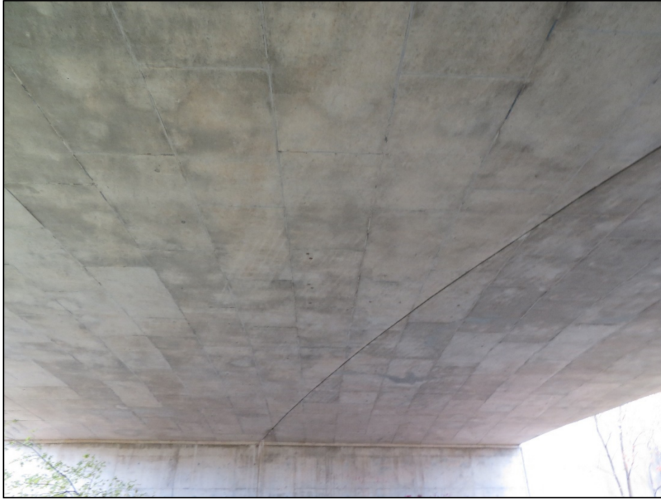
Photo P13 – Typical Condition of Soffit from West (fair-to-good condition – wet areas and efflorescence staining at construction joint)
