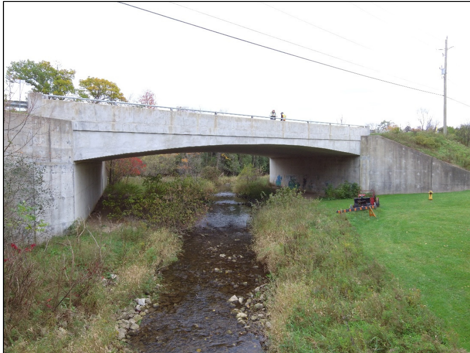
Photo P1 – North Elevation
