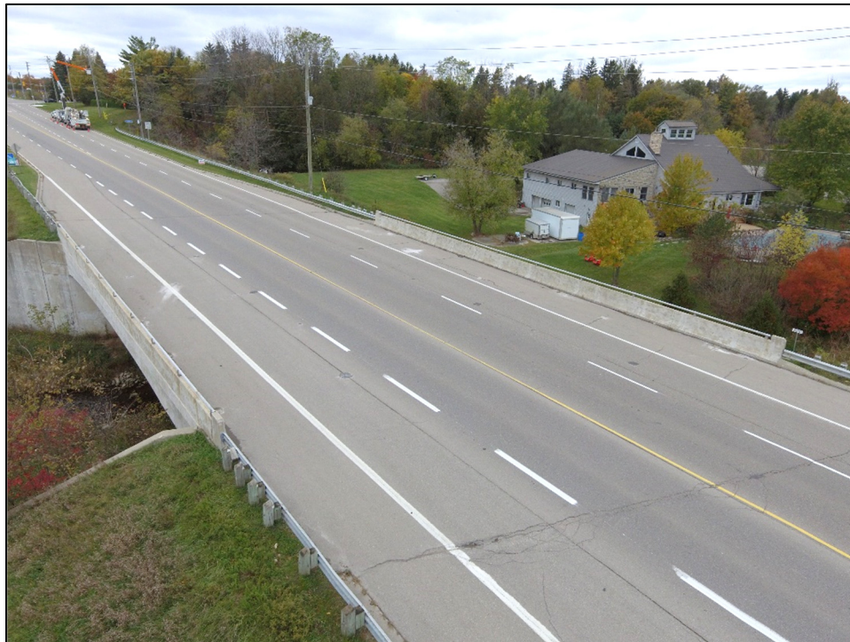
Photo P1: General View of Structure ID: 3801 Maple Grove Road / Chiligo / Fisher Mills Creek Bridge
