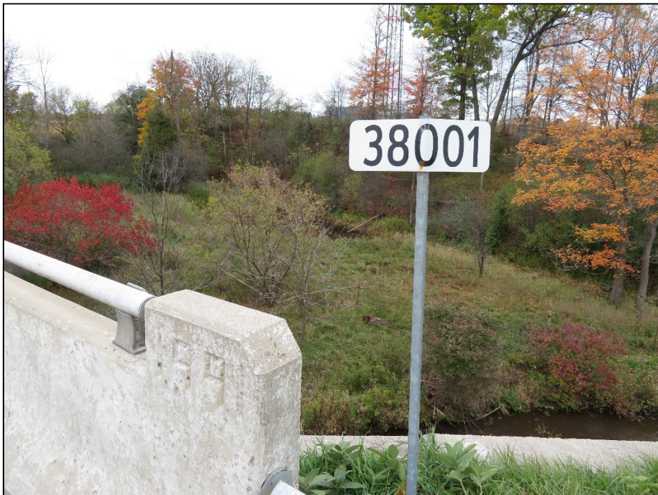
Photo P44 – Bridge Date Stamp on South Barrier Wall and Site Number Sign
