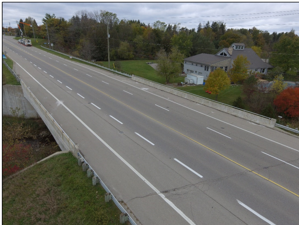
Photo P4 – Aerial Overview of Structure
