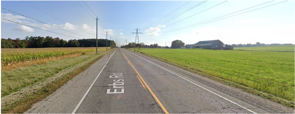
Figure 2.12: Erb's Road East of Nafziger Road (Source: Google Maps, 2025)
