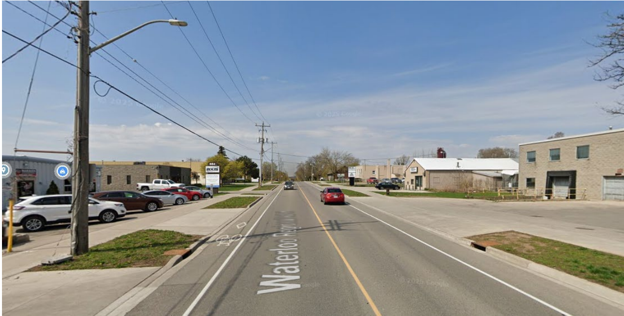
Figure 2.22: Bishop Street North in Cambridge (Source: Google Maps, 2025)
