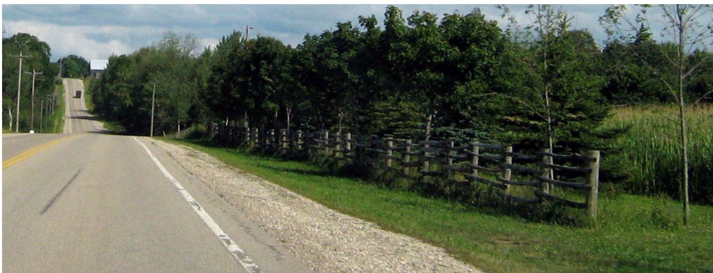
Shoulders provide a recovery area for errant vehicles, a refuge for stopping or disabled vehicles, and an area for emergency vehicles.
