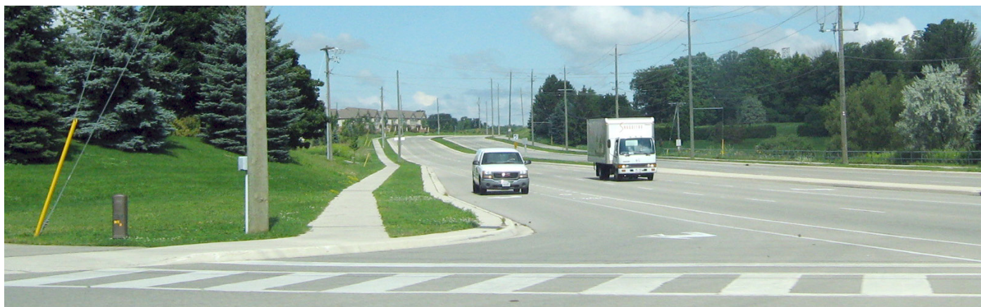
Right / left turn lanes are auxiliary lanes, which provide additional capacity at intersections and improve the level of roadway service.
