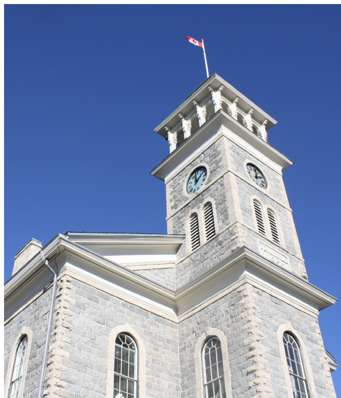
Historic downtowns, heritage buildings, and natural spaces provide an important quality of place and identity for their respective municipalities.
