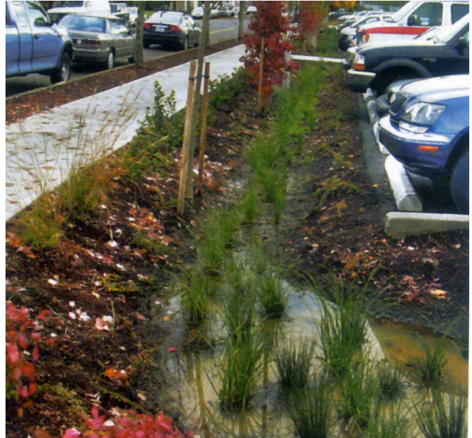
Bioswales capture, temporarily store, and treat stormwater runoff.
