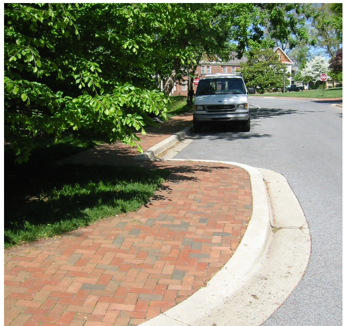
Curbs provide drainage control, right-of-way reduction, guidance, and access control.
