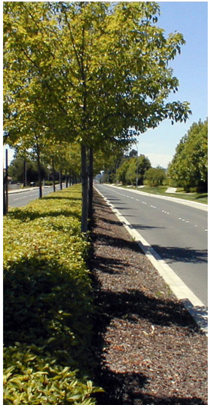
Medians can be used to control the location of vehicle turning movements along major roadways.
