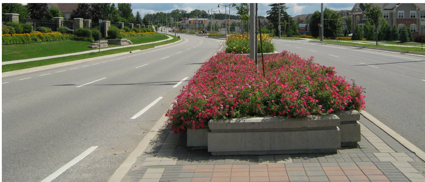
Medians can function as a safety barrier in order to reduce the risk of high speed head on collisions. They may also include vegetation.
