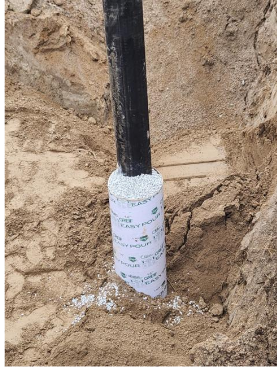
Photo 2: HD1 New Annular Seal
