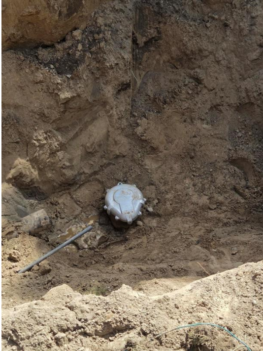
Photo 1: HD2 temporarily capped below grade
