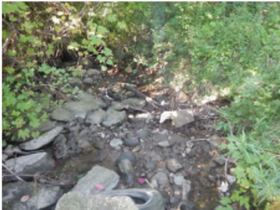
Photo #12: Looking at the channel condition of the downstream of C1.
