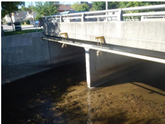
Photo #77: Looking at the downstream end of C10.
