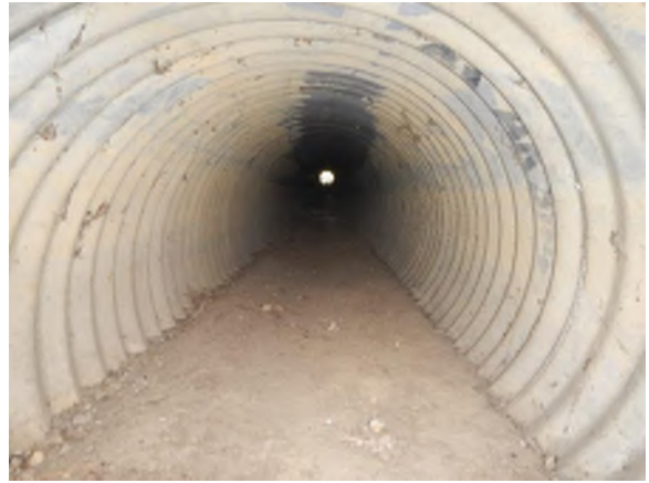
Photo #27: Looking inside the downstream end of C5.
