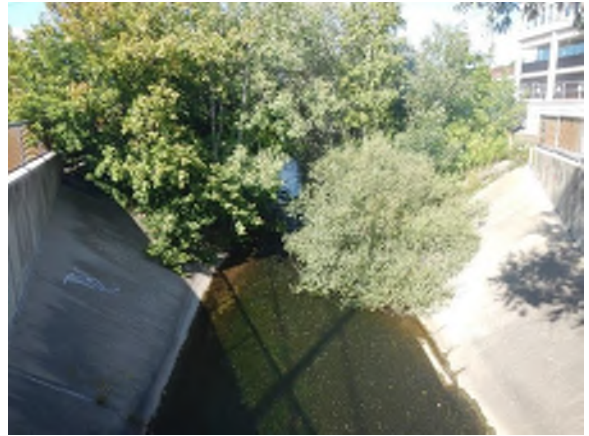
Photo #85: Looking at the channel upstream of C11.
