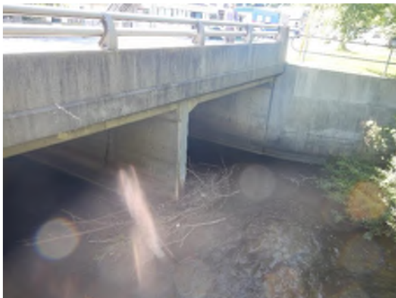
Photo #79: Looking at the upstream end of C10.
