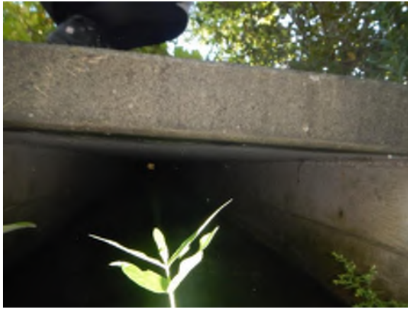
Photo #15: Looking at the downstream end of C3.
