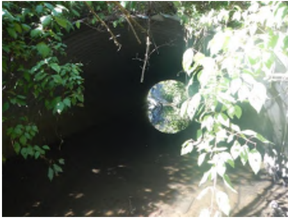
Photo #59: Looking at the upstream end of C7.
