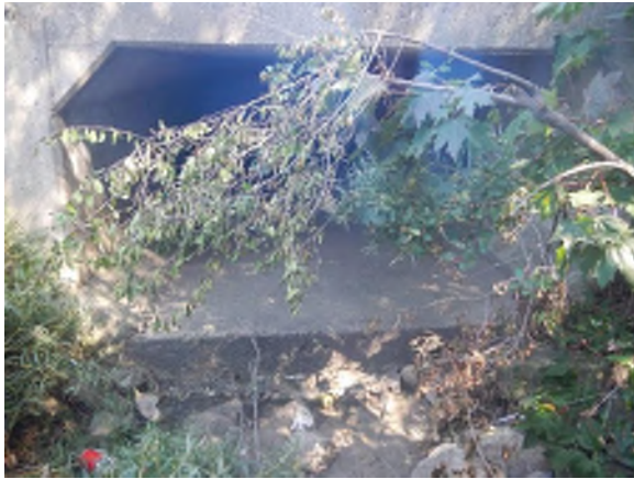
Photo #63: Looking at the upstream end of C8.
