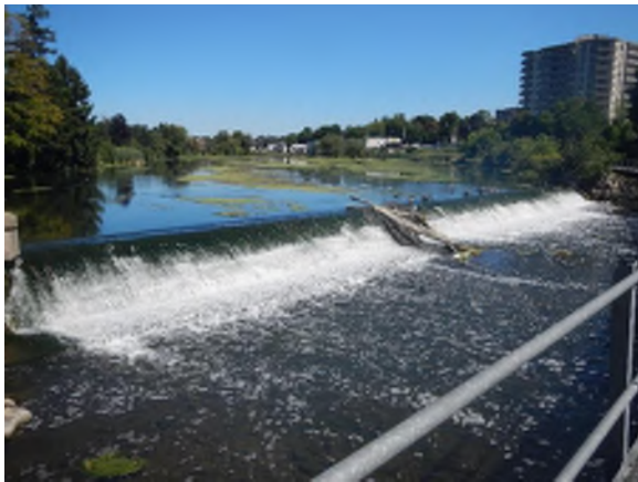
Photo #49: Looking northeast from the CN rail tracks at the Riverside Dam.
