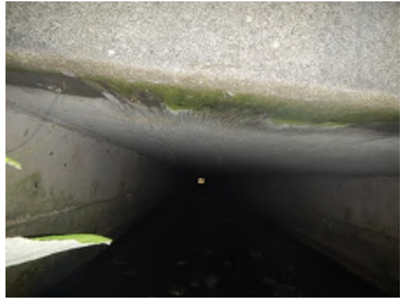
Photo #16: Looking inside the downstream end of C3.
