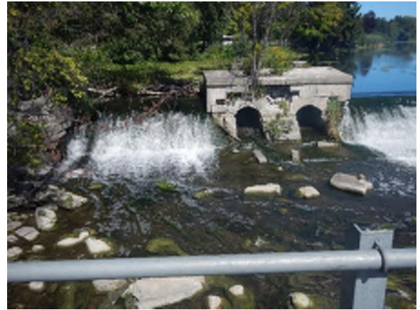
Photo #48: Looking northeast from the CN rail tracks at the Riverside Dam.
