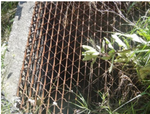
Photo #42: Looking at the ditch inlet on the south side of King St. and west of the 401 bridge.
