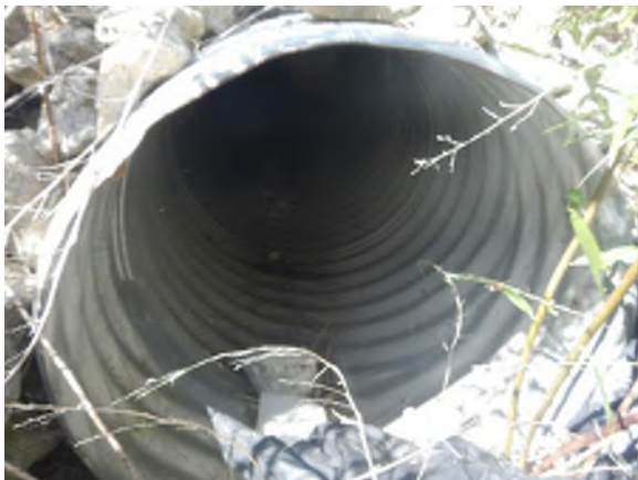
Photo #30: Looking at the upstream end of C5.
