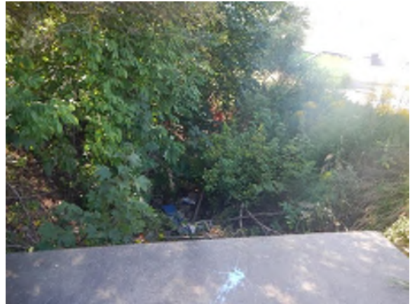
Photo #66: Looking at the channel upstream of C8.
