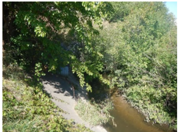
Photo #62: Looking at the channel and vegetation downstream of C7.
