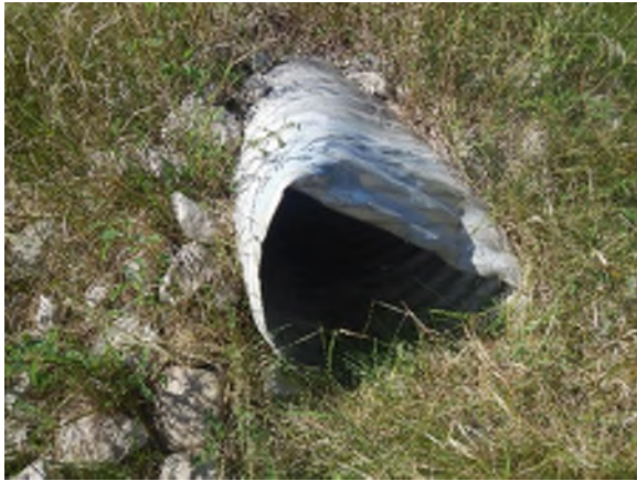
Photo #38: Looking at the upstream end of C6.
