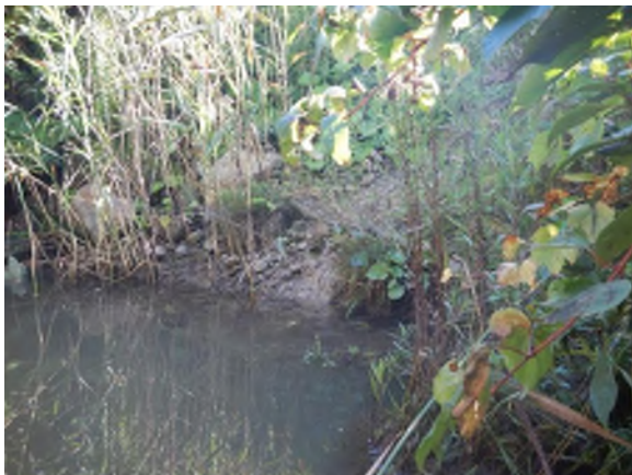
Photo #14: Looking at the slope to the right of C1.
