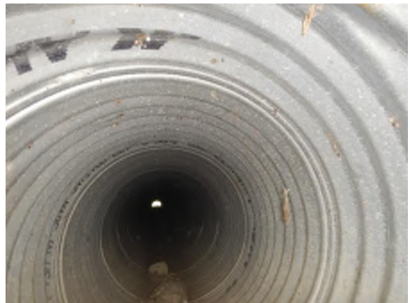
Photo #31: Looking inside the upstream end of C5.
