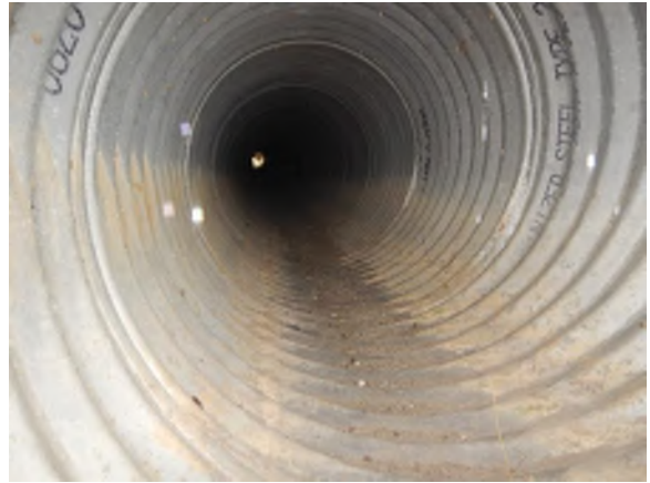
Photo #39: Looking inside the upstream end of C6.
