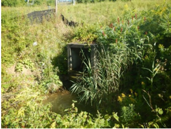
Photo #10: Looking at the downstream end of C2.
