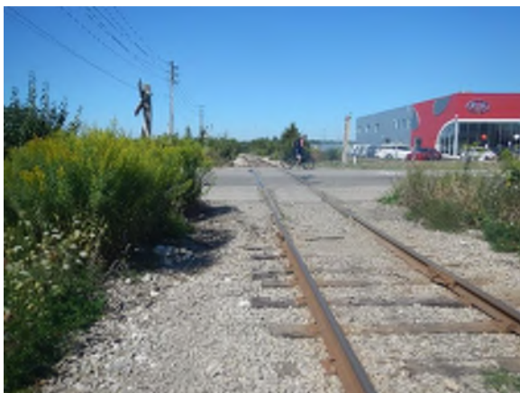
Photo #57: Standing on the rail tracks on the south side of Eagle St. looking north.
