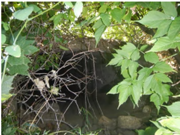
Photo #67: Looking at the downstream end of C8.
