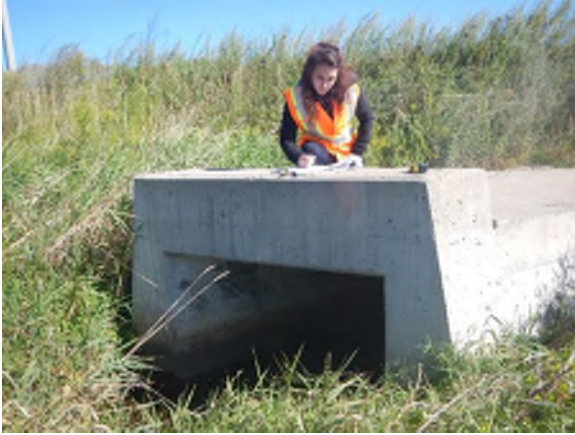
Photo #20: Looking at the downstream end of C4.
