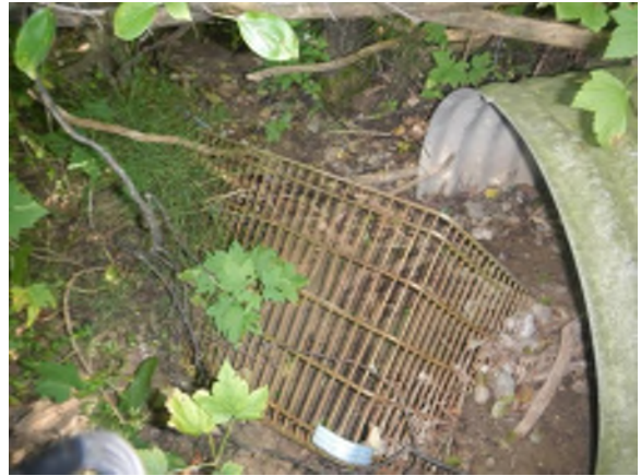
Photo #6: Looking inside the downstream end of culvert C1.
