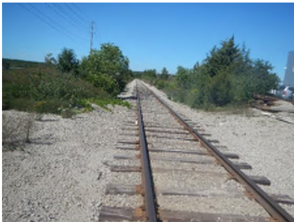
Photo #55: Standing on the rail tracks on the north side of Eagle St. looking north.
