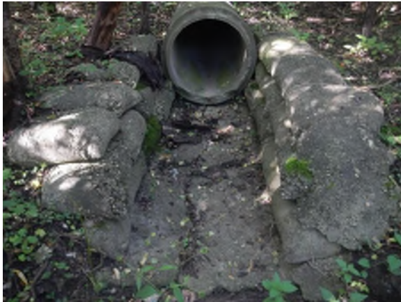
Photo #1: Looking at the downstream end of culvert discharging into C1. Located a short distance upstream of C1.
