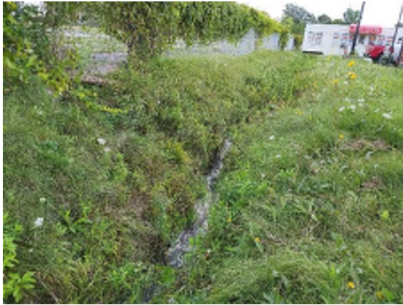
Photo #75: Looking at the channel upstream of C9.
