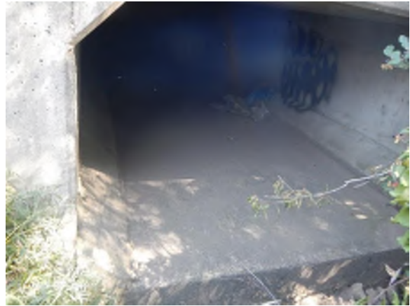
Photo #64: Looking at the upstream end of C8.
