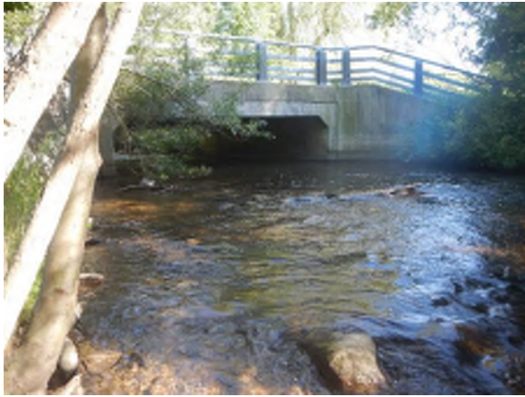
Photo #81: Looking at the downstream end of Soper Park Bridge.
