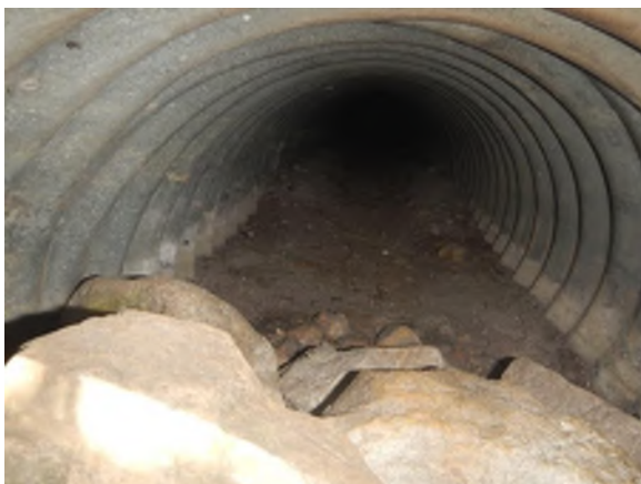
Photo #73: Looking inside the downstream end of C9.
