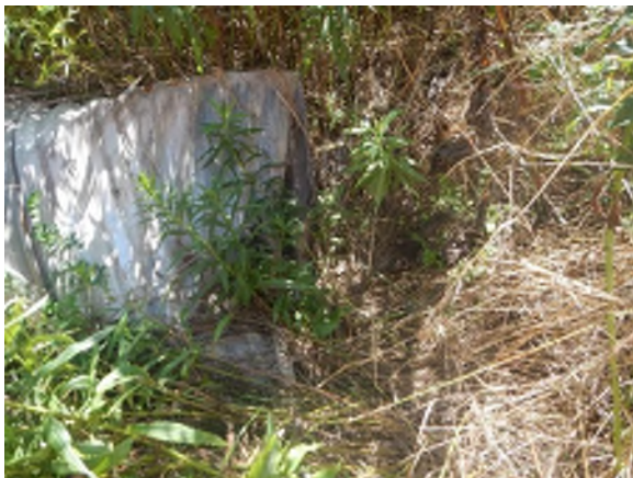
Photo #34: Looking at the downstream end of C6.
