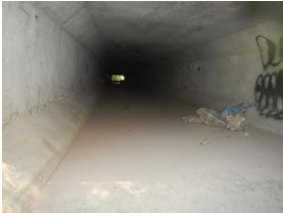
Photo #65: Looking inside the upstream end of C8.
