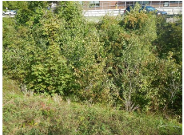
Photo #87: Looking at the vegetation in the upstream channel of C11.
