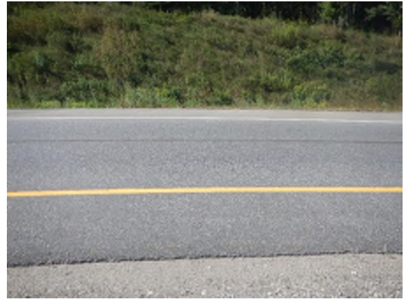
Photo #33: Looking at the condition of the road surface above C5.
