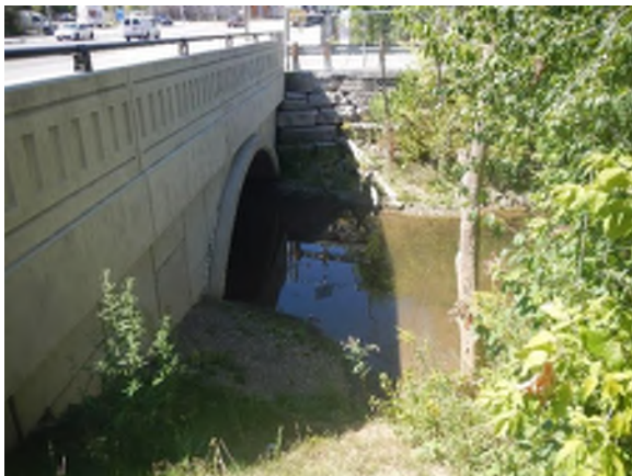
Photo #51: Looking at the upstream end of the King St. bridge at the Speed River.
