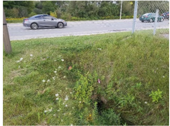
Photo #76: Looking at the road surface conditions above C9.
