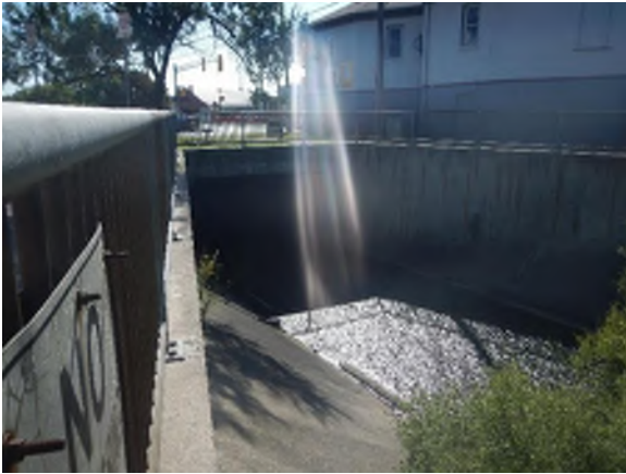
Photo #84: Looking at the upstream end of C11.
