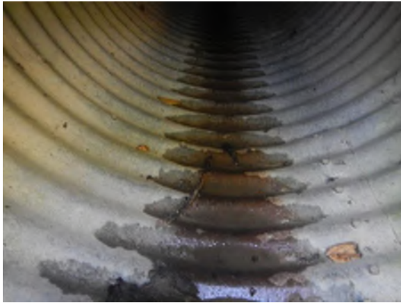
Photo #5: Looking inside the upstream end of culvert C1.
