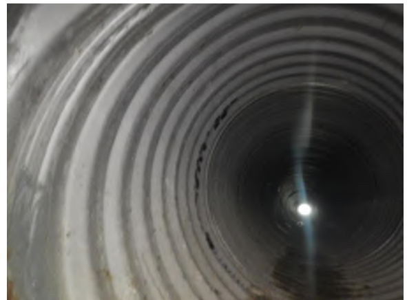
Photo #35: Looking inside the downstream end of C6.
