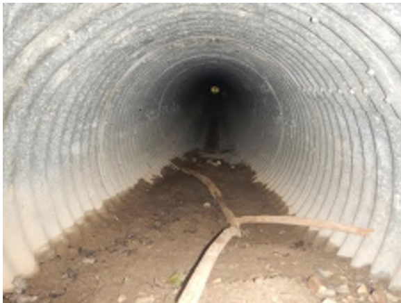
Photo #7: Looking inside the downstream end of culvert C1.
