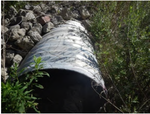
Photo #26: Looking at the downstream end of C5.
