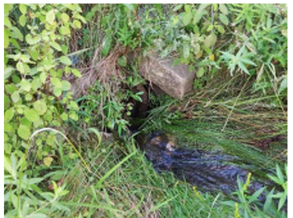
Photo #74: Looking at the upstream end of C9.
