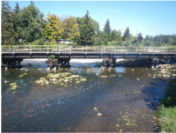
Photo #47: Looking northeast from the King St. East bridge at the CN rail tracks.
