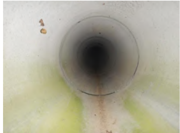
Photo #2: Looking inside the downstream end of the culvert discharging into C1. Located a short distance upstream of C1.
