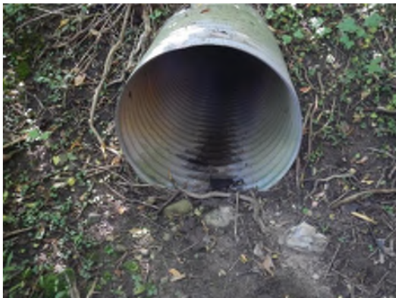
Photo #3: Looking at the upstream end of C1.
