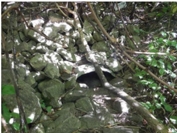
Photo #71: Looking at the downstream end of C9.
