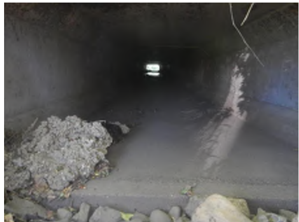
Photo #68: Looking inside the downstream end of C8.
