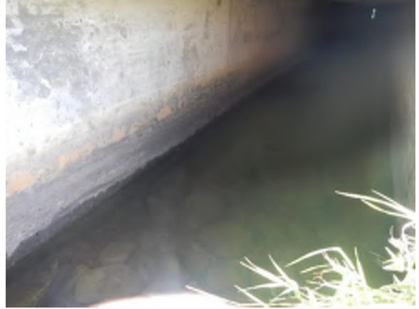
Photo #21: Looking inside the downstream end of C4.
