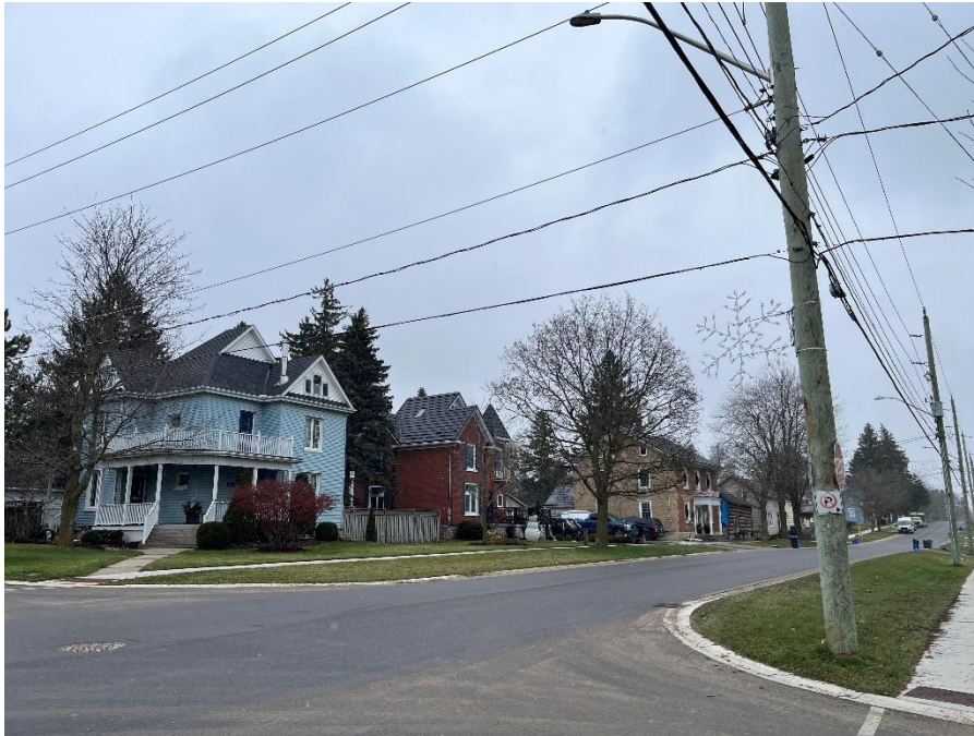
Plate 23: Homes on the northeast corner of Molesworth Street and Queen's Bush Road (A.S.I., 2024).
