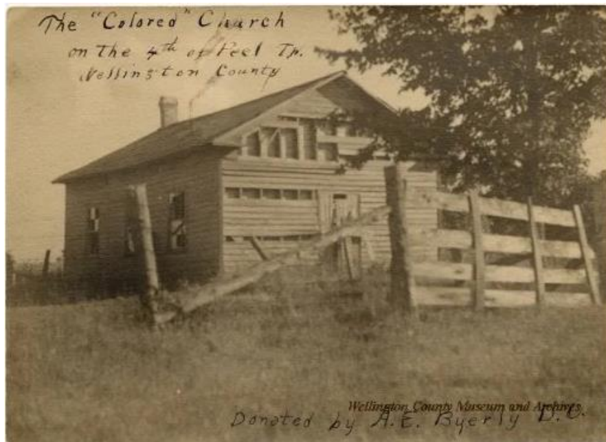
Figure 5: The African British Methodist Episcopal Church building in Peel Township (image source: Wellington County Museum and Archives)
