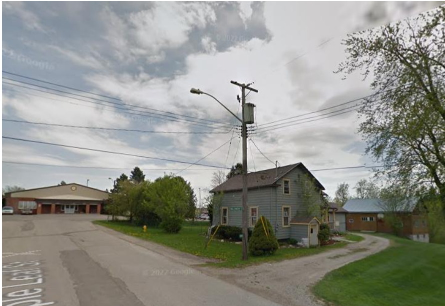
Plate 6: Example of a house within the central proposed elevated tank study area, west of the Wellesley Community Centre (Google Streetview). 5
