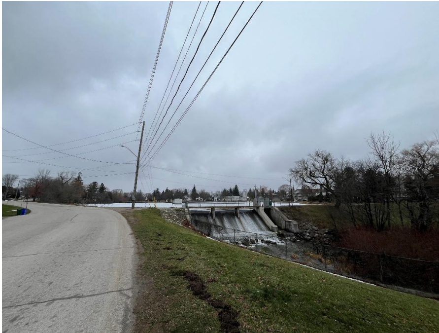
Plate 19: View of the dam at Wellesley Pond off David Street, facing north (A.S.I., 2024).
