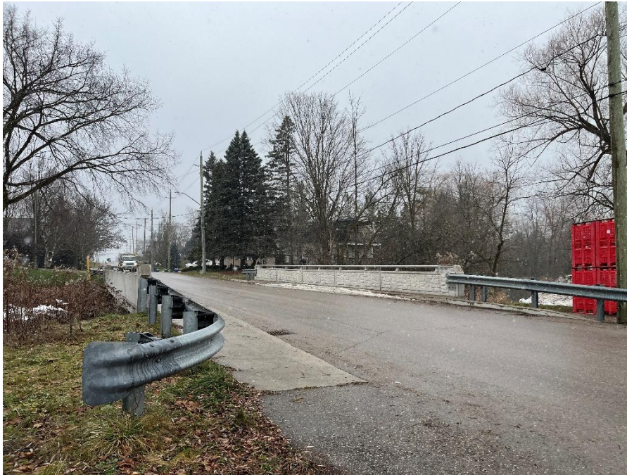
Plate 9: Northern approach to the Nafziger Road bridge over a creek from Mill Pond (A.S.I., 2024).
