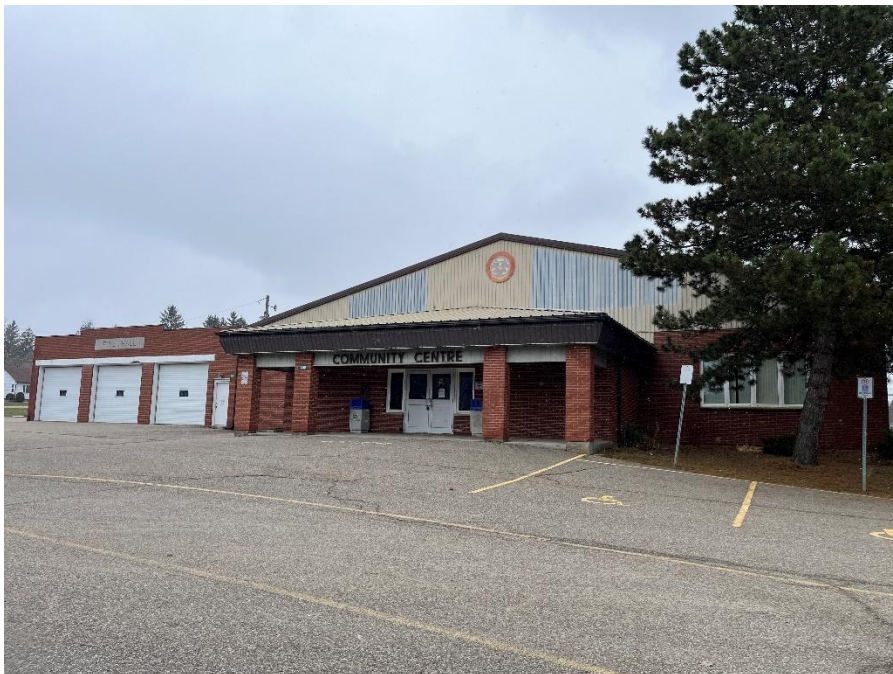
Plate 4: Wellesley Community Centre west elevation (A.S.I., 2024).
