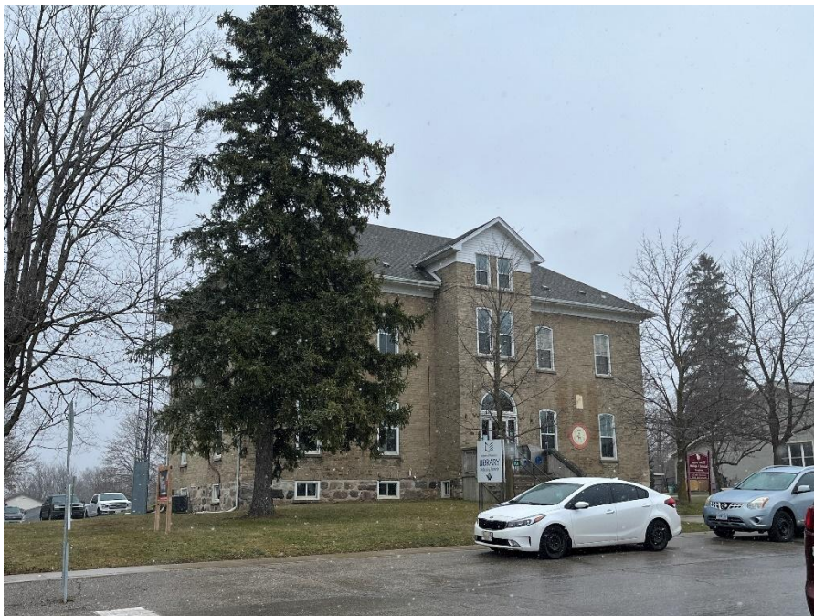
Plate 12: 1137 Henry Street, a Part IV designated property, looking north at the south elevation (A.S.I., 2024).
