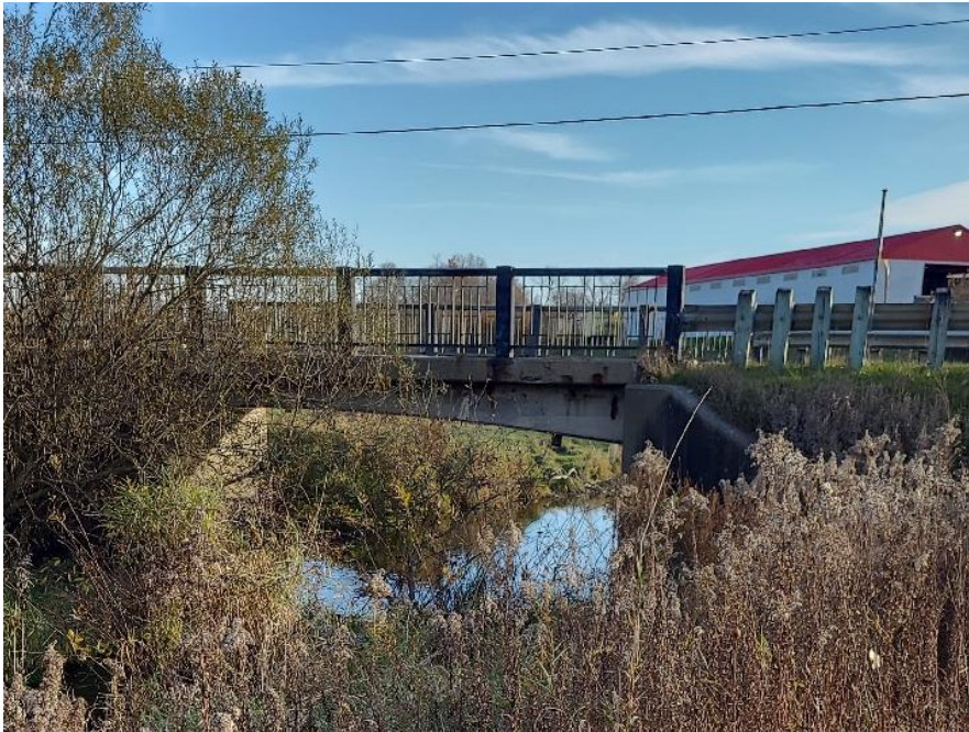
Plate 33: Gerber Road carried over a bridge at Firella Creek, looking south (A.S.I., 2024).
