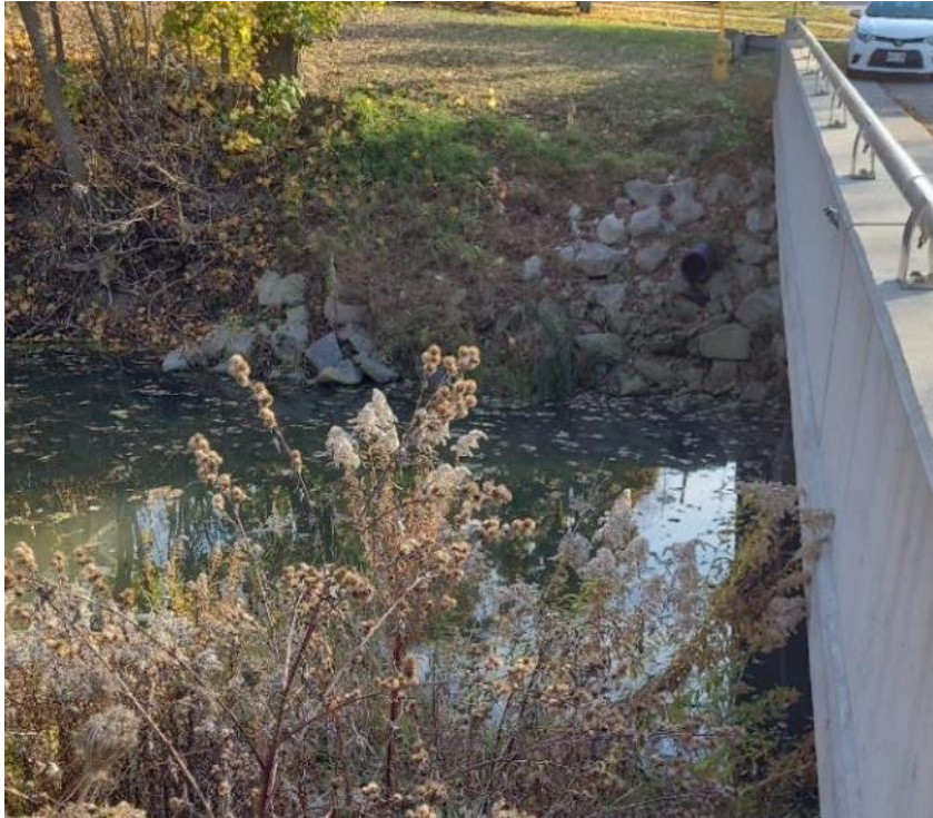
Image 17: Sanitary pipe west of Nafziger Road; disturbed, no archaeological potential.
