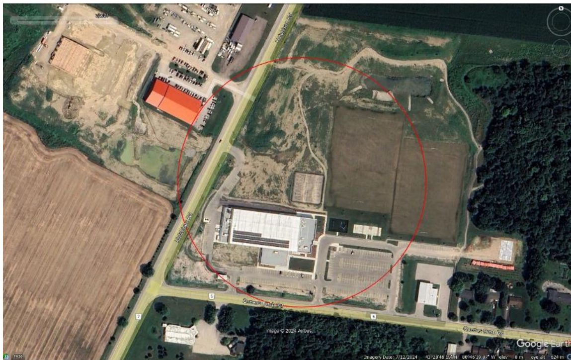
Image 41: 2024 Google satellite image showing active grading and construction west of Hutchinson Road within Elevated Tank Alternative 1.
