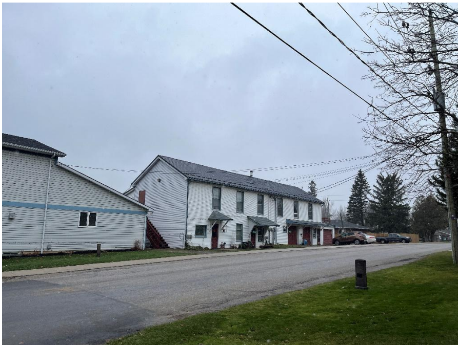
Plate 24: Multi-family residence at the northwest corner of Molesworth Street and Queen's Bush Road (A.S.I., 2024).
