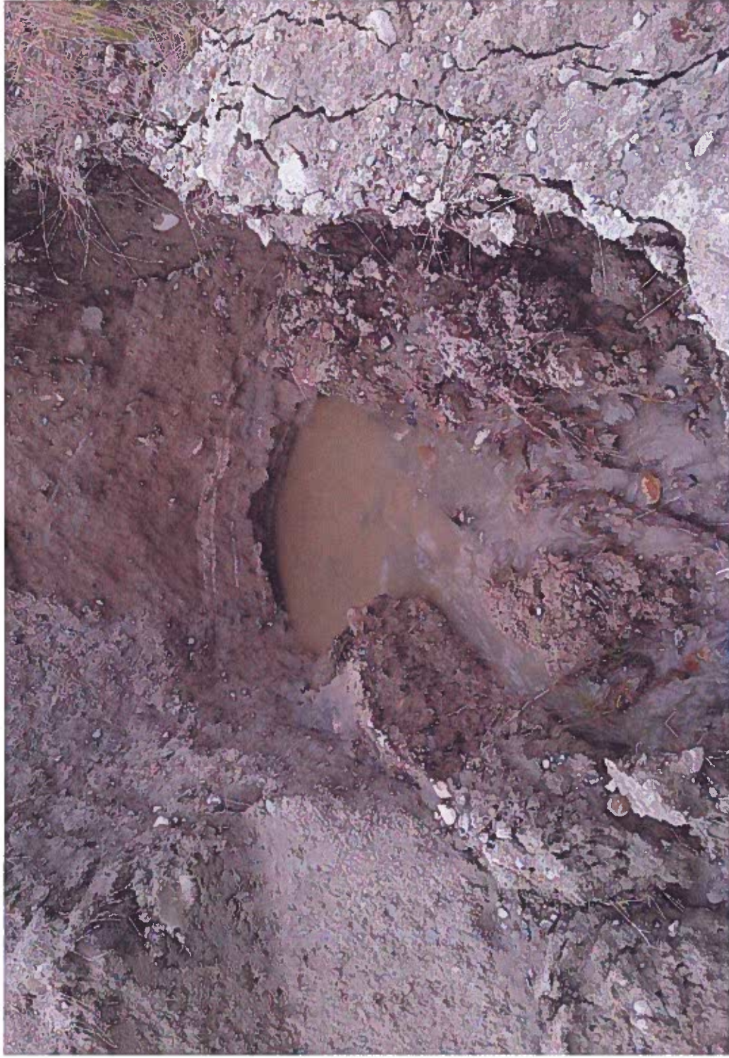
Photo 2. Spring on Lot 2 prior to backfilling with crushed gravel.
