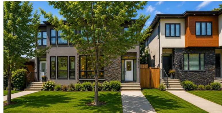
Figure 5 - Example of a pedestrian walkway connecting the sidewalk to the entrance
