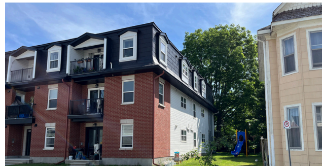
Figure 17 - Local example of a low-rise infill apartment that incorporates traditional architectural features, including a mansard roof and red brick, reflecting elements commonly found in Smiths Falls' built heritage.
