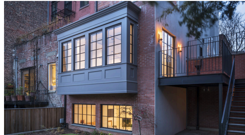
Figure 18 - Example of a projecting bay window integrated into an existing building façade
