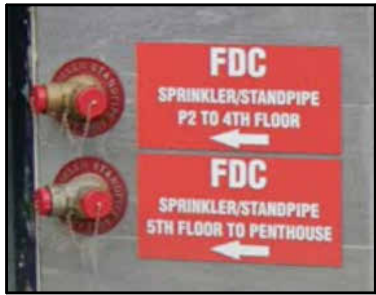
EXAMPLE REFERENCE STACKED FIRE DEPARTMENT CONNECTIONS
